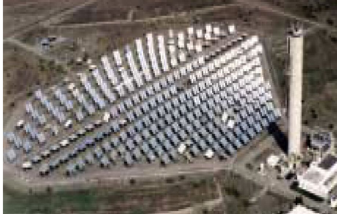
Figure 1.2. Solar Tower Test Site CESA - 1 at Plataforma Solar, PSA, Almería , Spain.
