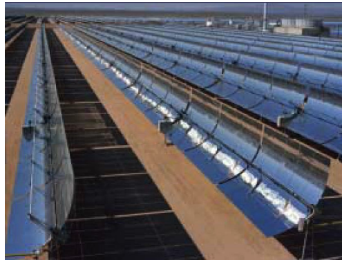
Figure 1.1. Trough Collector Field in Kramer Junction, California.
