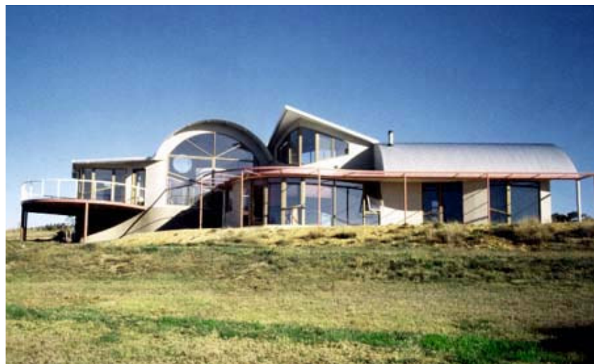
Figure 2.2. An example house built on direct gain principles in Wooden, Australia (Source: WEB_10, 2005)
