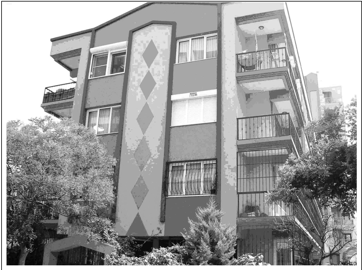
Figure 6.2. Front view of Doğan Apartment Building
