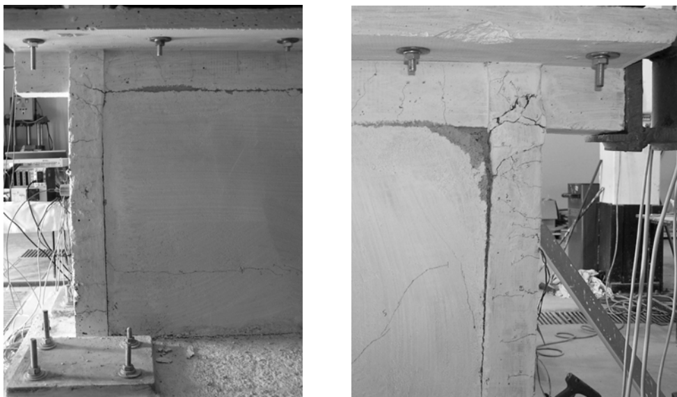
Figure 3.29. Damage in first story west column (left) and east column (right) at the end of the fifth loading group, south face
