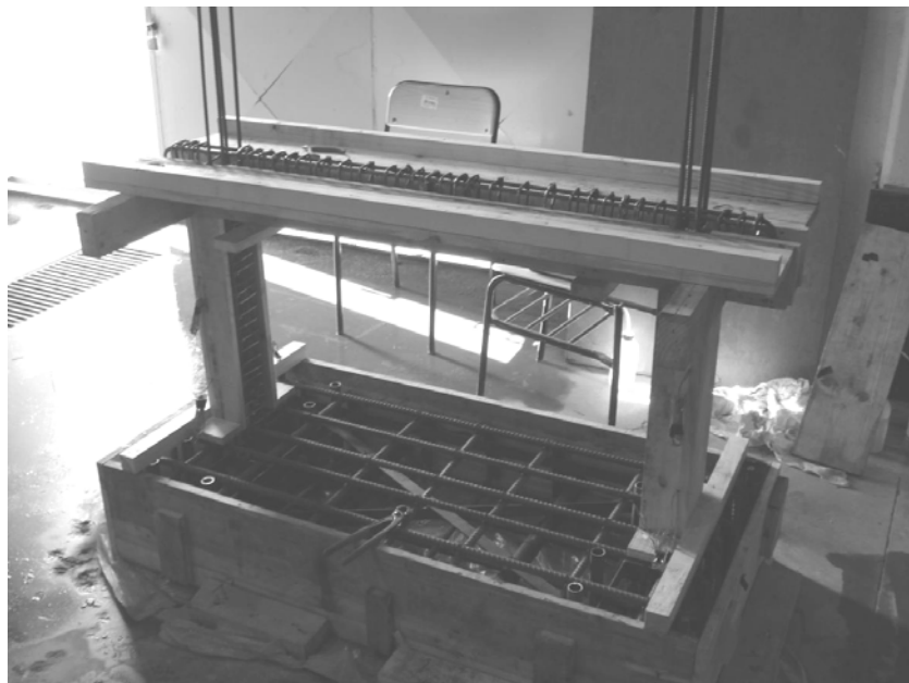
Figure 2.4. First floor cage and the formwork
