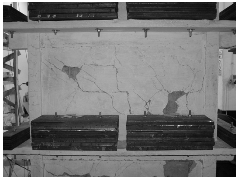
Figure 3.24. Residual deformation of the second story columns and the partition wall
