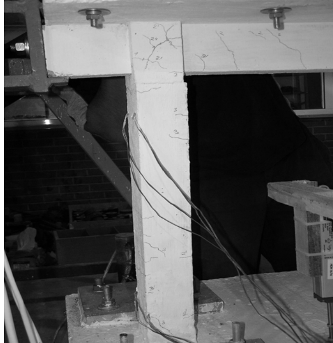
Figure 3.11. Cracks at the north face of the first story east column, at the end of the third loading group
