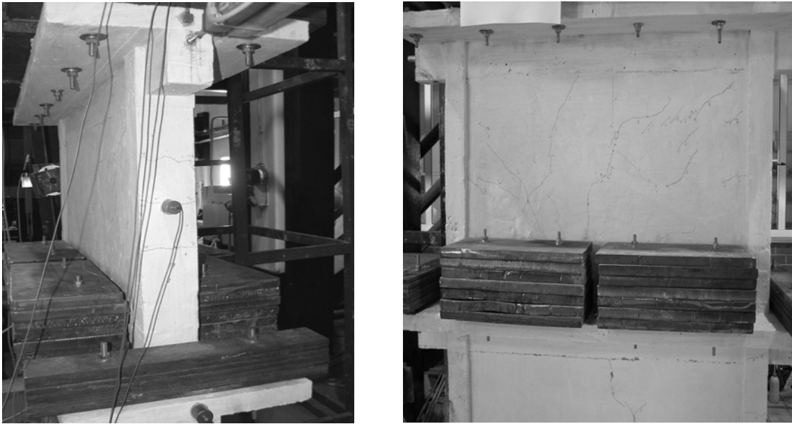
Figure 3.20. Spreading of flexural cracks in the west column (left) and shear cracks in the partition wall (right) of the second story, at the end of second loading group
