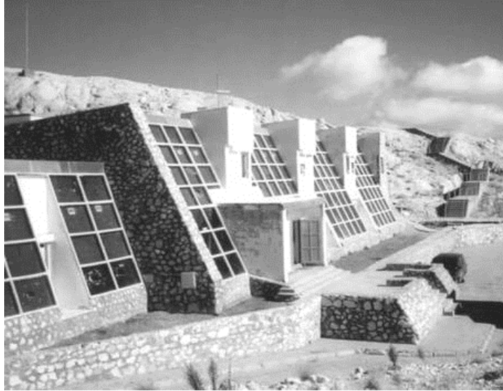
Figure 4.2: General view of TÜBİTAK National observatory. Greenhouses and trombe walls are seen on the south side of the rooms (Demirbilek et al., 2003).
