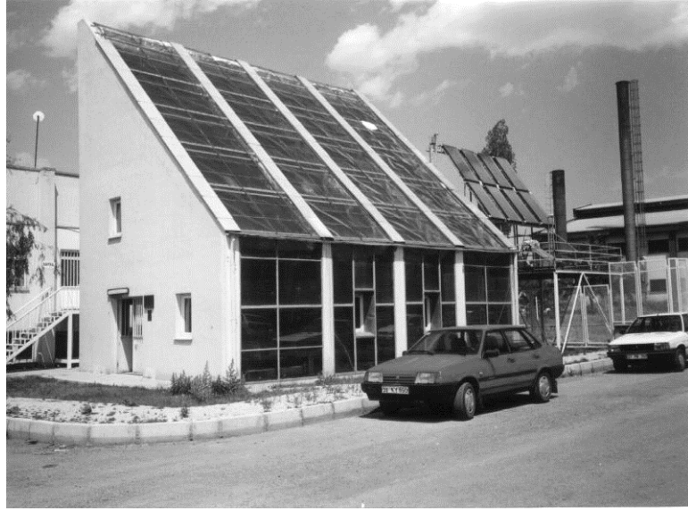
Figure 3.1: Solar house of Erciyes University, Kayseri, Türkiye. South facade of the building and the roof has active solar components. Trombe wall on facade, and air collector on the roof.
