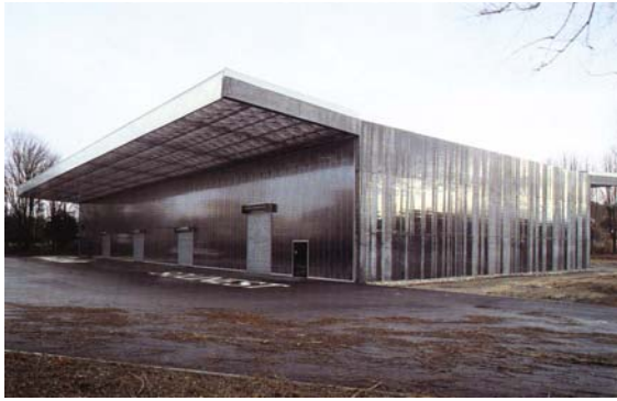
Fig 4.16 Ricola Factory, Mulhouse, General View
