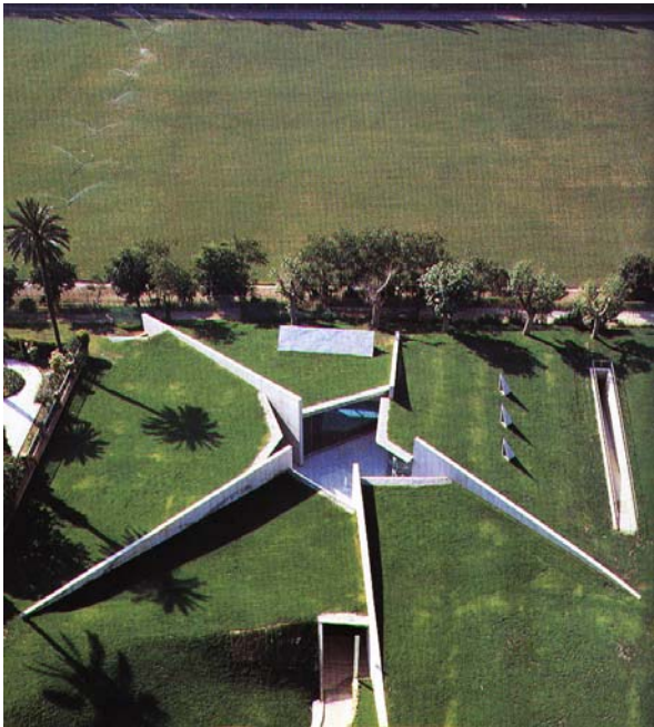
Fig 4.61 Fitness Center, Barcelona, 1993, Aerial View
