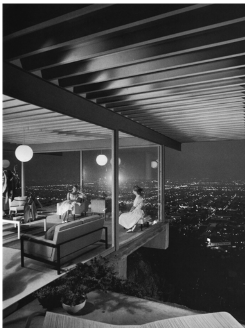
Fig 3.19 Stahl House, California, 1959-60, Pierre Koenig
