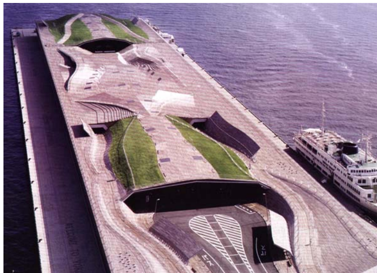
Fig 4.30 International Port Terminal, Yokohama, General View
