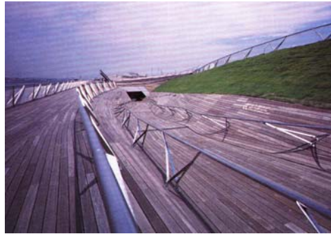
Fig 4.35 International Port Terminal, Yokohama, Detail from the Roof
