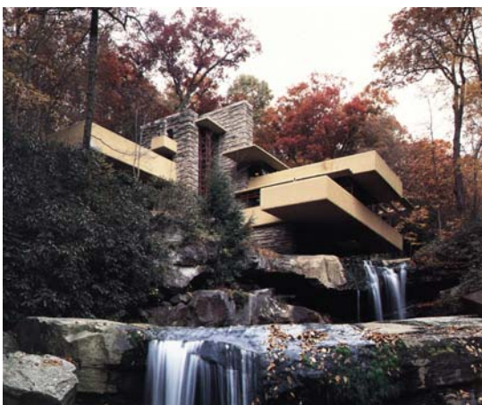
Fig 3.45 Fallingwater, View from below
