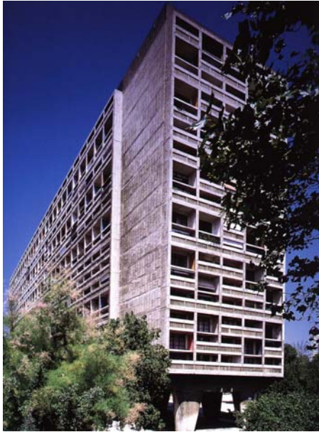
Fig 3.43 Unite D'Habitation, General View
