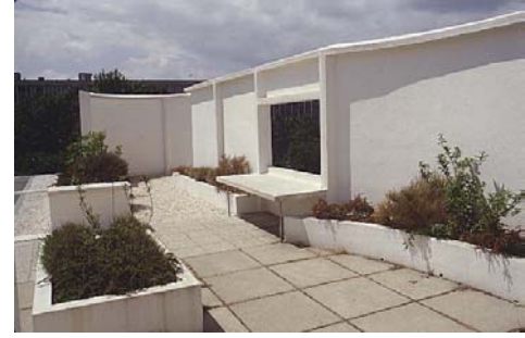
Fig 4.2 Villa Savoye, Roof Garden
