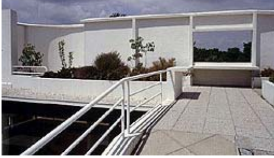
Fig 4.1 Villa Savoye, Roof Garden
