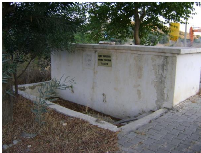
Figure 4.21. Kandıralı Fountain front façade
