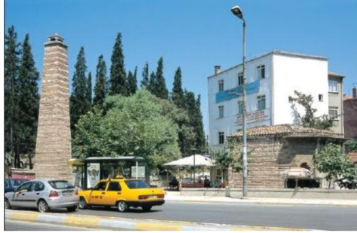
Figure 3.6. İstanbul Üsküdar Selimiye Water Tower (Source: Üsküdar Bld 2009)
