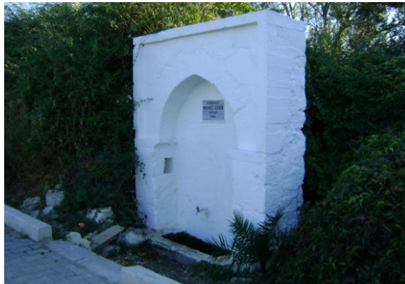
Figure 4.34. Tenekeci Fountain front and right façades
