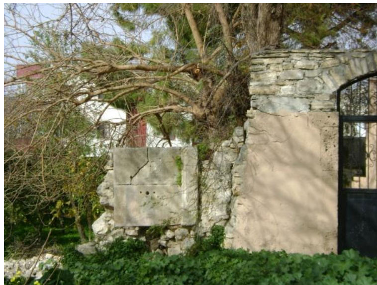
Figure 4.121. Reşid Ağa Fountain front façade
