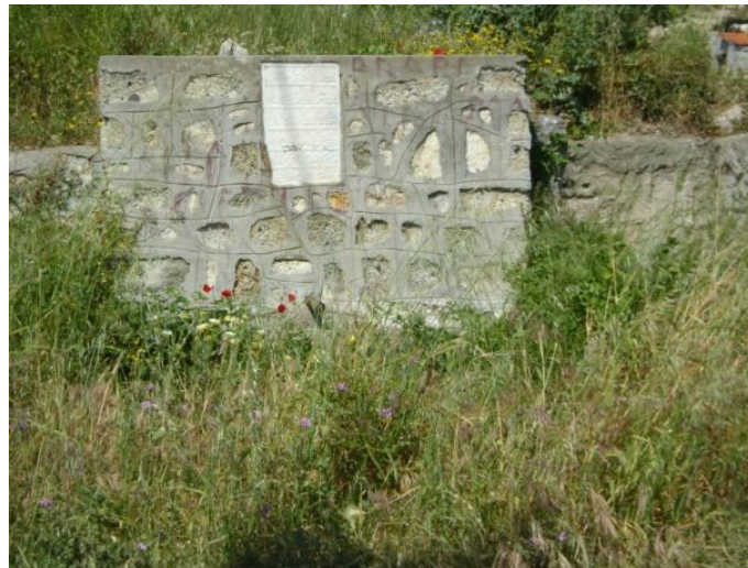
Figure 4.32. Şerif Ağa Fountain front façade
