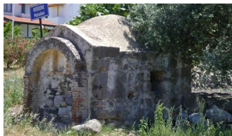
Figure 4.60. Reisdere Fountain front and right side façades
