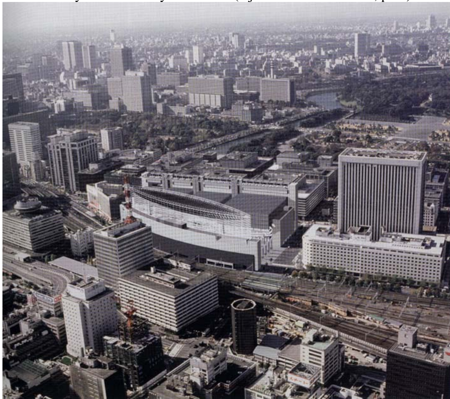
Figure 1.1 Hyper-realistic digital rendering - Tokyo International Forum by Rafael Vinoly Architects (Ojeda and Guerra 1996, p.37)
