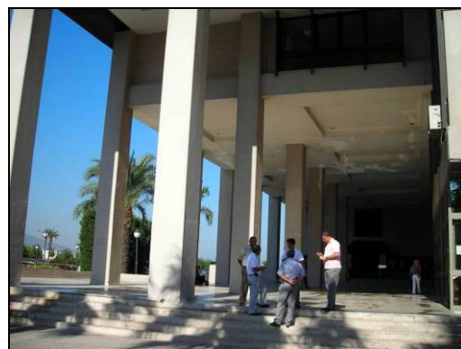
Figure 4.6. A view from the ground floor of the building
