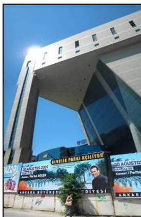
Figure 4.34. A view from the ground floor of the building
