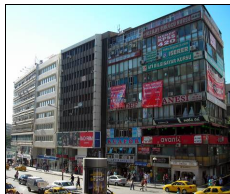
Figure 4.42. A view from low use of air conditioning
