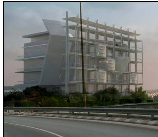
Figure 3.14. Tel Aviv University Building (Source: WEB_15 2009)
