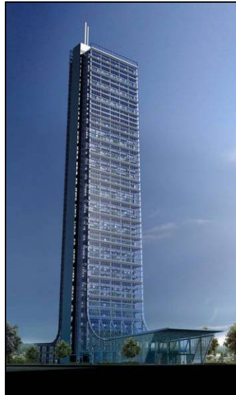
Figure 3.23. Istanbul Sapphire Green Tower (Source: WEB_24 2009)
