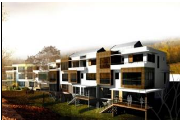
Figure 3.17. Çiğli Housing Development (Source: WEB_20 2009)
