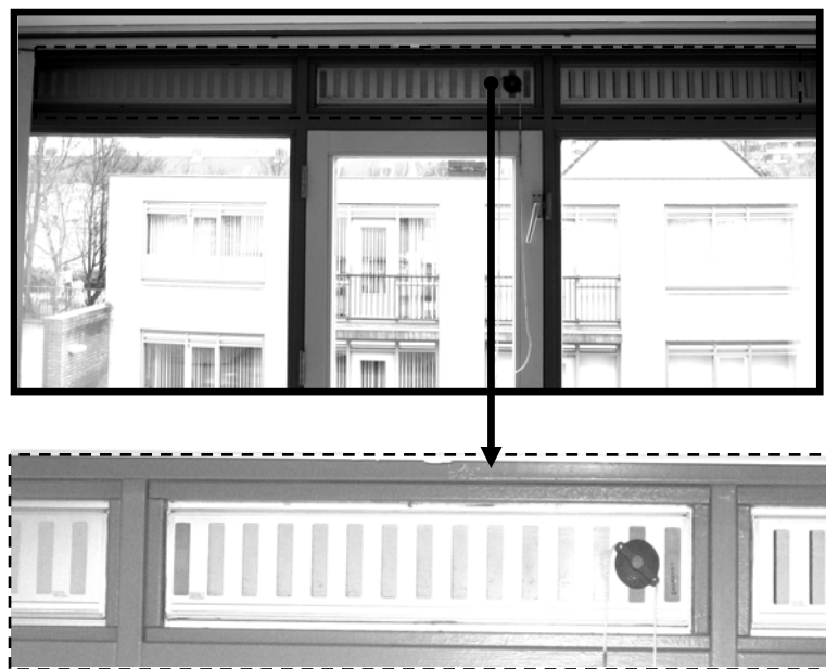
Figure 2.1. Window to provide controlled fresh air
