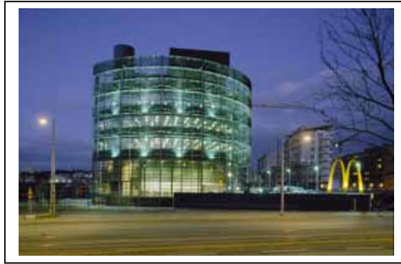
Figure 3.16 Mc Donald's office building, Helsinki-Finland 1995-97
