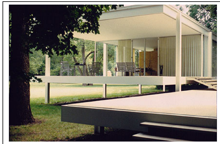
Figure 2.17 Farnsworth House, 14520 River Road, Plano, Illinois
