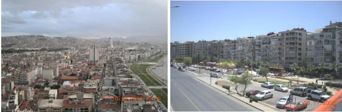
Figure 3.1. The urban sprawl in the year 2010. View from the Punta district towards Alsancak and Konak (Left), Figure 2.20. Continuous multistoried buildings along the coastal line in Güzelyalı, Izmir (2008) (Right).
