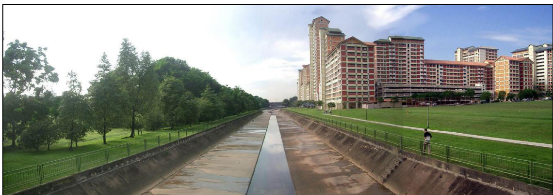
Figure 3.6. Kallang River before the rehabilitation project (Source: Ramboll Group, 2012)
