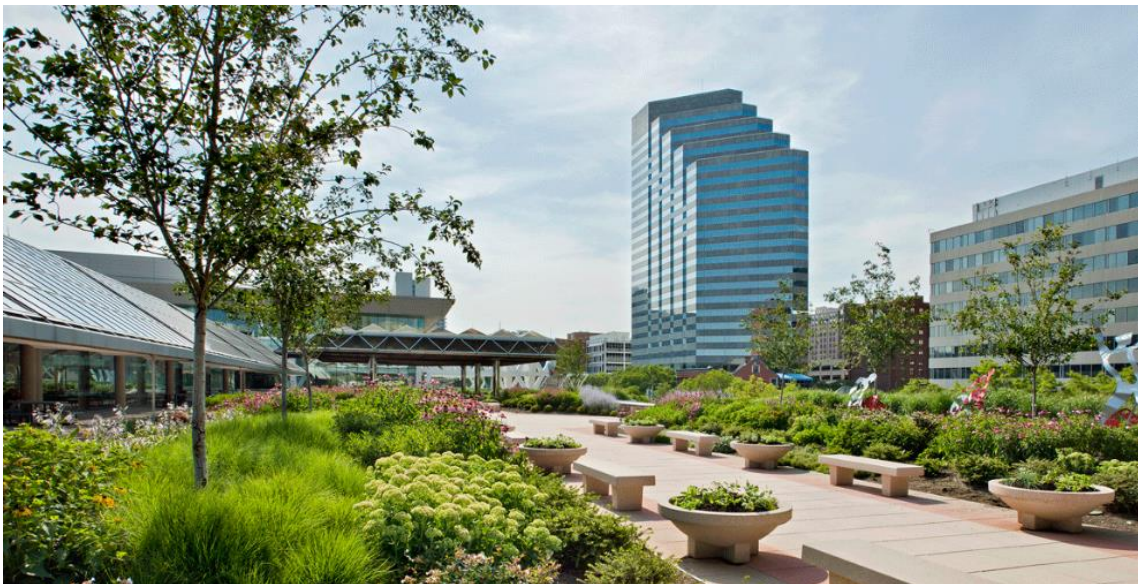
Figure 2.11. An intensive green roof from Baltimore, USA (Source: http://www.greenroofs.com/projects/pview.php?id=1337 )
