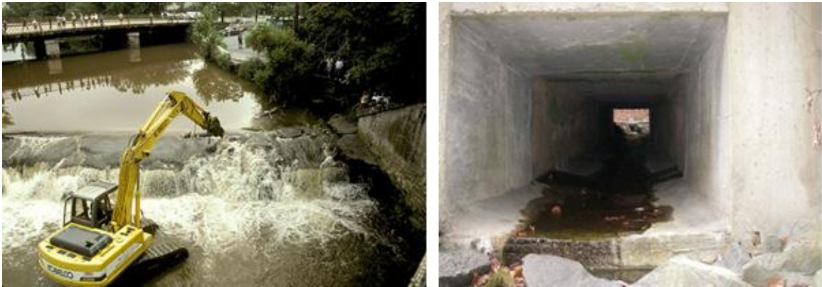
Figure 2.24. Removal of dam and road culverts (Source: Aadland, 2010)
