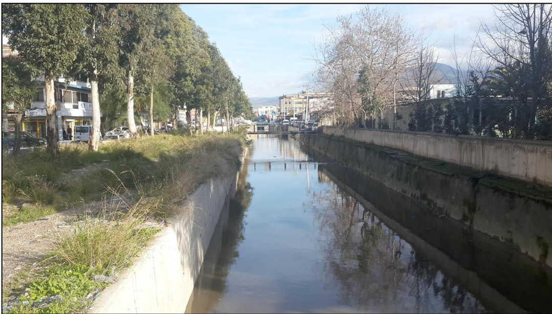
Figure 4.32. The banks of Arap Stream (December 2015)
