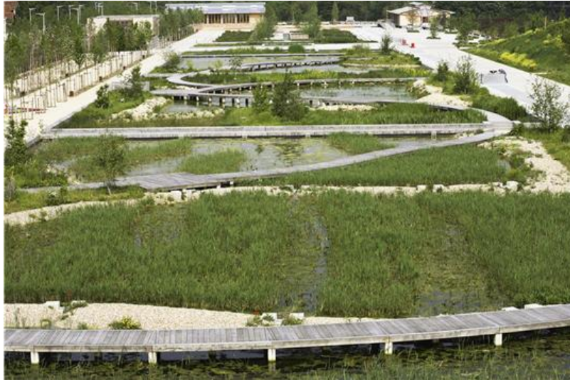
Figure 2.18. Phytoremediation technique depicting use of aquatic plants to clean water (Source: http://www.linternaute.com/savoir/grands-chantiers/06/dossier/seine-arche-nanterre/images/11.jpg )
