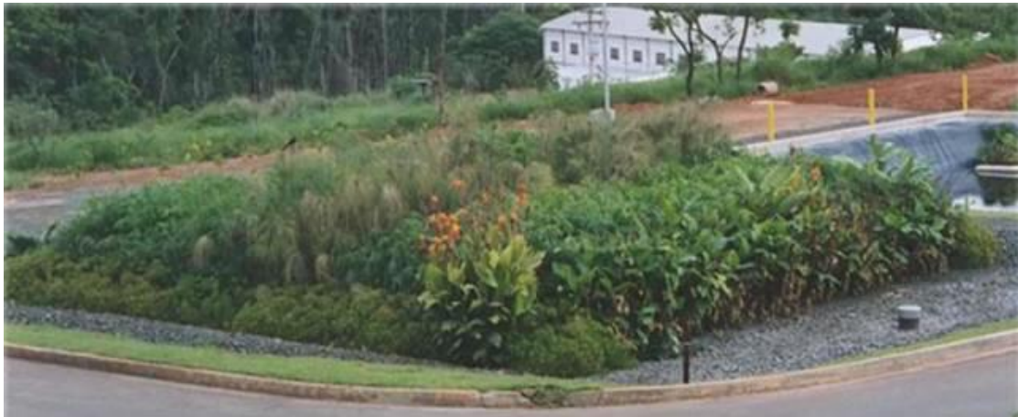
Figure 2.19. First constructed wetland in Turkey (Source: Yurtseven & Çakmak, 2007)
