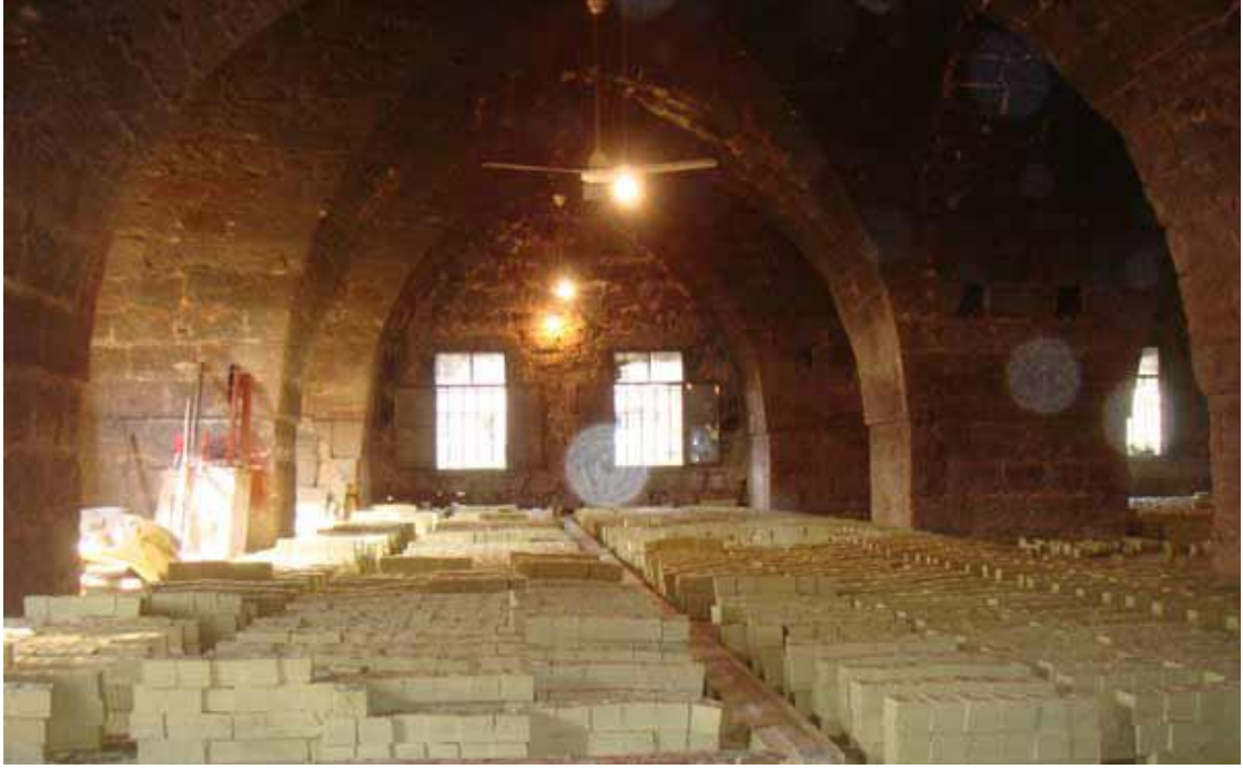
Figure 5.46. The cross vaults on the spreading and drying area in Sadık Adra Soap Factory, Tripoli
