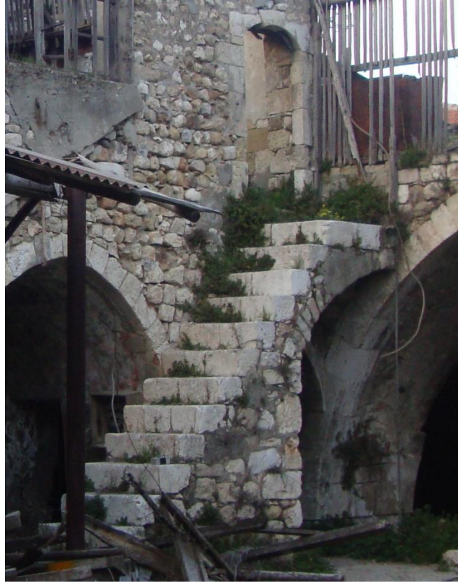
Figure 5.105. View of the straight stone stair on the courtyard facade in Aselci Soap Factory, Antakya
