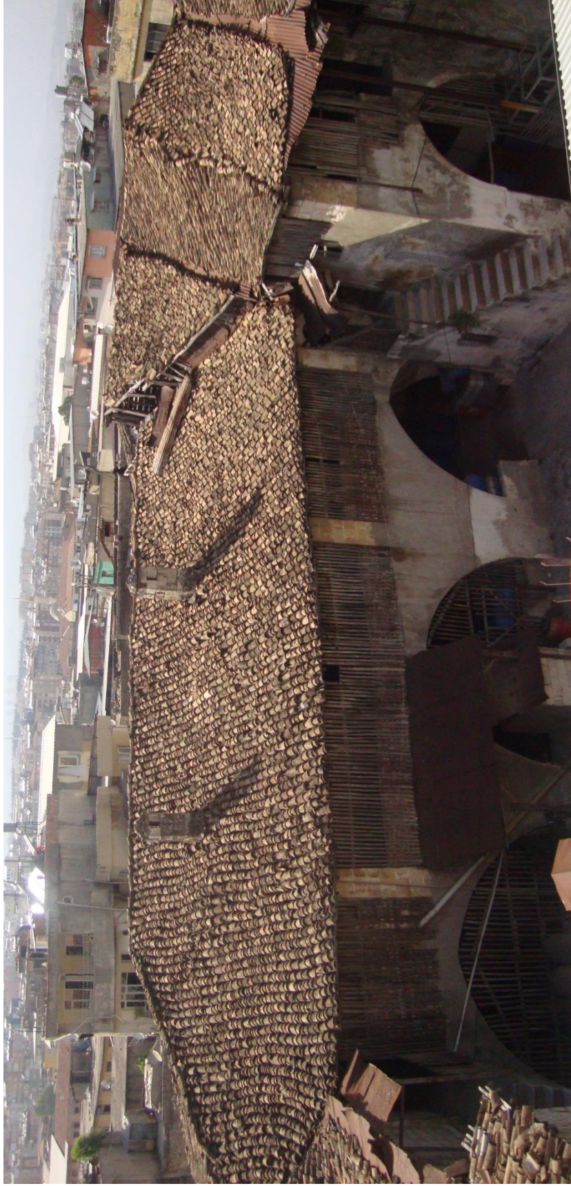
Figure 4.79. The original and renewed part of the hipped roof
