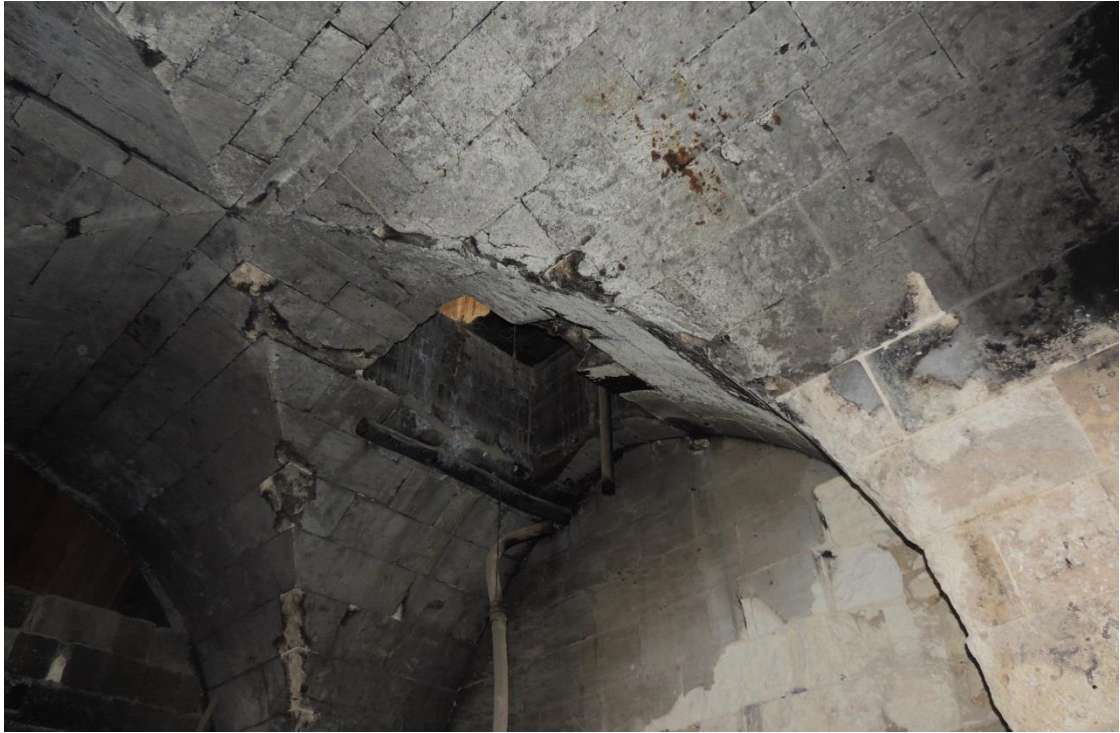
Figure 5.123. The rectangular hole on the vault of the closed gallery in Sayınlar Soap Factory, Nizip
