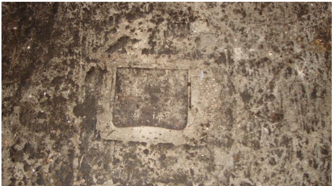
Figure 4.144. The trace of the cut stone masonry chimney on the floor of the semi-open gallery on the ground floor
