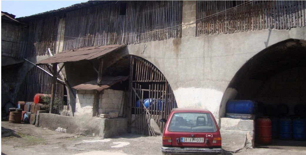
Figure 4.103. The depressed pointed arches on the courtyard facade
