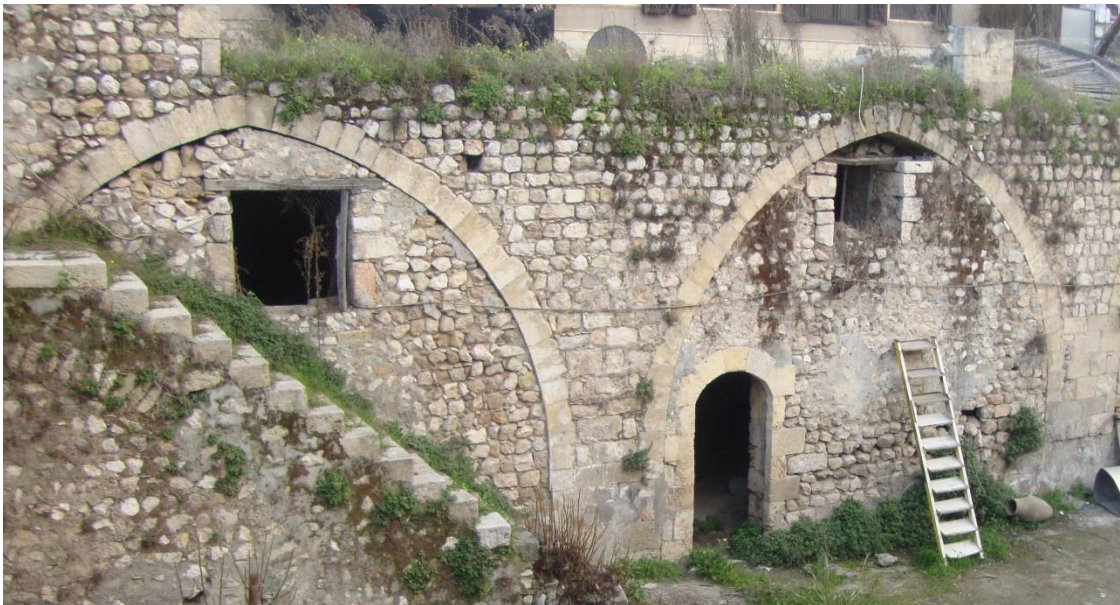
Figure 5.22. The closed gallery isolated from the courtyard by stone masonry walls between depressed pointed arches in Aselci Soap Factory, Antakya
