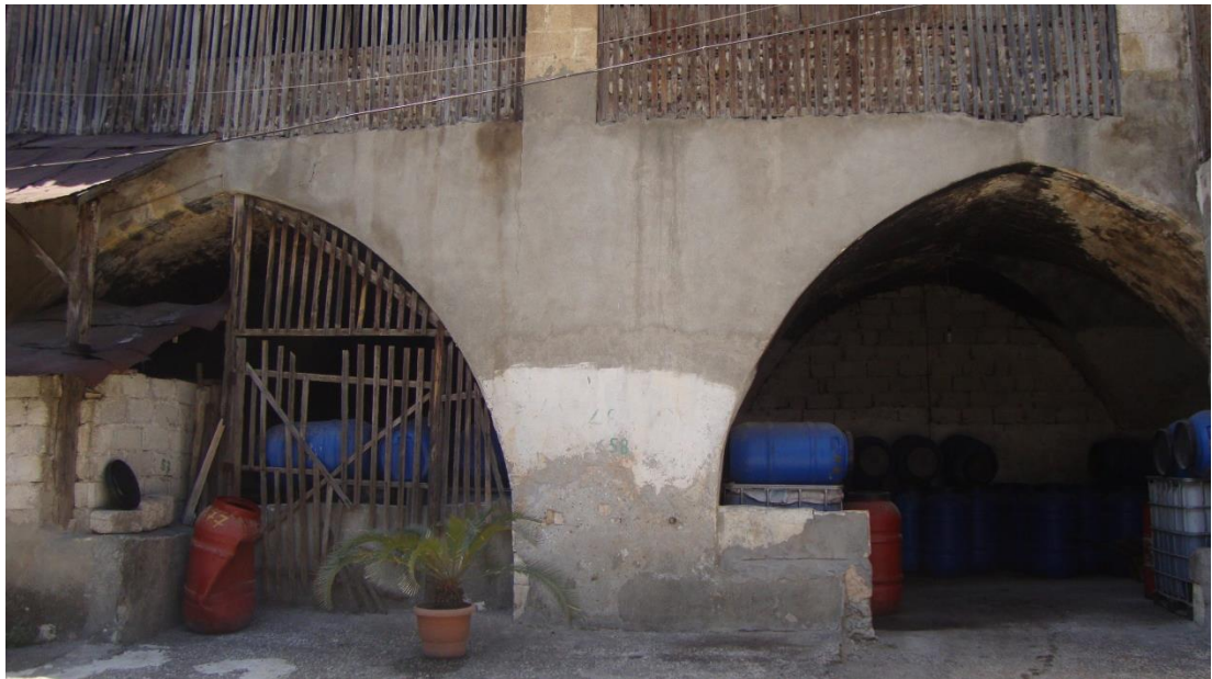
Figure 4.111. The depressed pointed arches on the courtyard facade
