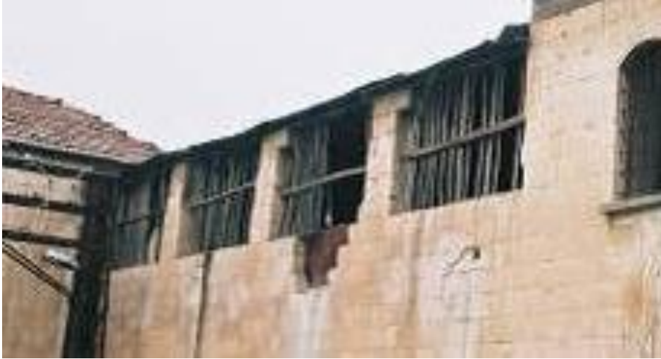
Figure 5.102. The wooden screen between cut stone masonry columns on the street facades of the spreading and drying area in Sayınlar Soap Factory, Nizip
