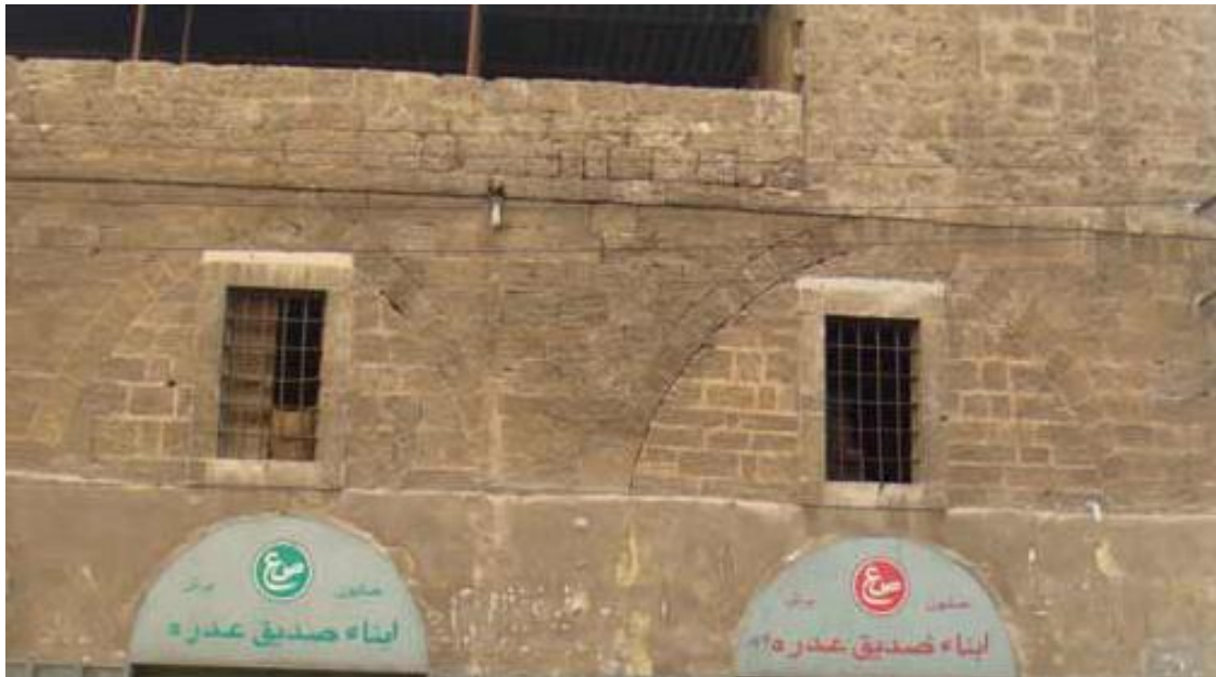
Figure 5.73. The depressed pointed arches on the street facade on the first floor in Sadık Adra Soap Factory, Tripoli
