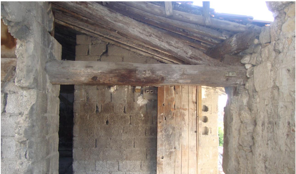
Figure 4.156. Decay on the wooden hipped roof
