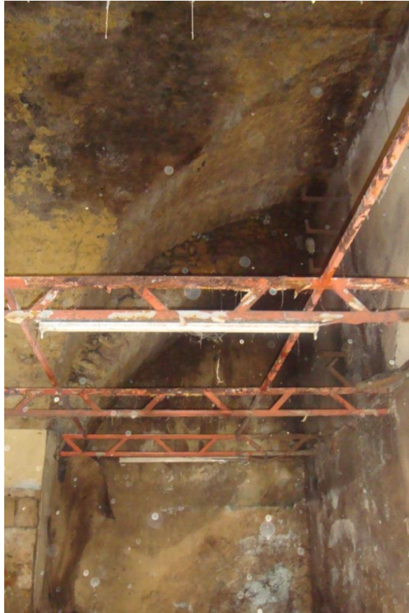
Figure 4.153. Microbiological colonization on the vault
