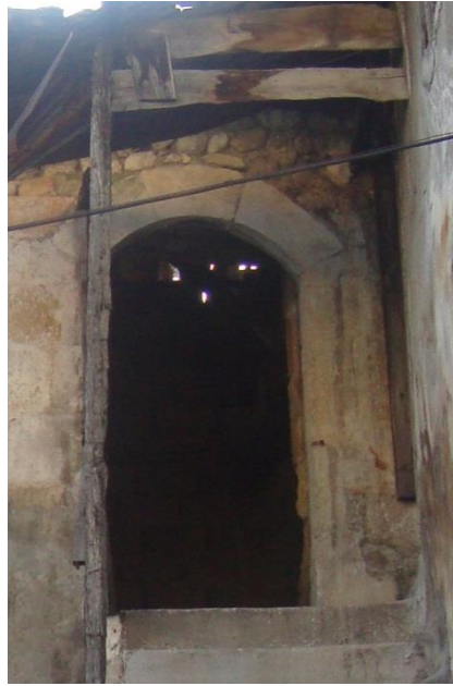
a) b) Figure 5.88. The depressed arched entrance door opening with stone casing on the courtyard facade on the first floor: a) View from the outside; b) View from the inside;
