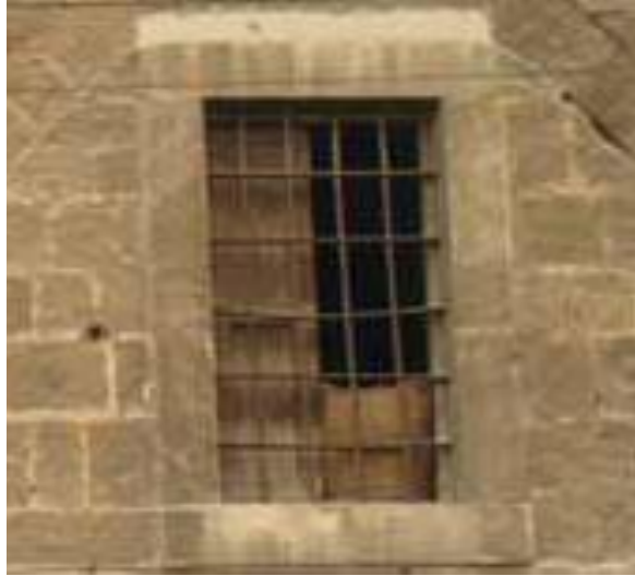
Figure 5.97. The vertical rectangular window openings with stone casing, grilled iron bars and inner wooden shutters on the first floor in Sadık Adra Soap Factory, Tripoli
