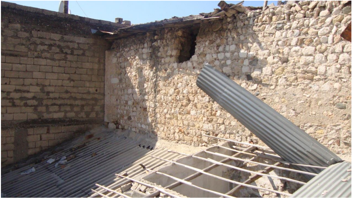
Figure 5.57. The rubble stone masonry wall on the west part of the building
