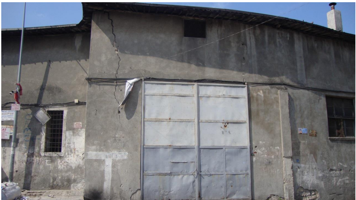
Figure 4.87. The later added double-winged iron door
