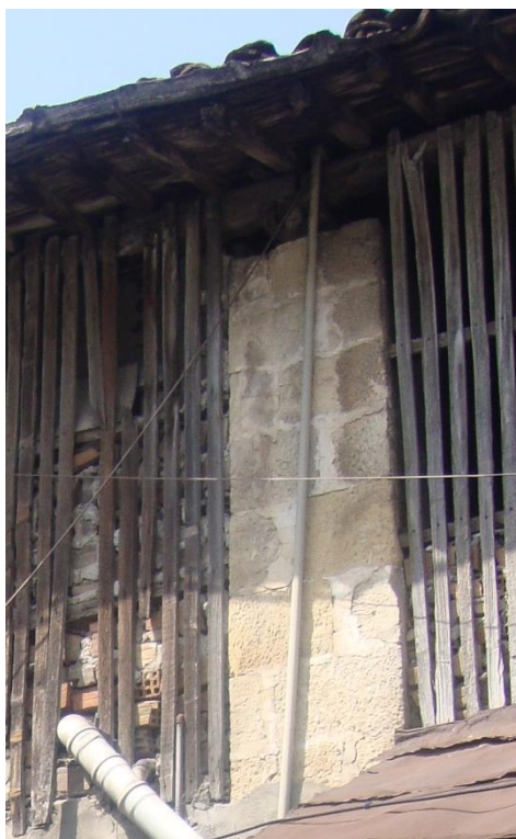
Figure 4.149. Detachment of a light colored crust changing the surface on the cut stone masonry column on the western courtyard facade
