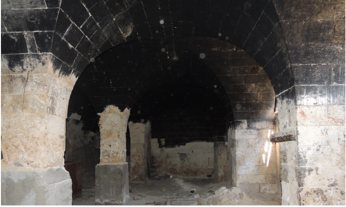
Figure 5.27. The closed gallery covered with cross vault on the ground floor of Sayınlar Soap Factory, Nizip
