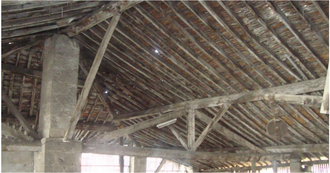
Figure 4.157. Natural aging on the wooden hipped roof
