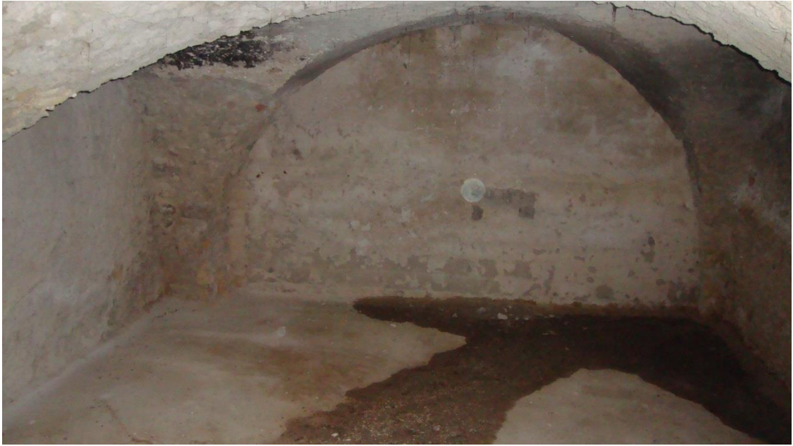
Figure 5.47. The fireplace room covered with cross vault and located below the stone cauldron on the basement floor in Selahattin Ökten Soap Factory, Antakya
