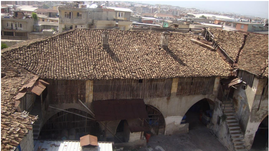
Figure 5.77. The hipped roof covered with over and under tiles in Kuseyri Soap Factory, Antakya
