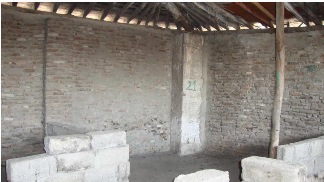
Figure 4.39. Brick wall between the original cut stone masonry columns on the northeastern part of the drying area
