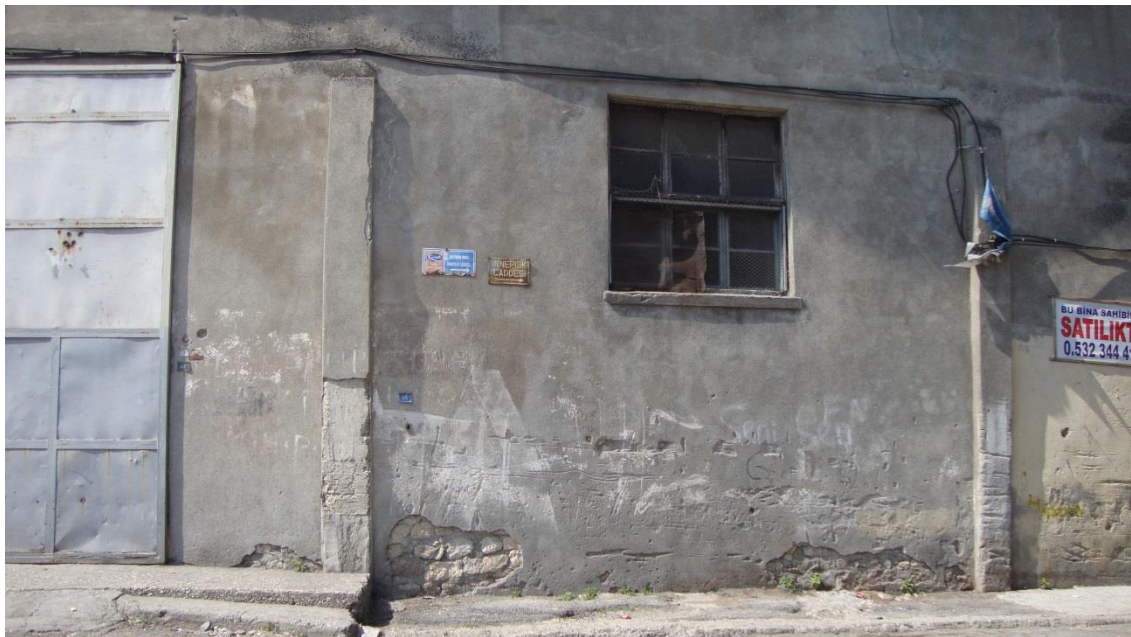
Figure 4.89. The later arranged square wooden sash window and reinforced concrete columns on the northern facade
