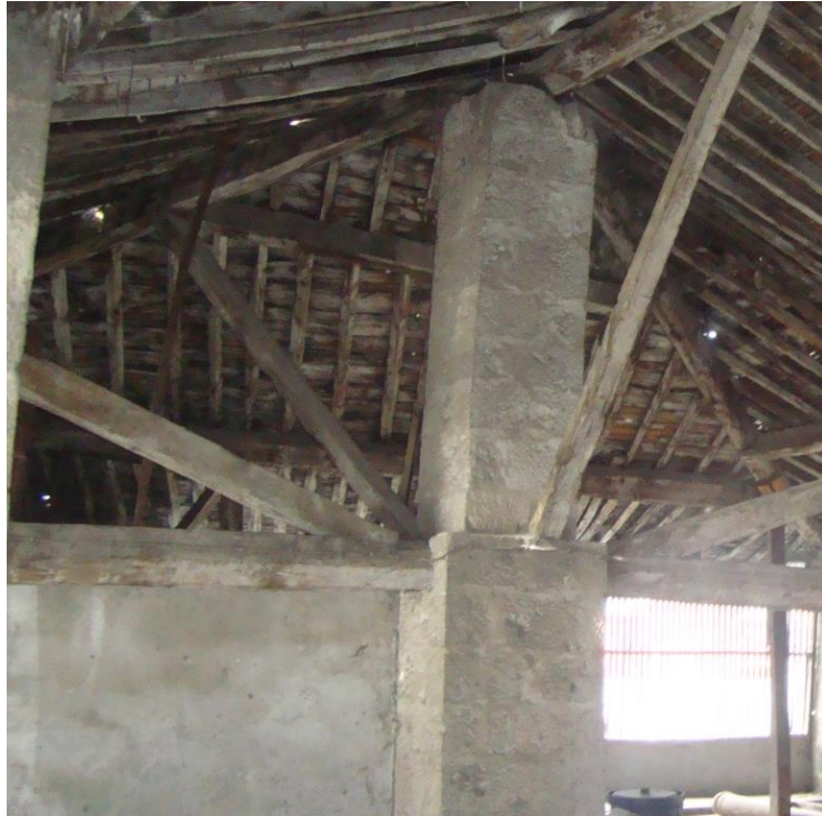
Figure 4.151. Efflorescences on the cut stone masonry columns on the spreading area
