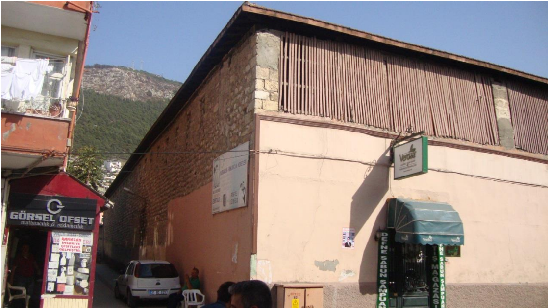
Figure 5.39. The stone masonry wall on the adjacent facade of the spreading and drying area in Selahattin Ökten Soap Factory, Antakya
