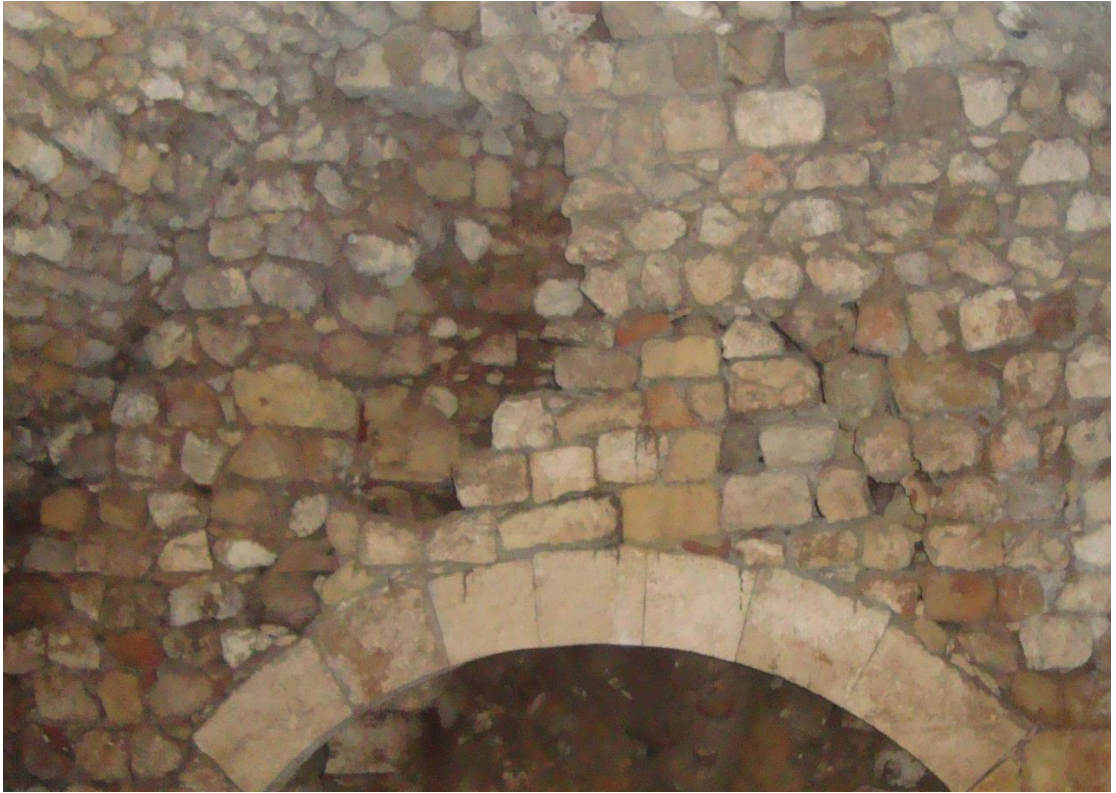
Figure 4.155. Loss of material and cracks on the fireplace on the basement floor
