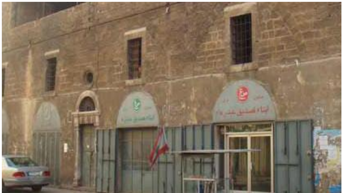
Figure 5.87. The semicircular arched entrance openings on the entrance facade on the ground floor in Sadık Adra Soap Factory, Tripoli
