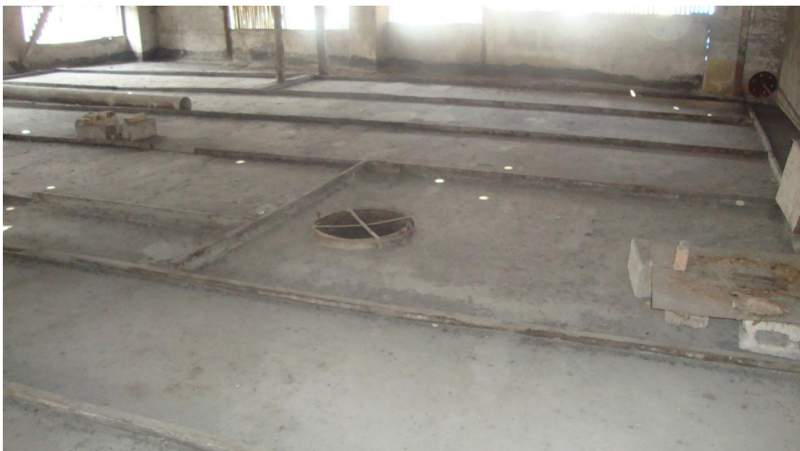
Figure 4.126. View of the later arranged circular hole from the floor of the spreading area on the first floor
