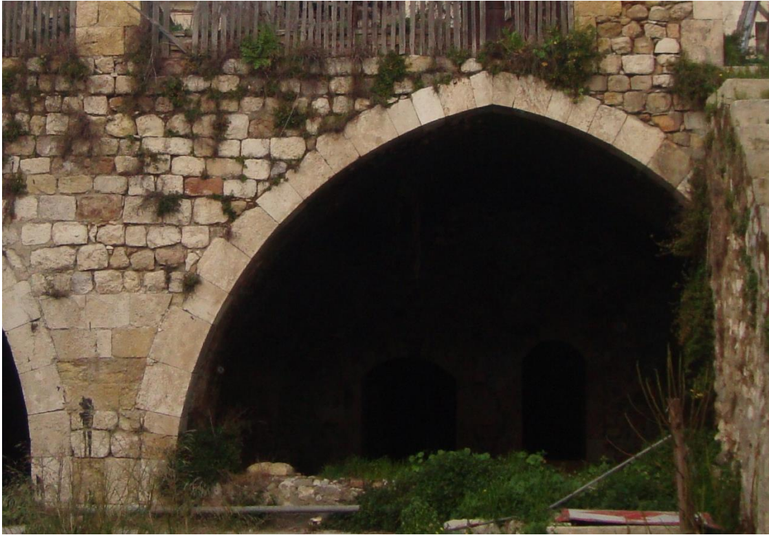
Figure 5.69. The depressed pointed arch on the courtyard facade in Aselci Soap Factory, Antakya
