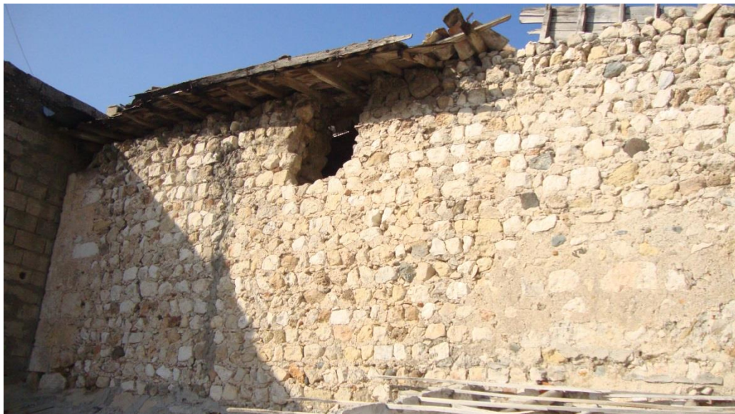
Figure 4.102. The rubble stone masonry wall on the west part of the building
