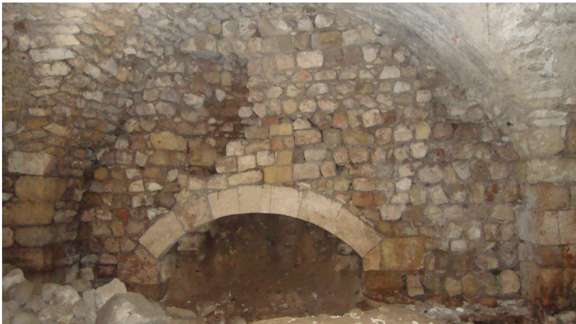
Figure 4.32. Depressed arched fireplace located on the southern wall of the fireplace room
