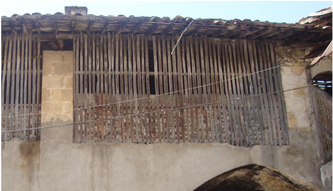
Figure 5.67. The cut stone masonry columns on the courtyard facade of the spreading area in Kuseyri Soap Factory, Antakya
