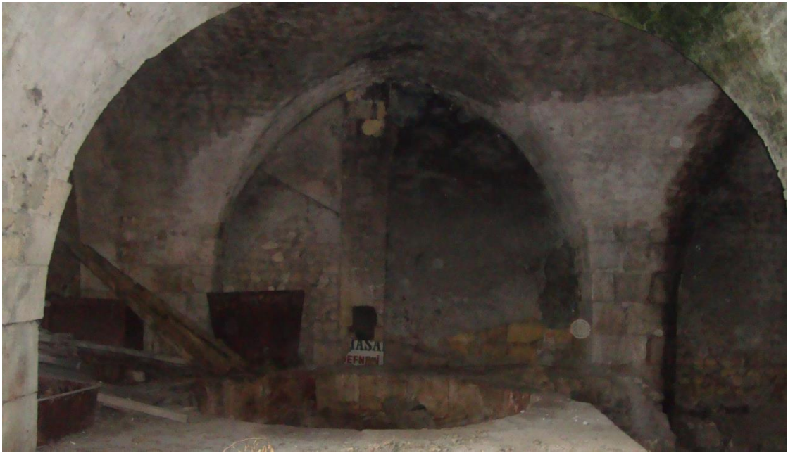
Figure 5.117. The cut stone masonry chimney rising from the fireplace room on the basement floor adjacent to the stone cauldron on the ground floor in Aselci Soap Factory, Antakya
