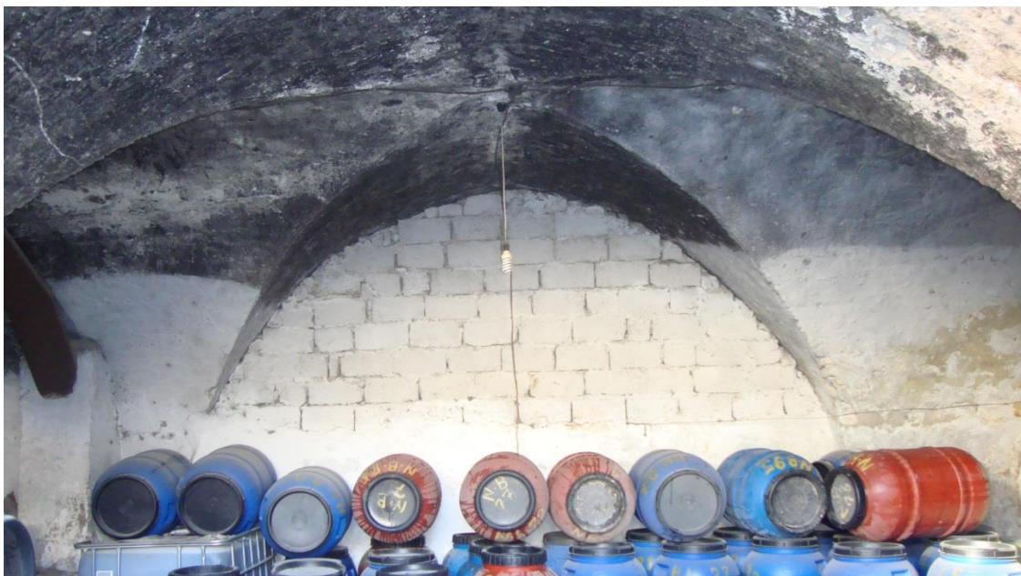
Figure 4.136. One of the later added cinder block masonry wall that divide the building into two parts on the ground floor
