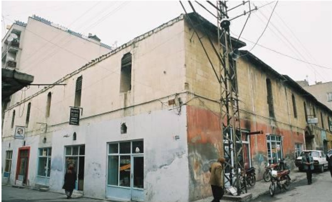
Figure 5.41. The stone masonry wall on the street facades of the spreading and drying areas in Fincancıoğlu Soap Factory, Nizip
