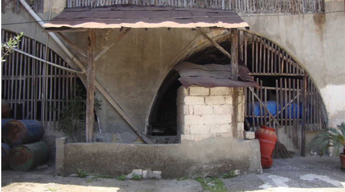
Figure 4.74. Partially removed wooden screen in the depressed pointed arch and mass addition on the western courtyard facade
