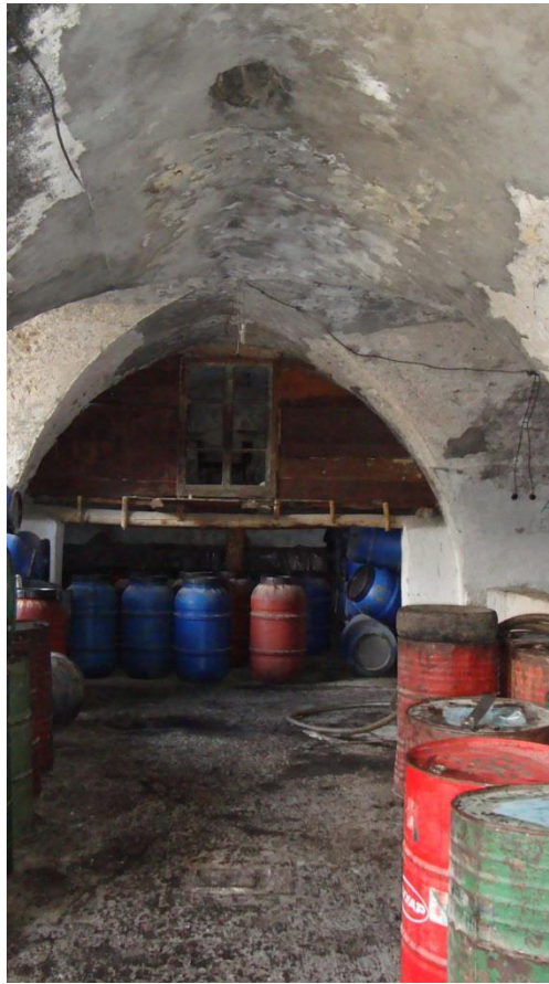
Figure 4.143. The traces of the cut stone masonry chimney on the floor and cross vault of the semi-open gallery on the ground floor
