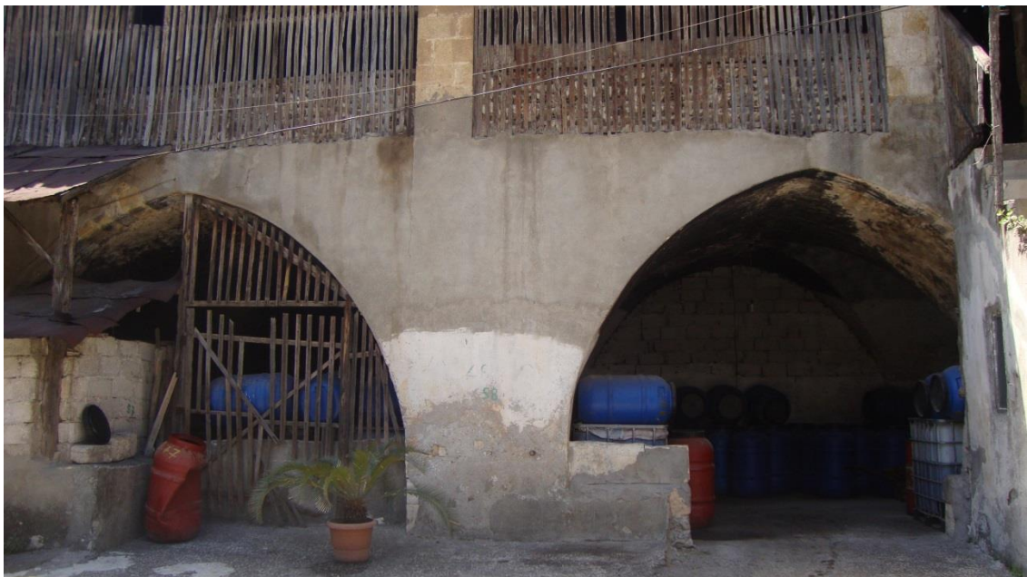
Figure 4.75. The northern depressed pointed arch on the western courtyard facade
