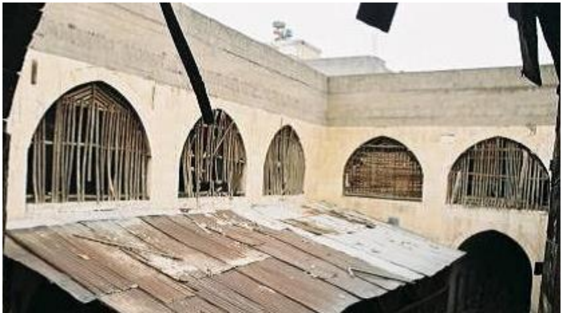
Figure 5.101. The wooden screen between depressed pointed arches on the courtyard facades of the spreading and drying area in Sayınlar Soap Factory, Nizip
