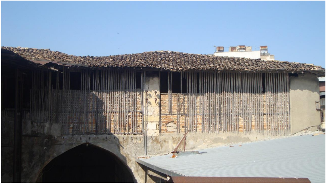
Figure 4.40. The original wooden screen and later added low partition brick masonry walls between the original cut stone masonry columns on the south part of the drying area
