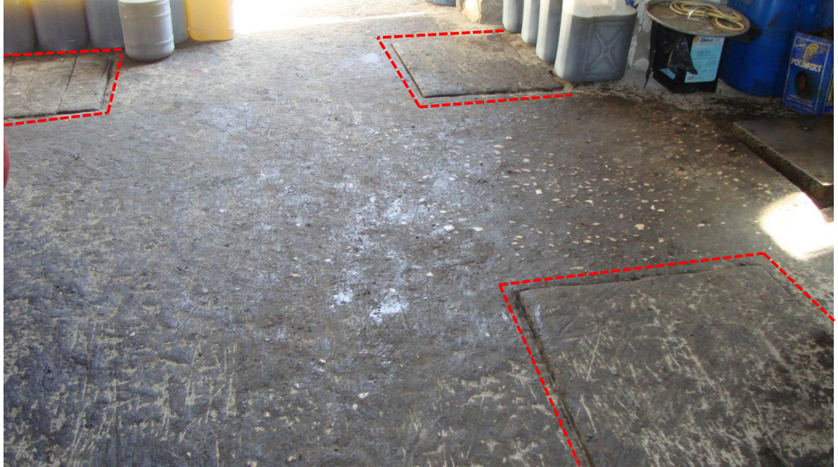
Figure 4.16. The tracks of the wooden shutters of the original circular olive oil wells buried on the ground of L shaped semi-open gallery
