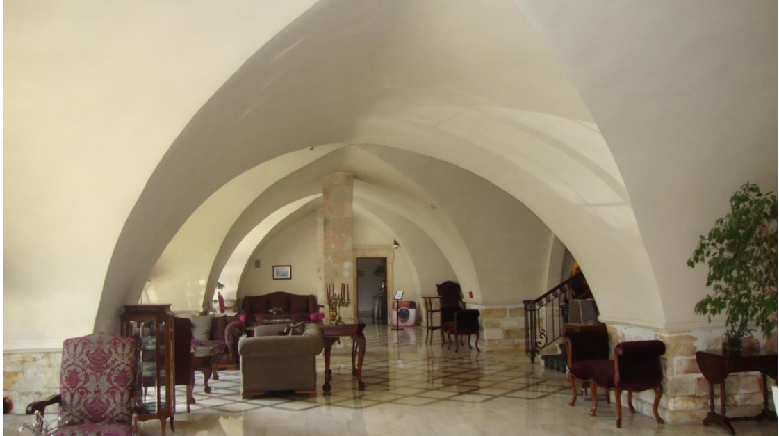
Figure 5.75. The cross vault on the ground floor in Şeyhoğlu Soap Factory, Antakya
