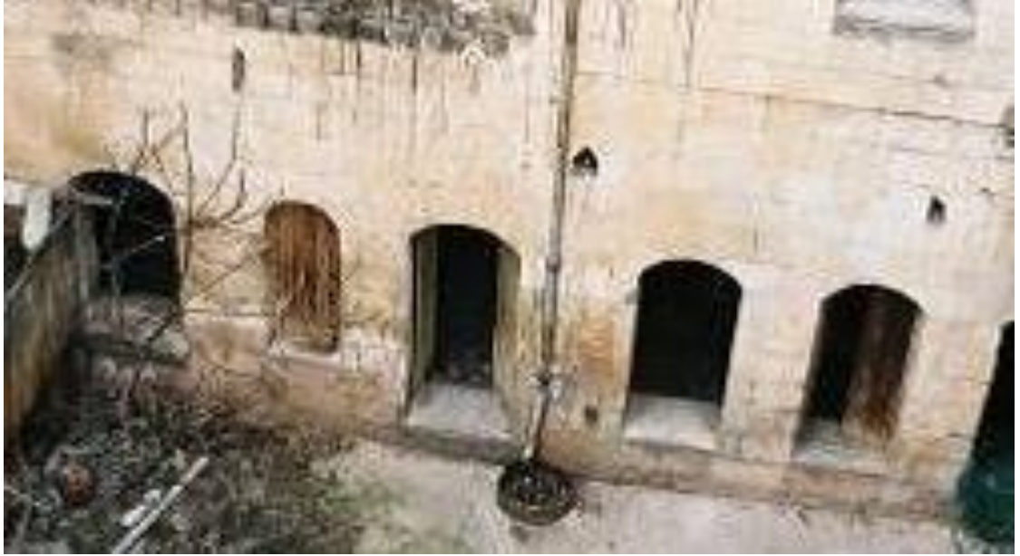
Figure 5.84. The depressed arched door and window openings of the accommodation units opening to the courtyard in Sayınlar Soap Factory, Nizip
