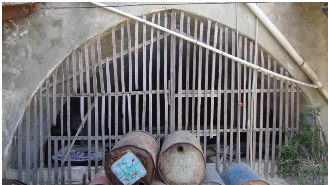
Figure 5.71. The depressed pointed arch on the courtyard facade on the ground floor in Kuseyri Soap Factory, Antakya
