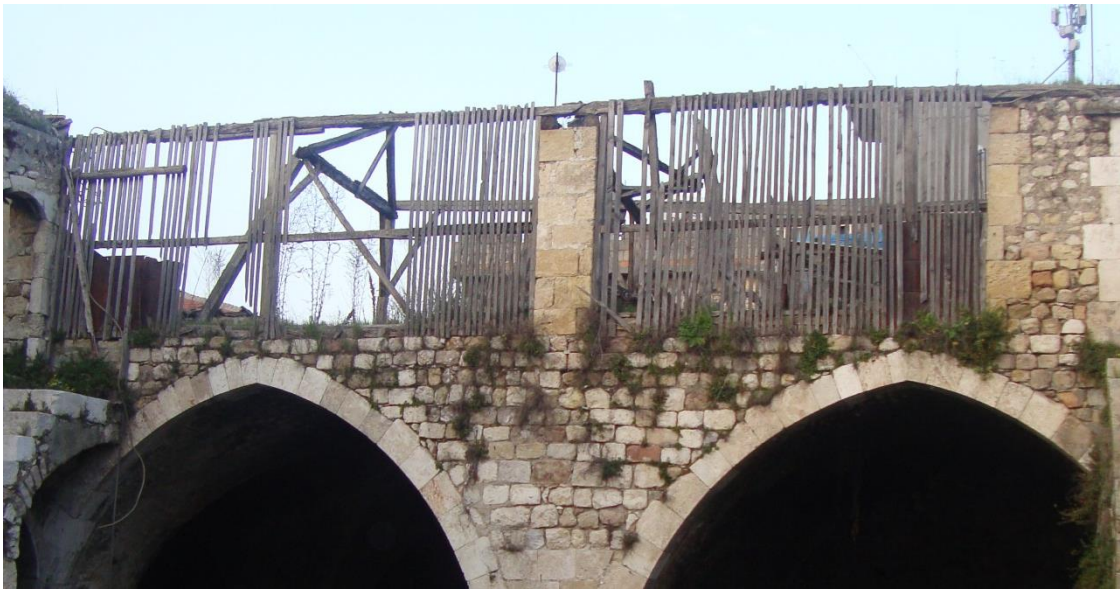
Figure 5.35. The wooden screen on the courtyard façade of the spreading and drying area in Aselci Soap Factory, Antakya
