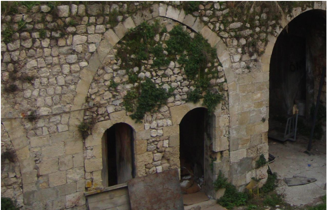
Figure 5.91. The vertical rectangular depressed arched window opening of the office looking onto the courtyard in Aselci Soap Factory, Antakya
