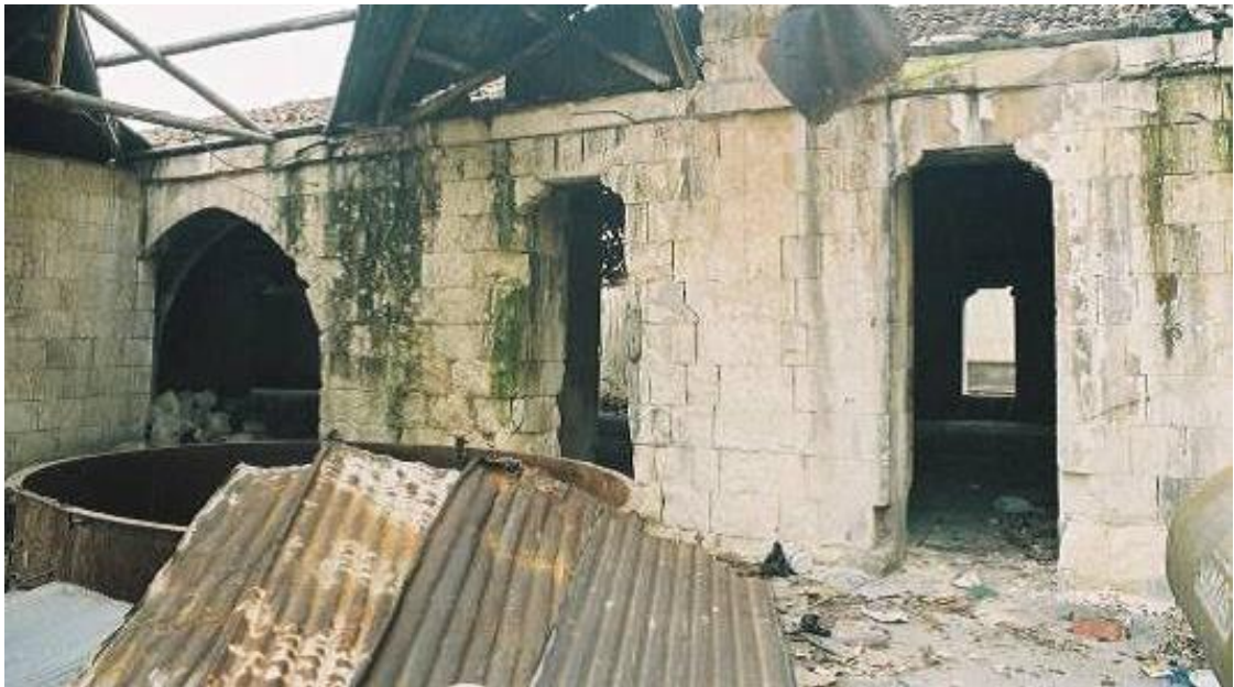
Figure 5.58. The cut stone masonry wall without plaster on the first floor in Fincancıoğlu Soap Factory, Nizip
