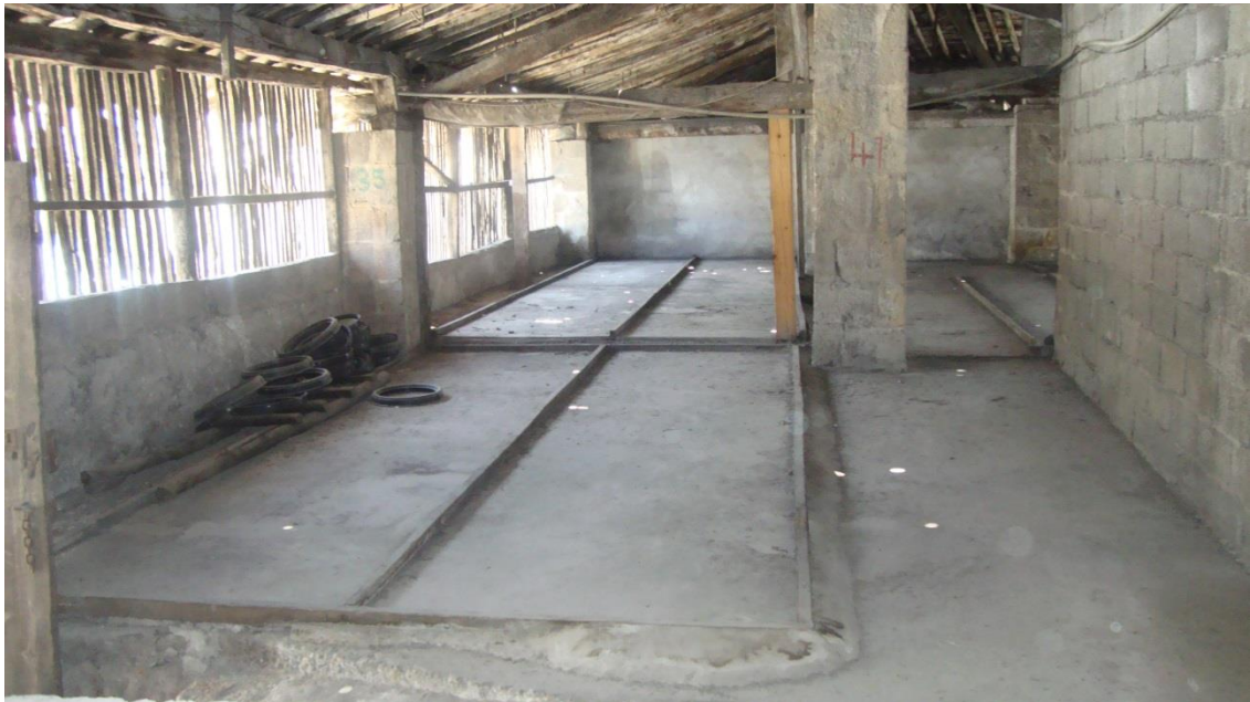
Figure 4.44. The spreading area with original wooden screen and later added low partition brick walls between three cut stone masonry columns on its courtyard facade
