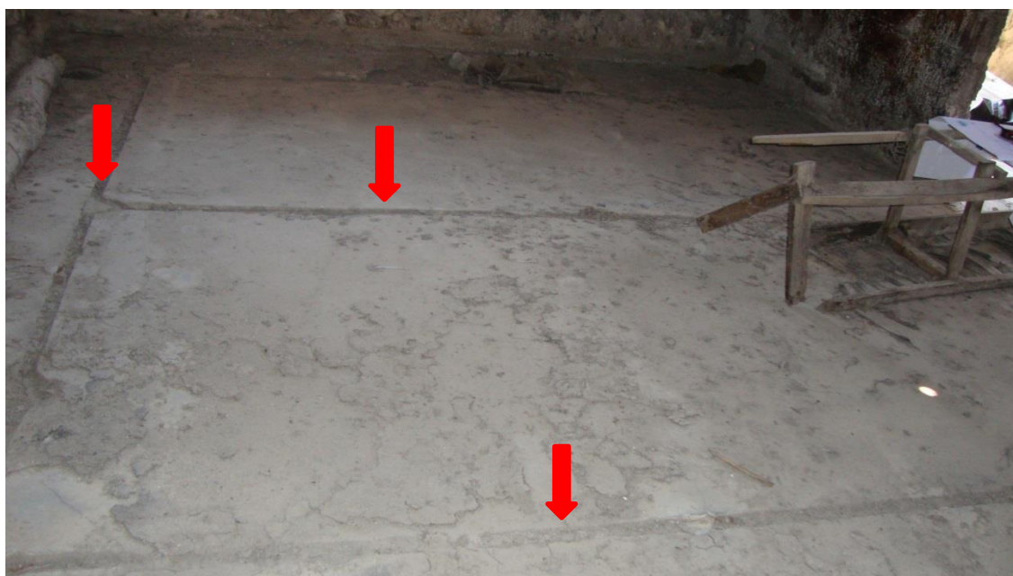
Figure 4.69. Traces of the wooden laths of the soap molds on the floor
