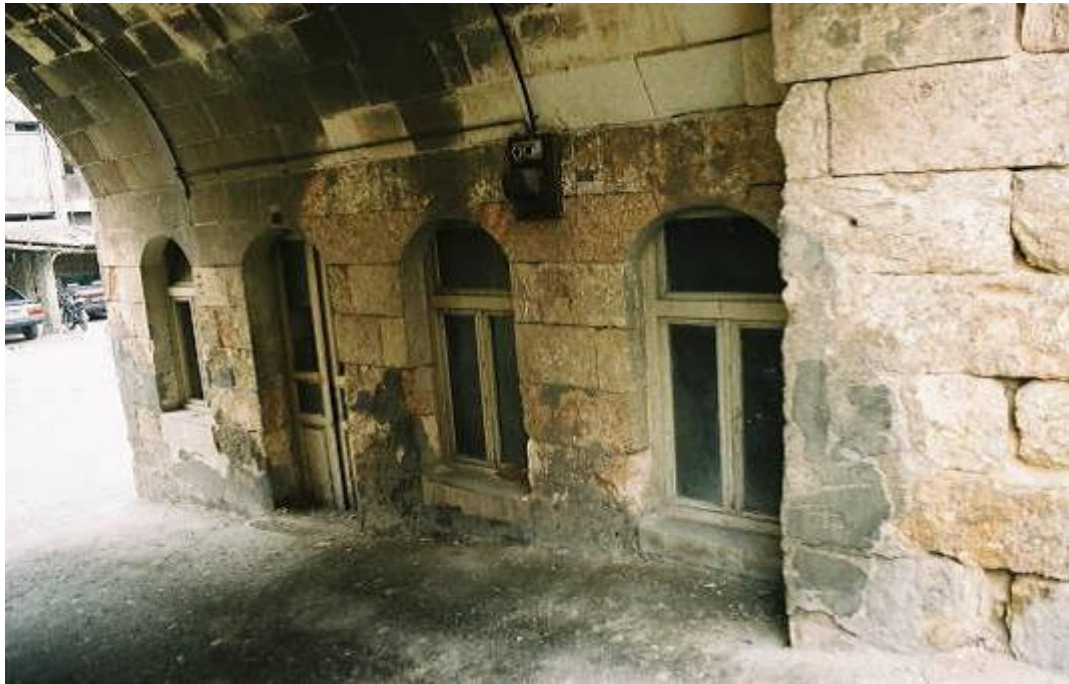
Figure 5.83. View of the depressed arched door and window openings of the office connected to the semi-open entrance space in Fincancıoğlu Soap Factory, Nizip
