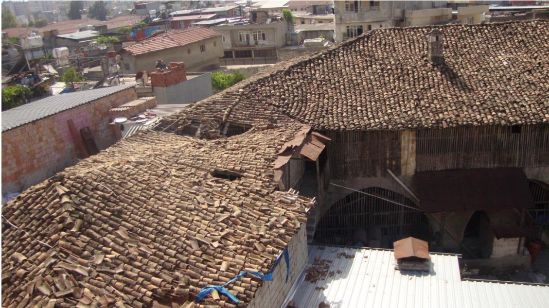
Figure 4.52. Partially collapsed part of the roof
