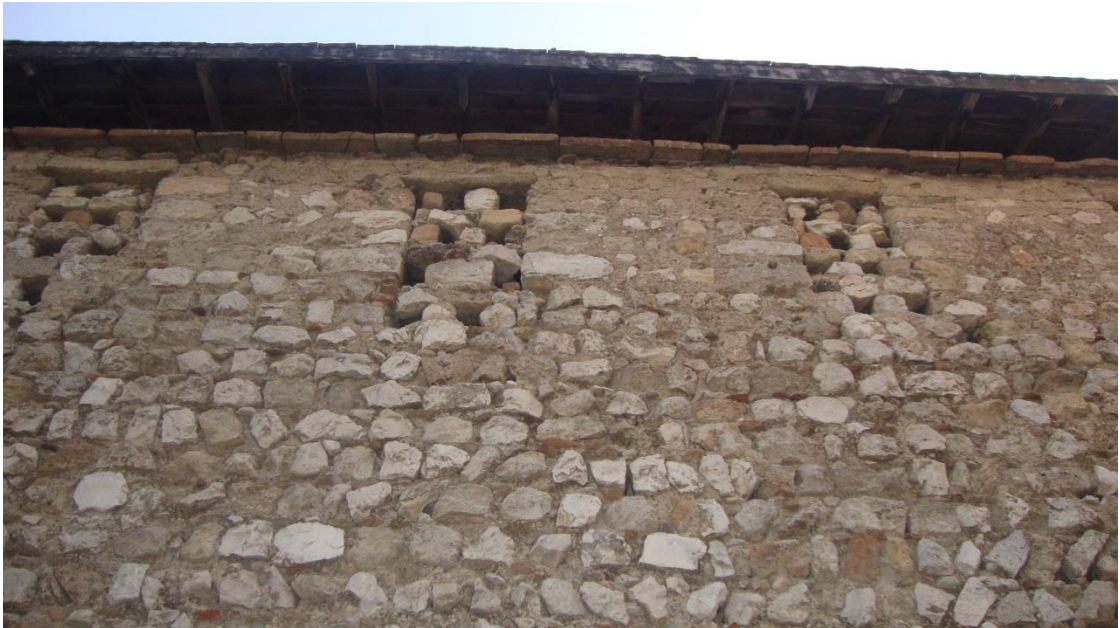
Figure 5.93. The vertical rectangular window openings on the stone masonry wall on the adjacent facade of the spreading and drying area in Selahattin Ökten Soap Factory, Antakya
