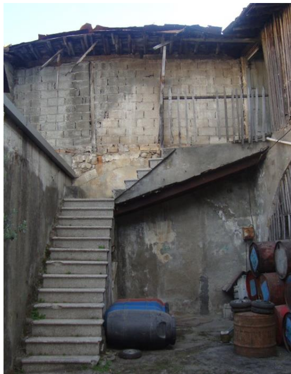
Figure 4.35. The later added quarter landing reinforced concrete stair
