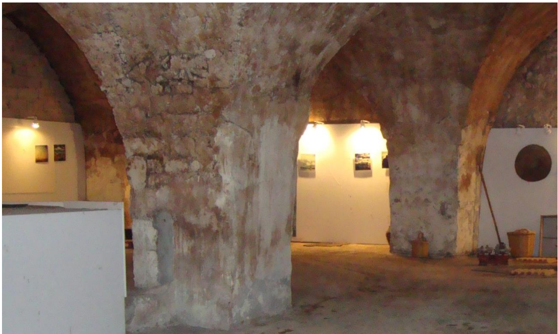
Figure 5.61. The cut stone masonry piers on the closed gallery on the ground floor in Selahattin Ökten Soap Factory, Antakya
