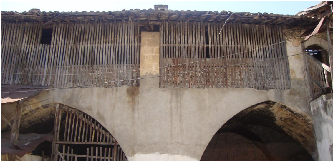
Figure 4.77. The wooden screen between the cut stone masonry columns on the first floor of the western courtyard facade
