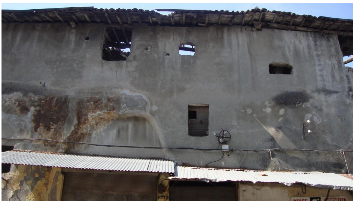
Figure 4.90. Later arranged window openings without joinery on the upper part of the northern facade
