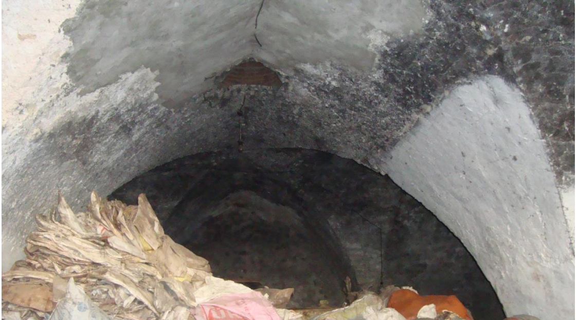
Figure 5.122. The later arranged circular hole for carrying the liquid soap on the vault of the closed gallery in Kuseyri Soap Factory, Antakya
