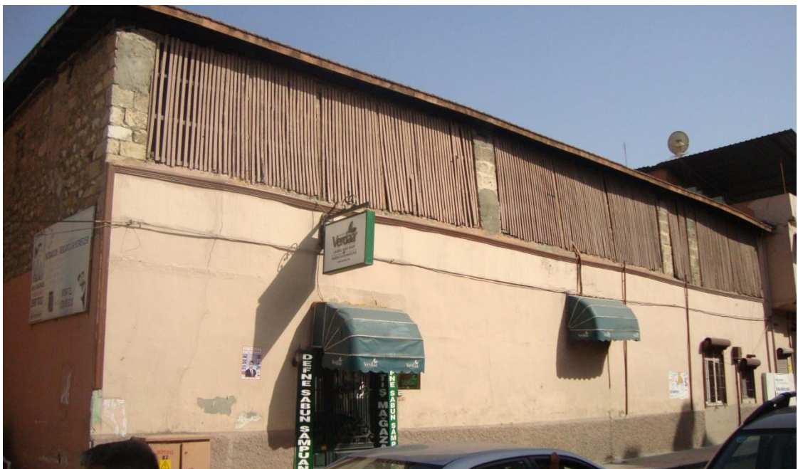
Figure 5.99. The wooden screen on the street facade of the spreading and drying area in Selahattin Ökten Soap Factory (at present Verdaa Soap Factory), Antakya
