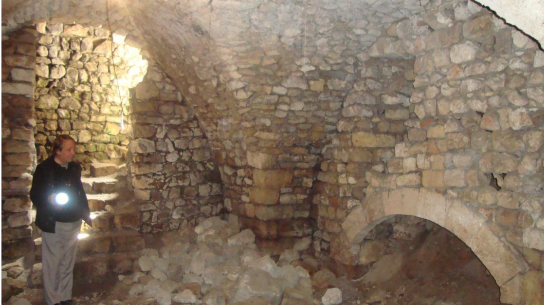
Figure 5.48. The fireplace room covered with cros vault, located on the asement floor and accessed from the courtyard by stone stair in Kuseyri Soap Factory, Antakya
