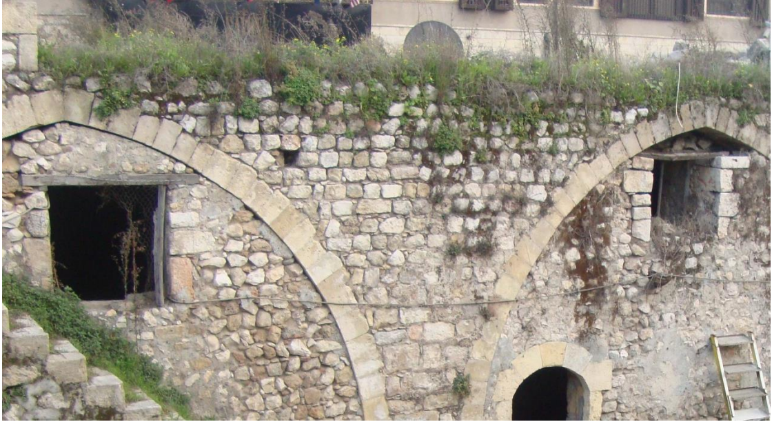
Figure 5.92. The top window openings without frame on the courtyard facade in Aselci Soap Factory, Antakya
