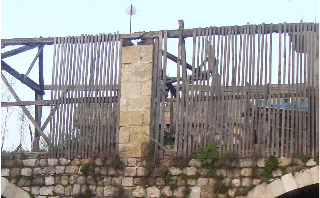
Figure 5.66. The cut stone masonry columns on the courtyard facade of the spreading area in Aselci Soap Factory, Antakya
