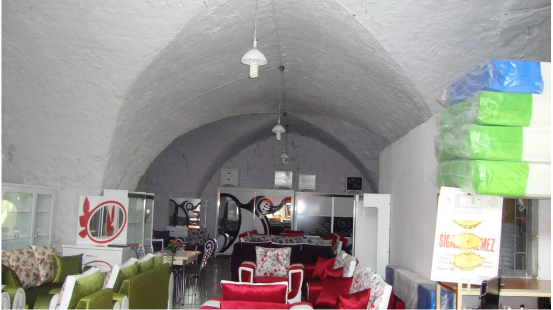
Figure 5.25. The gallery covered with cross vault on the ground floor of Hasan Ökten Soap Factory, Antakya
