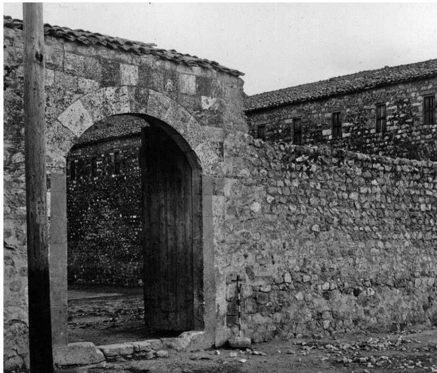
Figure 5.81. The double winged wooden door of the entrance space in stone casing and depressed arched door opening in Kuseyri Soap Factory, Antakya (Source: Princeton University, n.d.)
