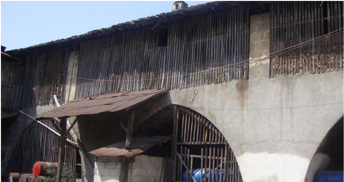
Figure 5.37. The wooden screen on the courtyard facade of the spreading and drying area in Kuseyri Soap Factory, Antakya
