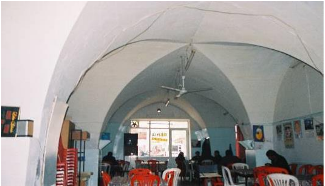
Figure 5.26. The closed gallery covered with cross vault on the ground floor of Fincancıoğlu Soap Factory, Nizip
