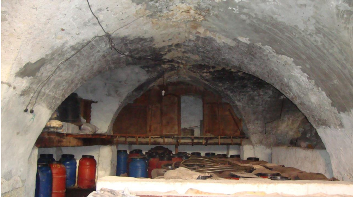
Figure 4.24. A view of closed gallery covered with cross vault
