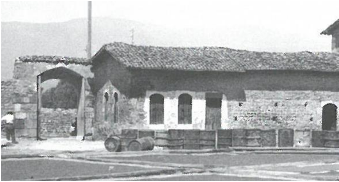
Figure 5.90. The vertical rectangular depressed arched window openings of the office looking onto the courtyard and entrance space in Selahattin Ökten Soap Factory, Antakya
