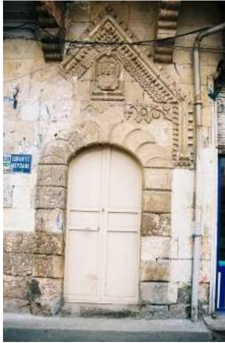
Figure 5.86. The depressed arched door opening of the stair hall accessed directly from the street in Sayınlar Soap Factory, Nizip
