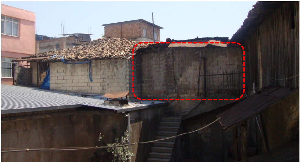
Figure 4.131. The later arranged cinder block masonry wall on the southern courtyard facade on the first floor
