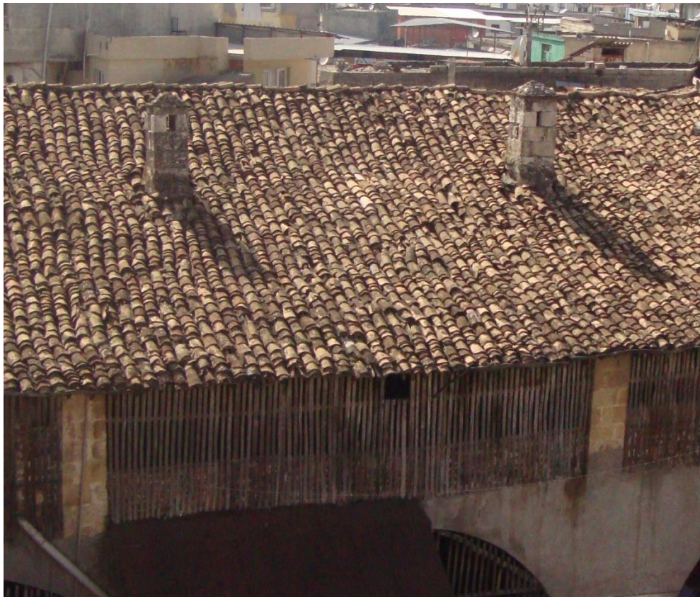
Figure 4.123. The original cut stone masonry chimney rising from the fireplace room to the roof
