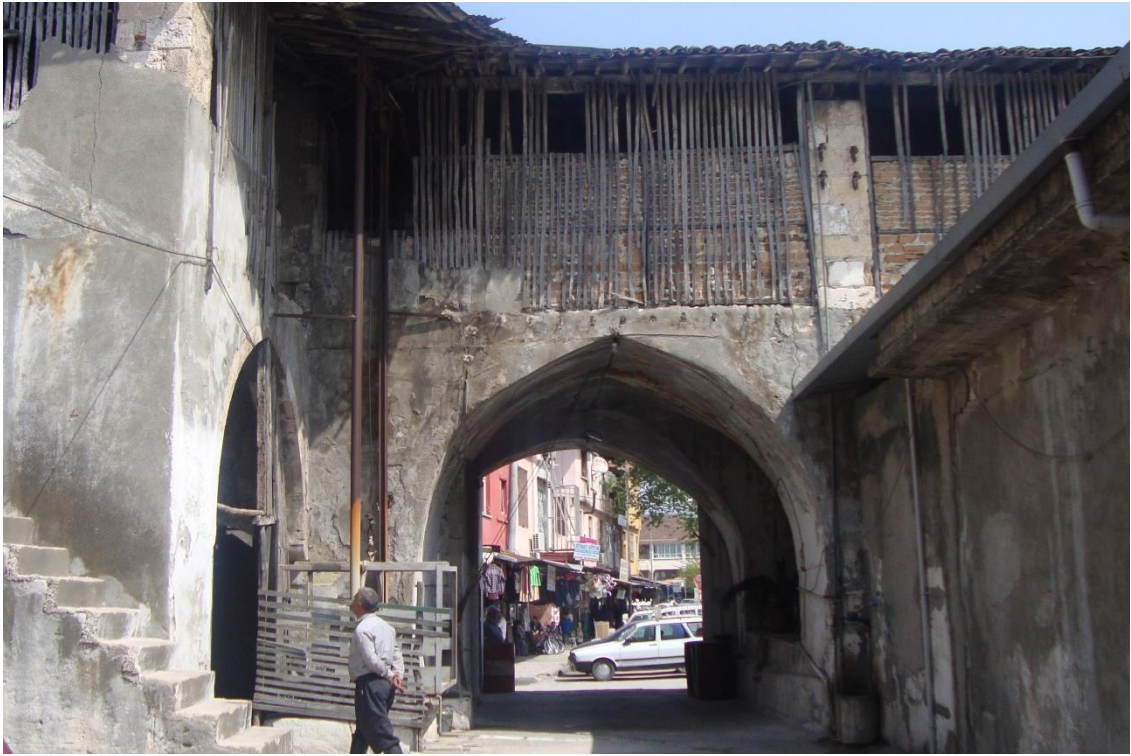
Figure 4.82. The depressed pointed arch of the later arranged semi-open entrance space
