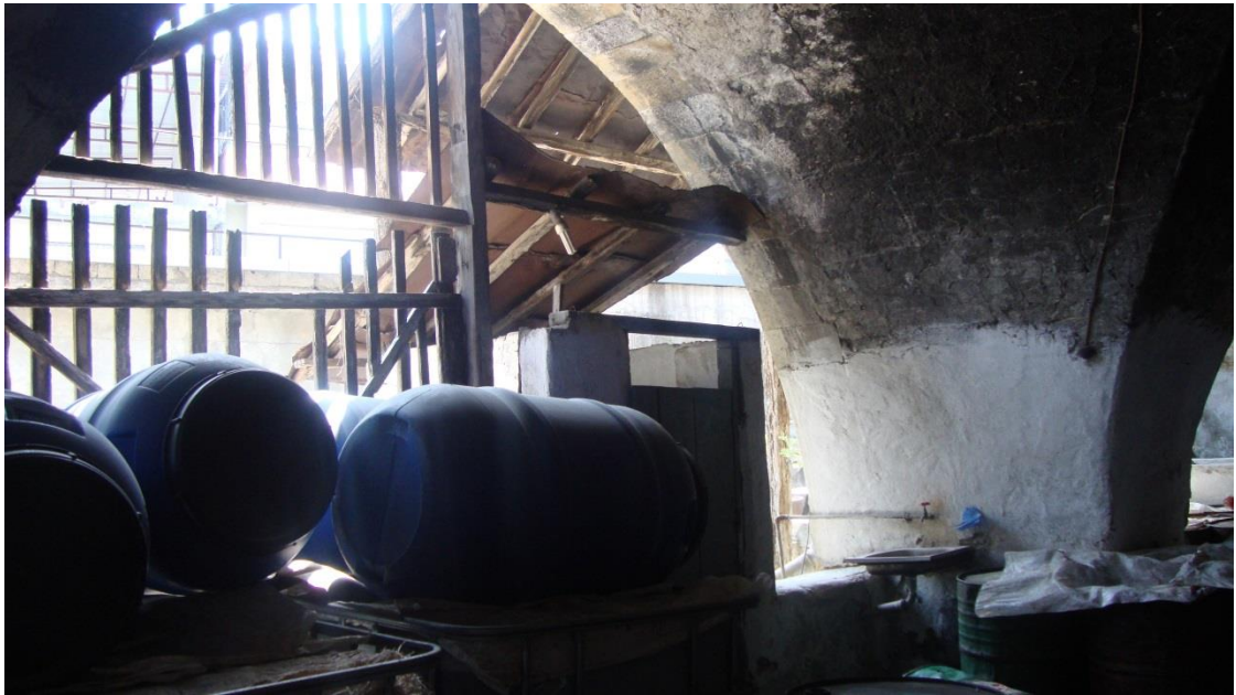
Figure 4.145. The removed part of the wooden screen on the courtyard facade of the semi-open gallery on the ground floor
