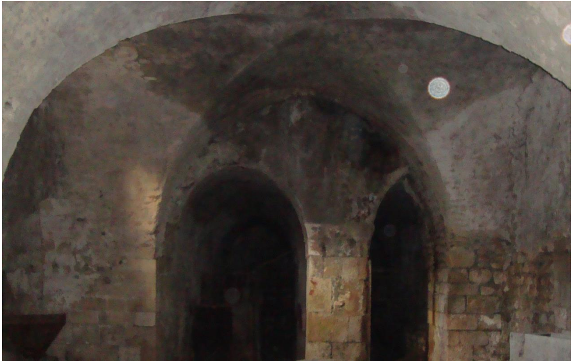
Figure 5.74. The cross vault on the ground floor in Aselci Soap Factory, Antakya
