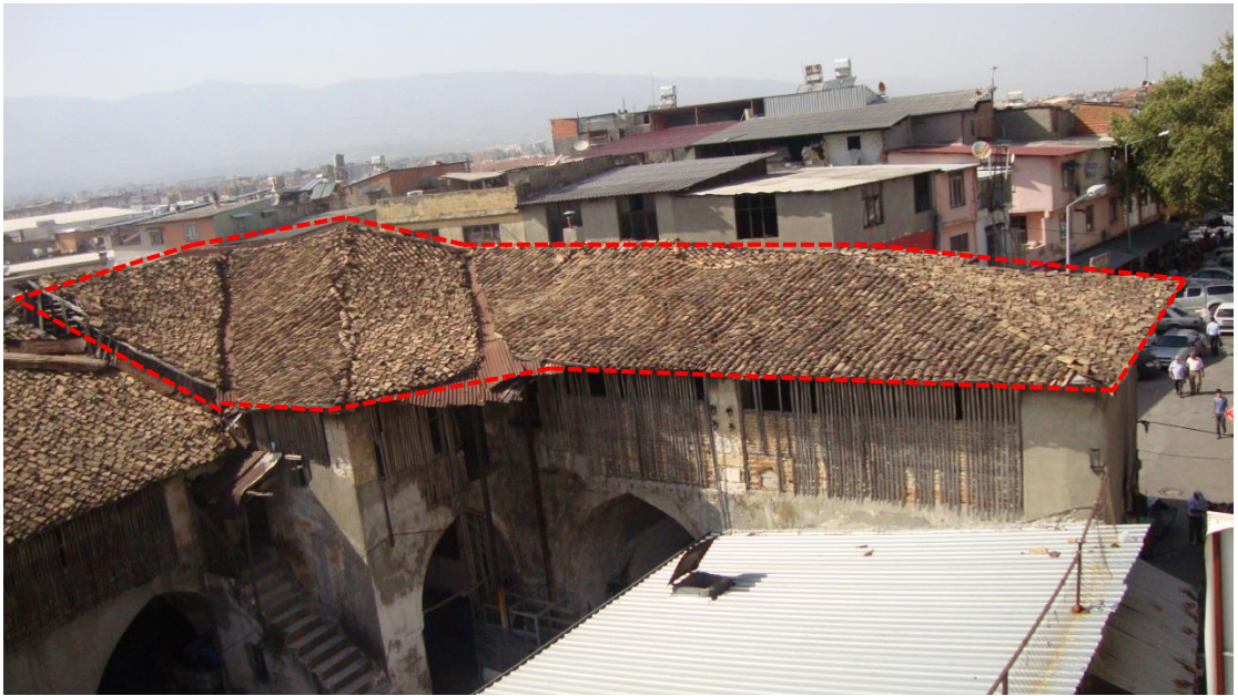
Figure 4.106. The renewed part of the hipped roof on the north of the building
