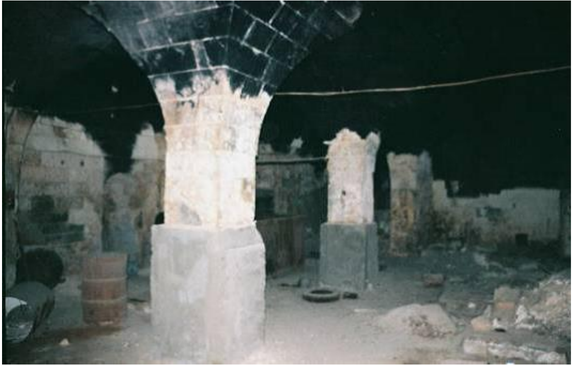
Figure 5.64. The cut stone masonry piers on the closed gallery on the ground floor in Sayınlar Soap Factory, Nizip
