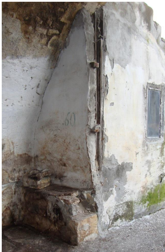
Figure 4.146. The traces of the removed low partition stone wall and wooden screen on the depressed pointed arch of the northern semi-open gallery
