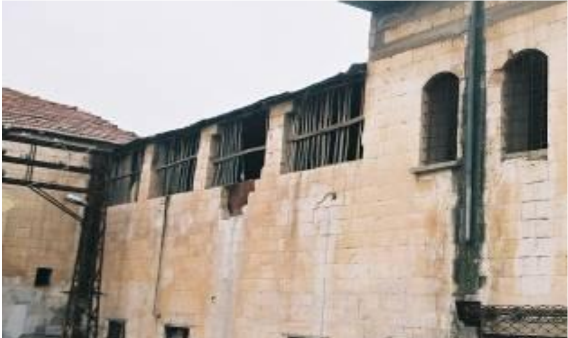
Figure 5.68. The cut stone masonry columns on the street facade of the spreading and drying area in Sayınlar Soap Factory, Nizip
