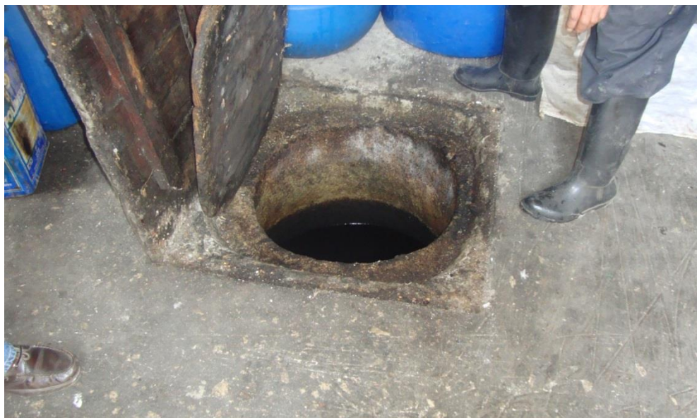
Figure 4.120. The original circular olive oil well buried beneath the ground of the semi-open gallery on the ground floor
