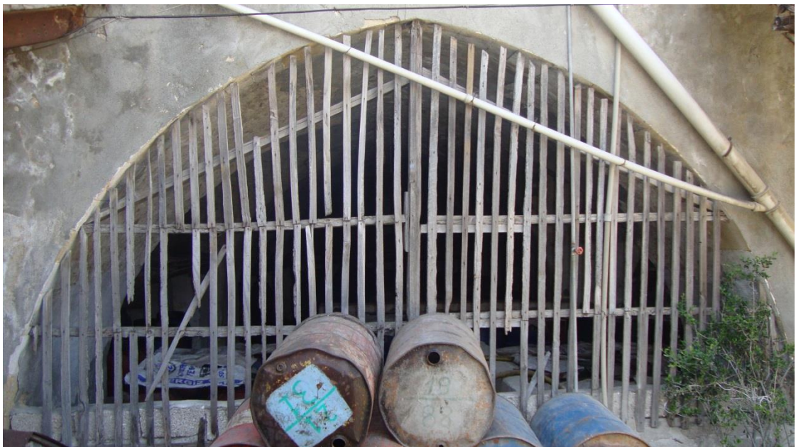
Figure 4.140. The renewed wooden screen between depressed pointed arch of the semi-open gallery on the courtyard facade
