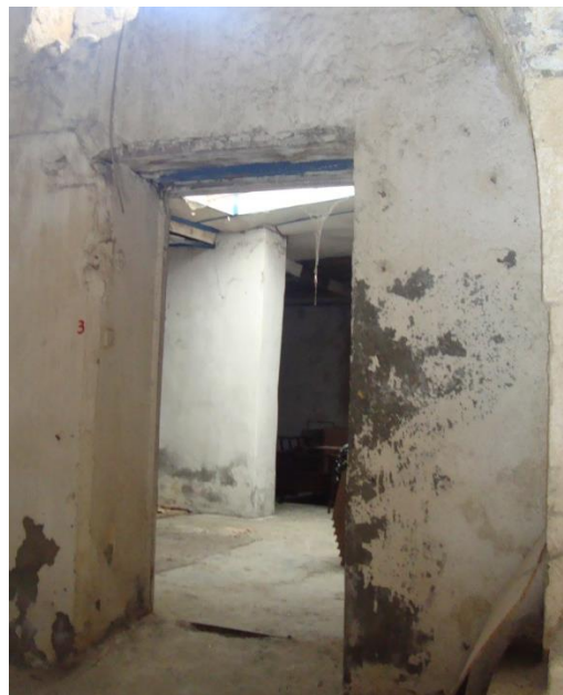
Figure 5.89. The original door opening on the stone masonry wall on the west part of the building in Kuseyri Soap Factory, Antakya
