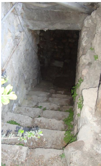
Figure 5.103. The quarter landing stone stair of the fireplace room located on the basement floor in Kuseyri Soap Factory, Antakya
