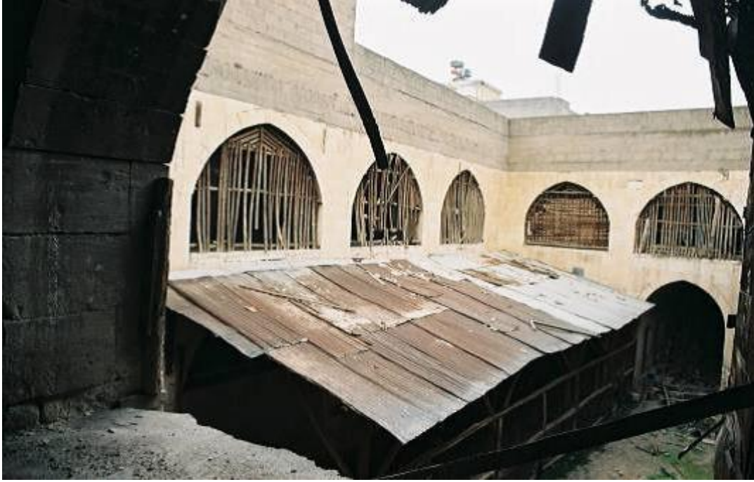
Figure 5.42. The depressed pointed arches on the courtyard facades of the spreading and drying areas in Sayınlar Soap Factory, Nizip
