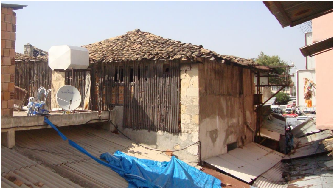
Figure 5.100. The wooden screen on the street and adjacent facades of the spreading and drying area in Kuseyri Soap Factory, Antakya
