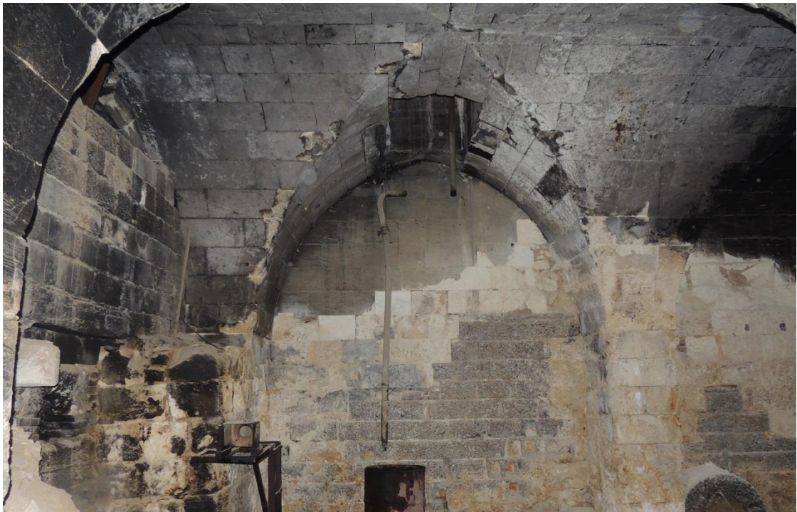
Figure 5.124. View of the rectangular hole on the vault of the closed gallery in Sayınlar Soap Factory, Nizip
