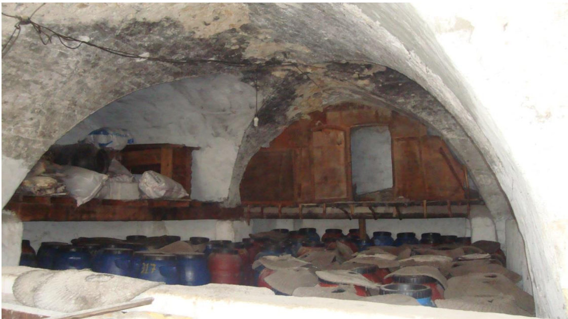
Figure 4.138. The later added wooden platforms and their pedestals on the closed gallery on the ground floor
