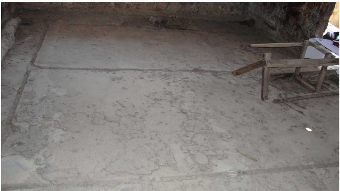
Figure 4.142. Traces of the missing wooden laths of the soap molds on the spreading and drying area on the west part of the building
