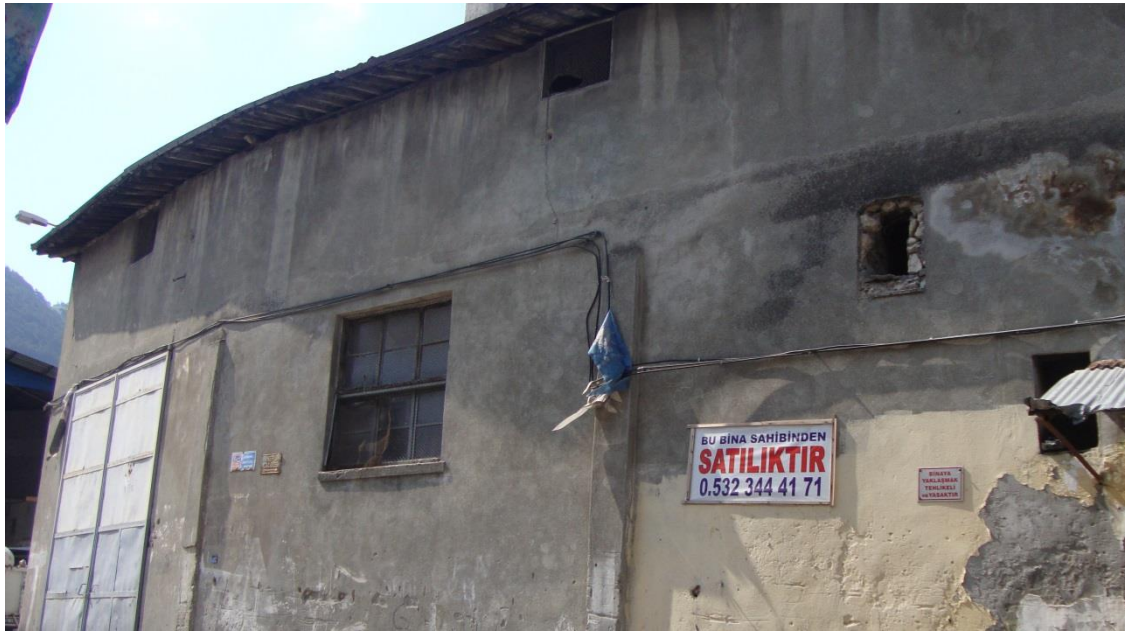
Figure 4.130. The later arranged cinder block walls on the northern facade of the spreading and drying are on the first floor
