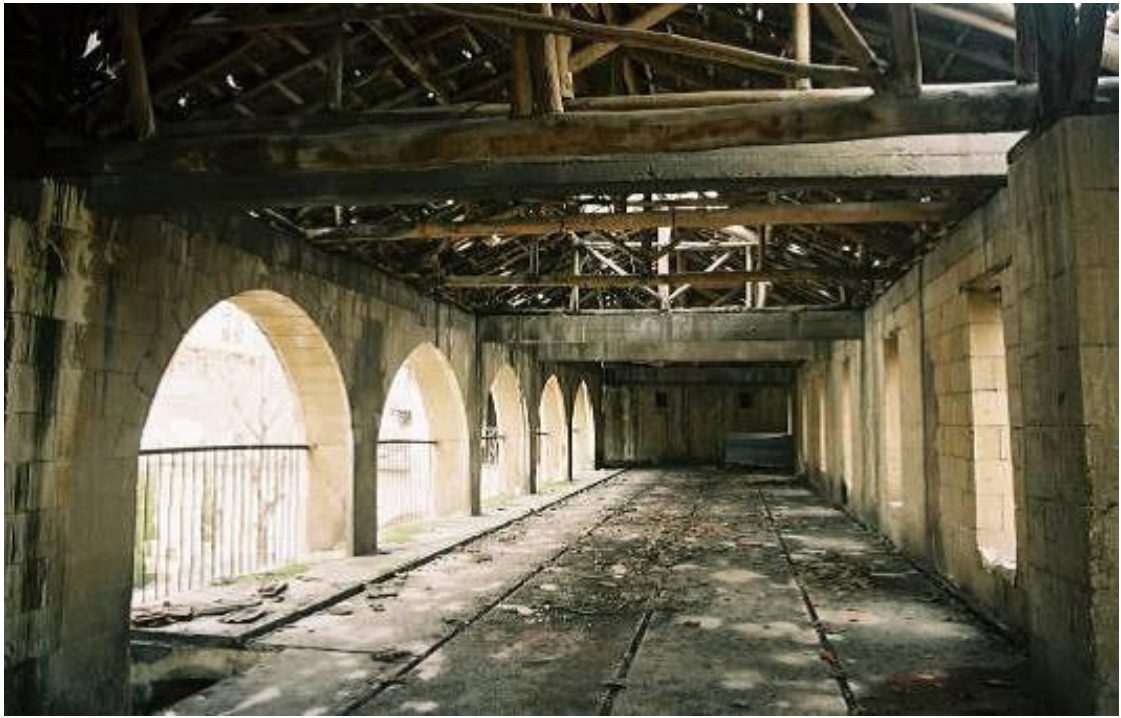
Figure 5.40. The depressed pointed arches on the courtyard facade and the stone masonry walls on the street facades of the spreading and drying areas in Fincancıoğlu Soap Factory, Nizip
