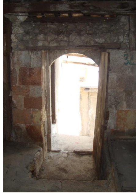
a) b) Figure 5.88. The depressed arched entrance door opening with stone casing on the courtyard facade on the first floor: a) View from the outside; b) View from the inside;
