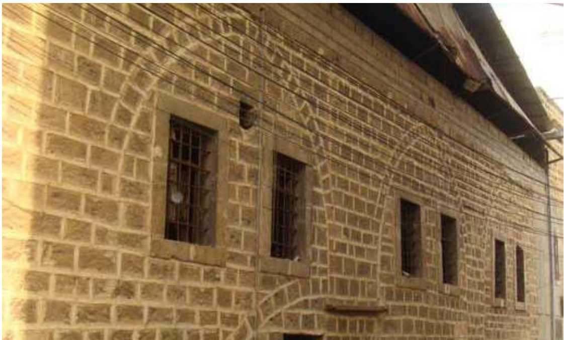
Figure 5.59. The cut stone masonry wall without plaster in Sadık Adra Soap Factory, Tripoli
