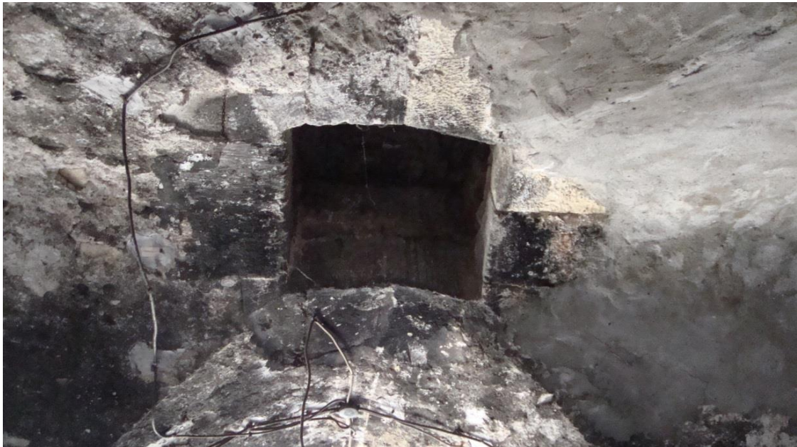
Figure 4.125. The original rectangular hole for transferring the liquid soap to the first floor on the center of the vault on the semi-open gallery
