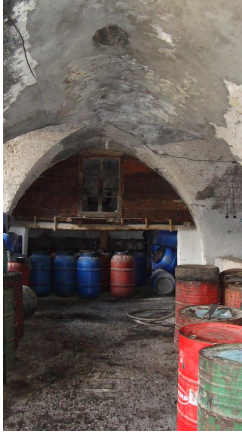
Figure 5.121. The traces of the removed part of the cut stone masonry chimney on the floor and cross vault of the semi-open gallery in Kuseyri Soap Factory, Antakya
