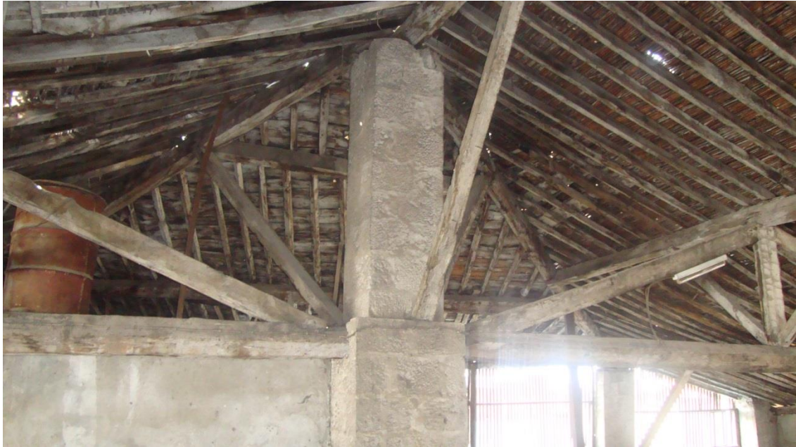
Figure 4.50. The wooden hipped roof on the west part
