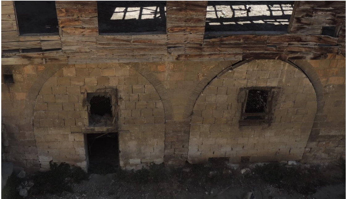
Figure 5.72. The depressed pointed arches on the courtyard facade on the ground floor in Sayınlı Soap Factory, Nizip
