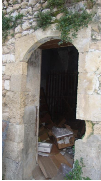
Figure 5.79. The depressed arched door opening with cut stone casing of the office in Aselci Soap Factory Soap Factory, Antakya
