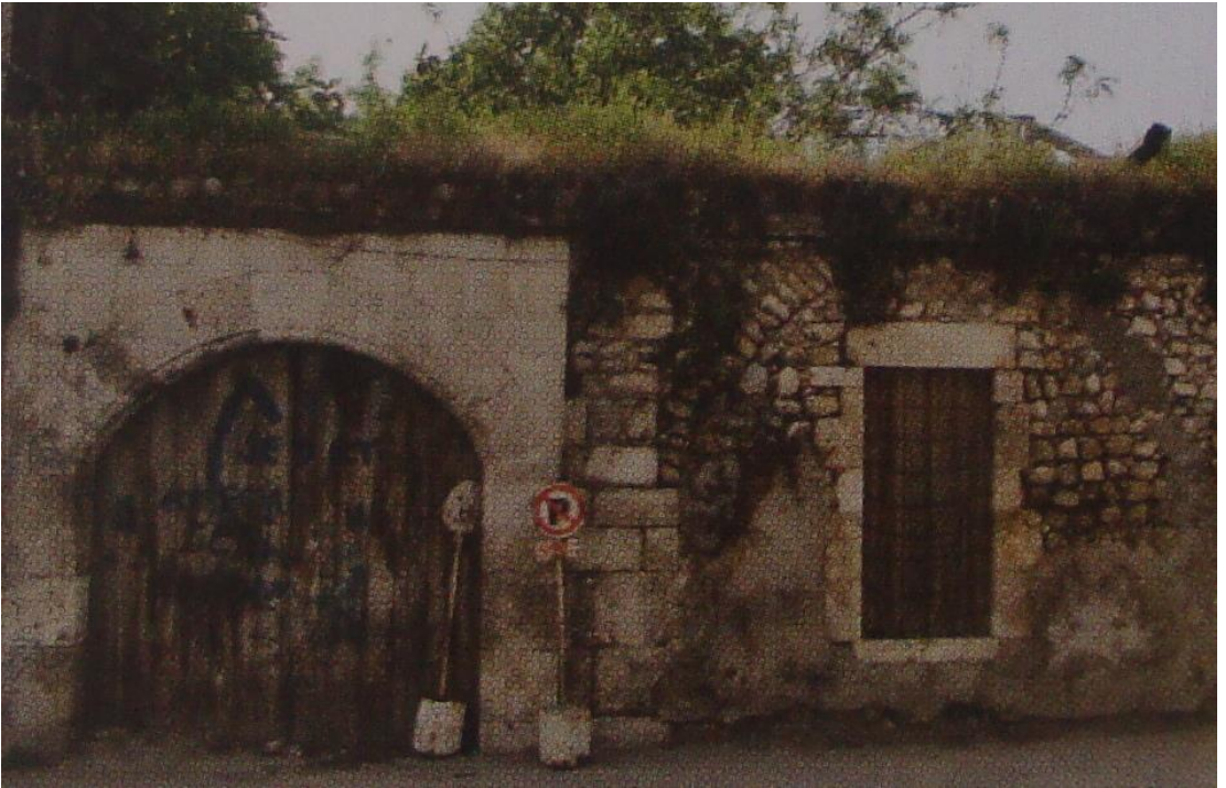
Figure 5.11. The double winged wooden entrance door in stone casing and depressed arched door opening of Aselci Soap Factory, Antakya
