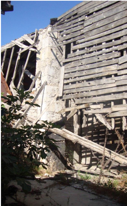
Figure 4.141. The missing part of the roof on the west part of the building
