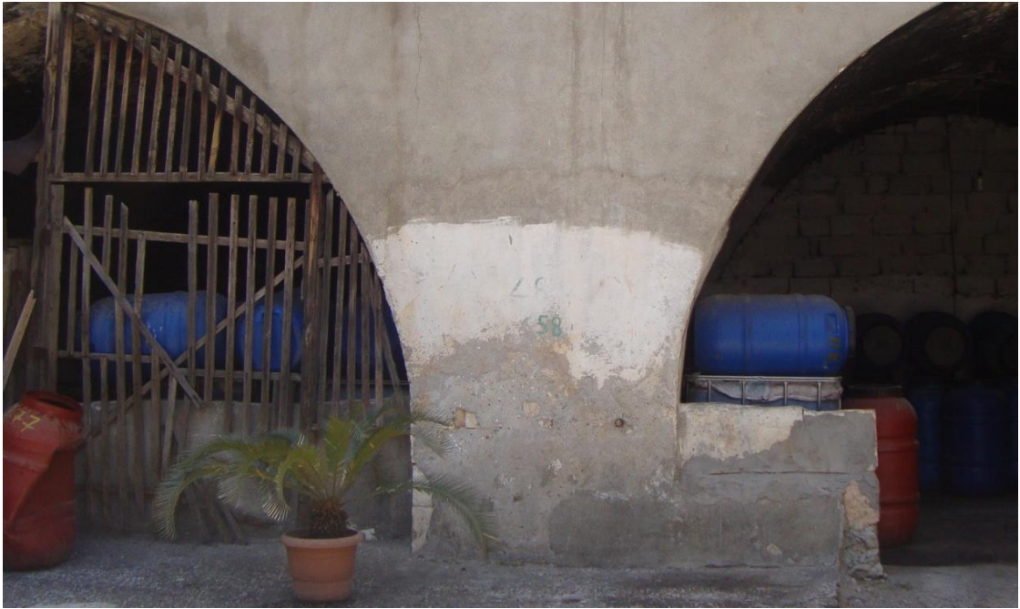
Figure 5.62. The cut stone masonry pier in Kuseyri Soap Factory, Antakya
