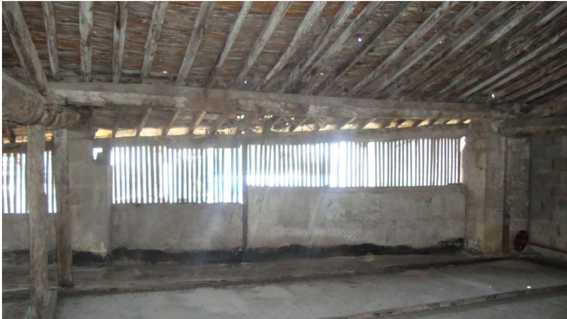
Figure 4.137. The later added low partition brick masonry wall in front of the original wooden screen on the adjacent facade of the spreading area
