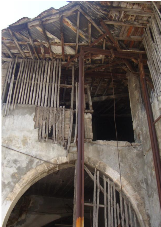
Figure 4.78. Partially missing wooden screen on the first floor on the projected part of the facade
