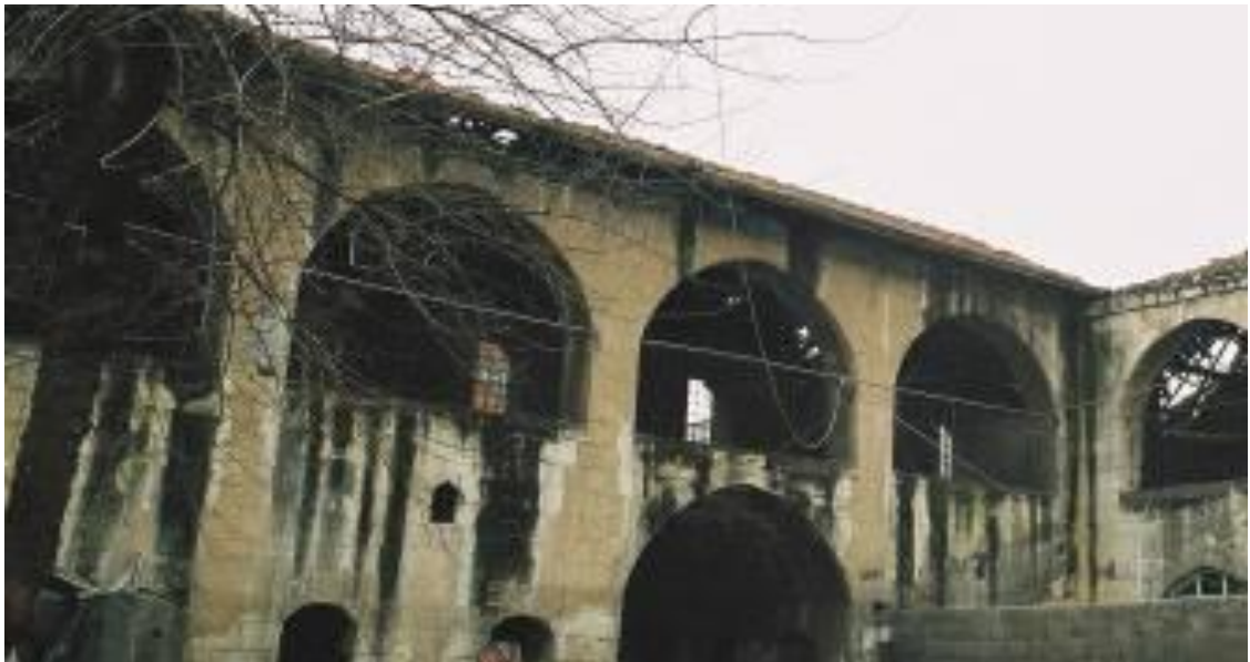
Figure 5.63. The cut stone masonry piers on the courtyard facade of the spreading area in Fincancıoğlu Soap Factory, Nizip
