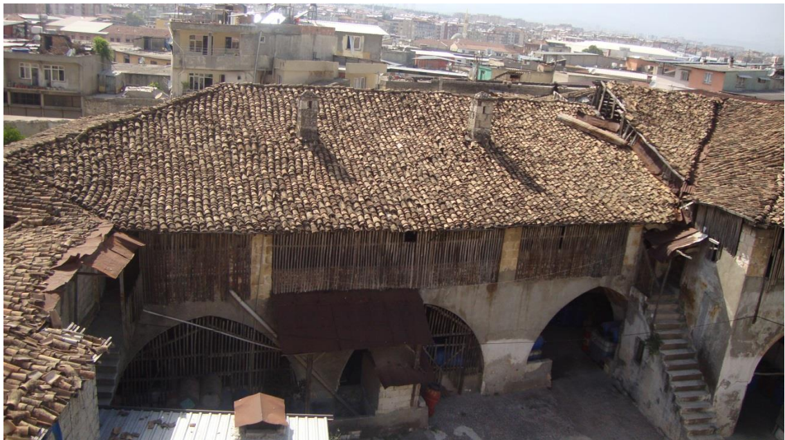
Figure 4.105. View of the hipped roof covered with over and under tiles
