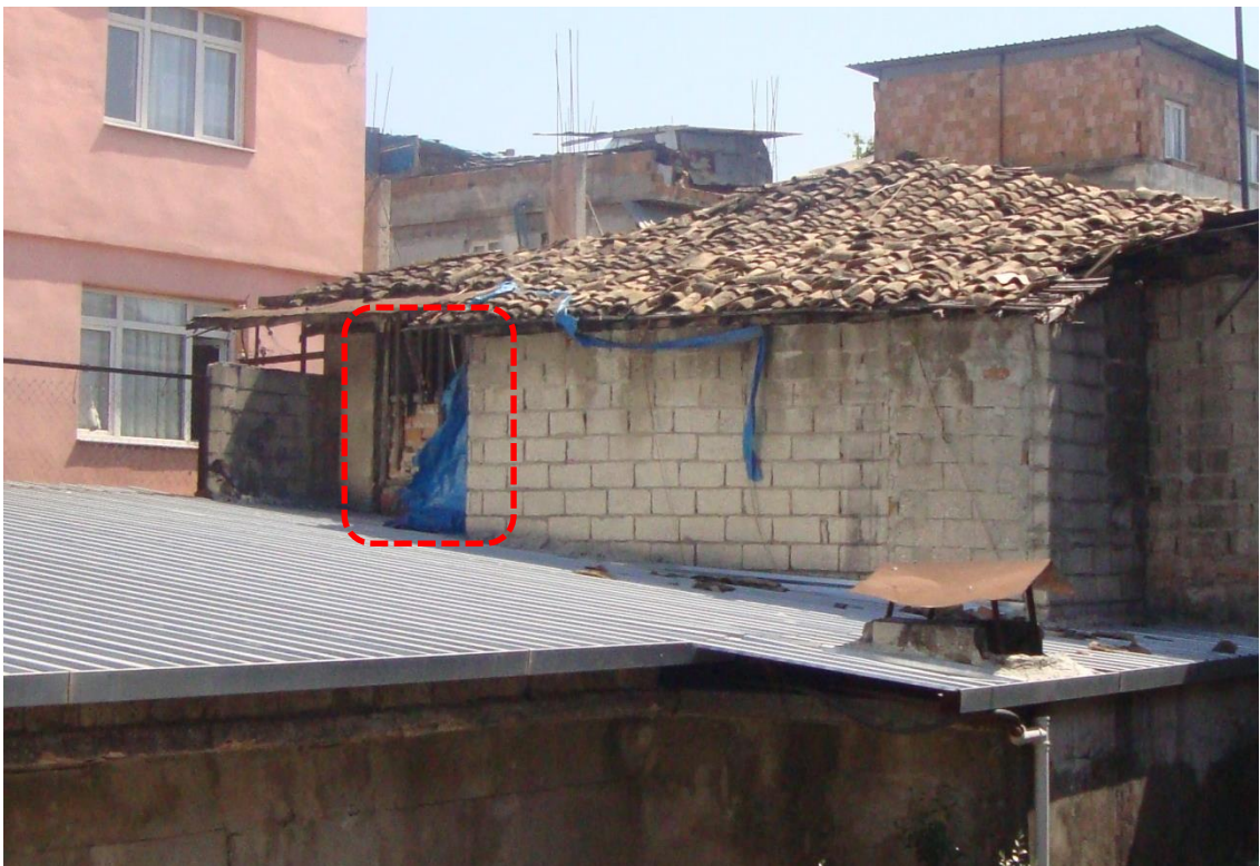
Figure 4.84. The original cut stone stone masonry columns and a part of the wooden screen on the east of the facade
