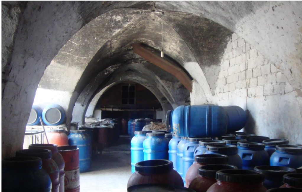
Figure 4.104. The cross vaults on the galleries on the ground floor
