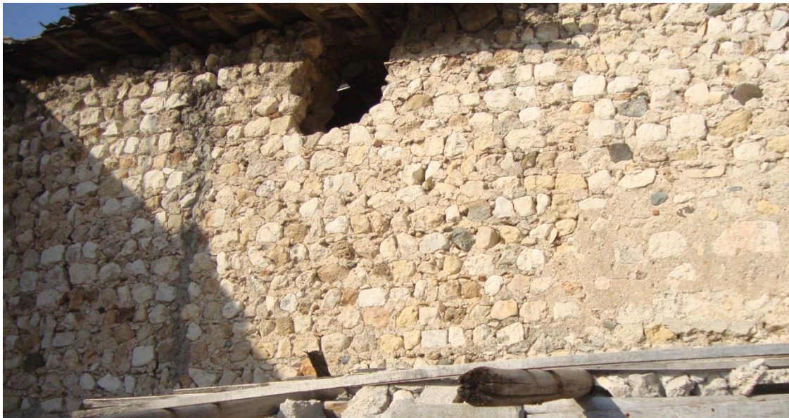
Figure 4.147. Granular disintegration on the stone wall on the west part of the building
