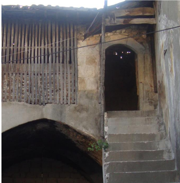
Figure 4.36. The original depressed arched door opening
