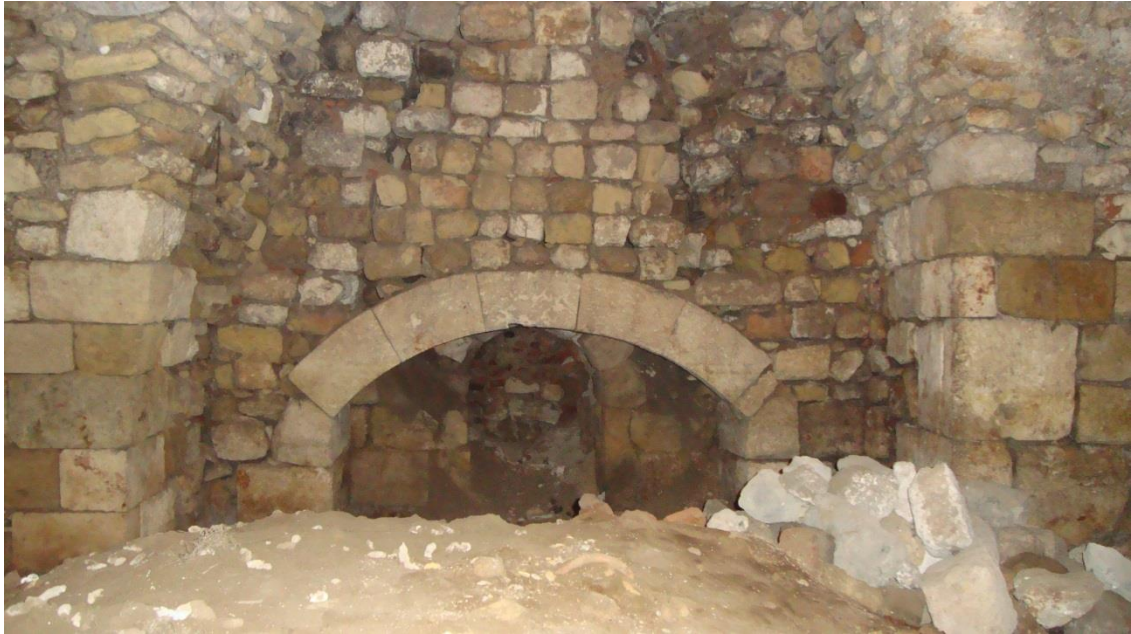
Figure 4.33. Depressed arched fireplace located on the northern wall of the fireplace room
