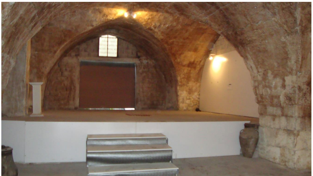
Figure 5.107. View of the stone cauldron covered with plywood in the gallery on the ground floor in Selahattin Ökten Soap Factory, Antakya
