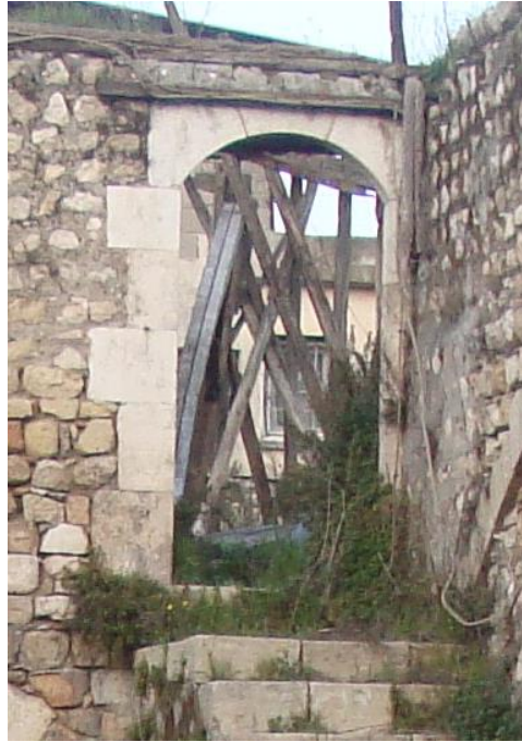
Figure 5.80. The depressed arched door opening of the spreading and drying area with stone casing on the courtyard facade in Aselci Soap Factory, Antakya
