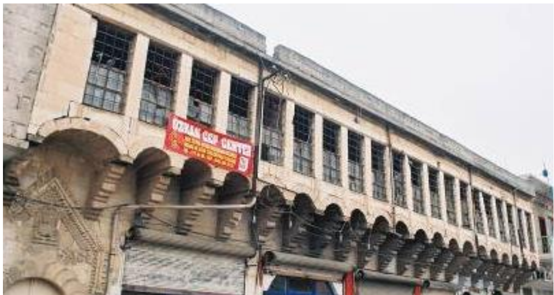
Figure 5.95. The vertical rectangular window openings with grilled iron bars on the street facade on the first floor in Sayınlar Soap Factory, Nizip
