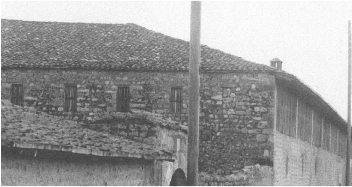
Figure 5.38. The vertical rectangular windows on the stone masonry wall on the adjacent facade of the spreading and drying area in Şeyhoğlu Soap Factory, Antakya
