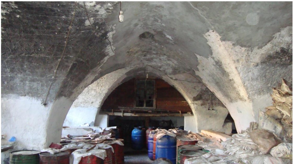
Figure 5.76. The cross vault on the ground floor in Kuseyri Soap Factory, Antakya
