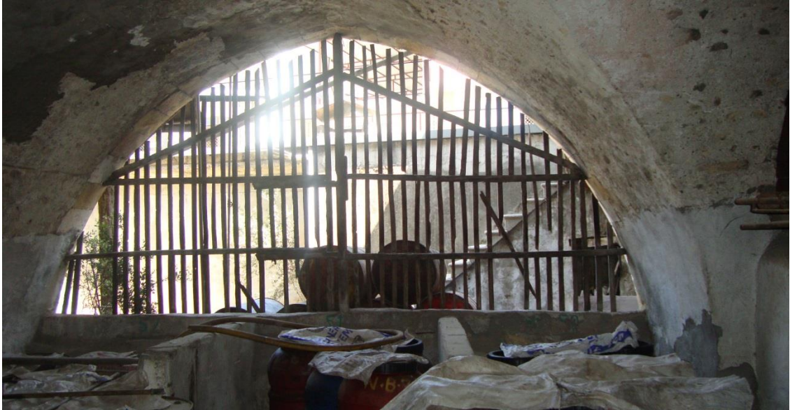
Figure 4.21. The wooden screen on the courtyard facade of I shaped semi-open gallery
