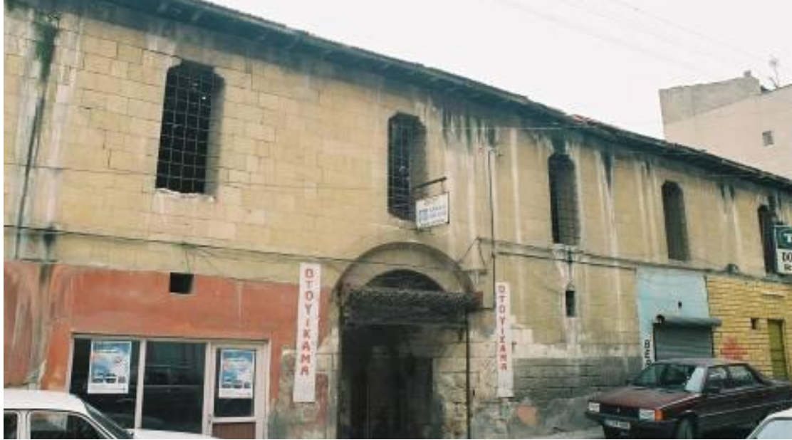
Figure 5.94. The vertical rectangular shouldered arched window openings with grilled iron bars on the street facade on the first floor in Fincancıoğlu Soap Factory, Nizip
