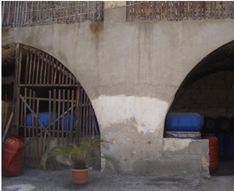
Figure 4.101. The cut stone masonry piers covered with cement plaster
