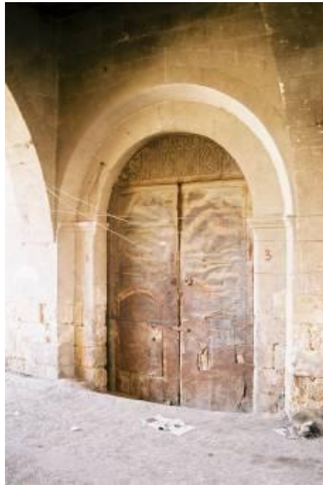
Figure 5.85. The semicircular arched entrance door opening of the semi-open entrance space in Sayınlar Soap Factory, Nizip
