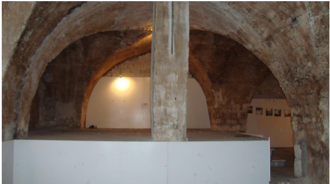
Figure 5.118. The cut stone masonry chimney rising from the fireplace room on the basement floor adjacent to the stone cauldron on the ground floor in Selahattin Ökten Soap Factory, Antakya
