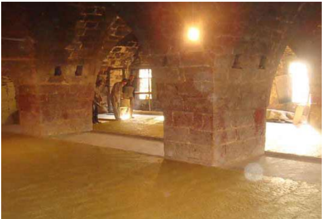
Figure 5.65. The cut stone masonry piers on the spreading area on the first floor in Sadık Adra Soap Factory, Tripoli
