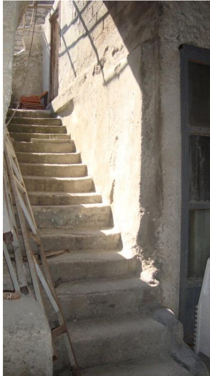
Figure 4.59. The later arranged half-space landing reinforced concrete stair on the west of the distribution space
