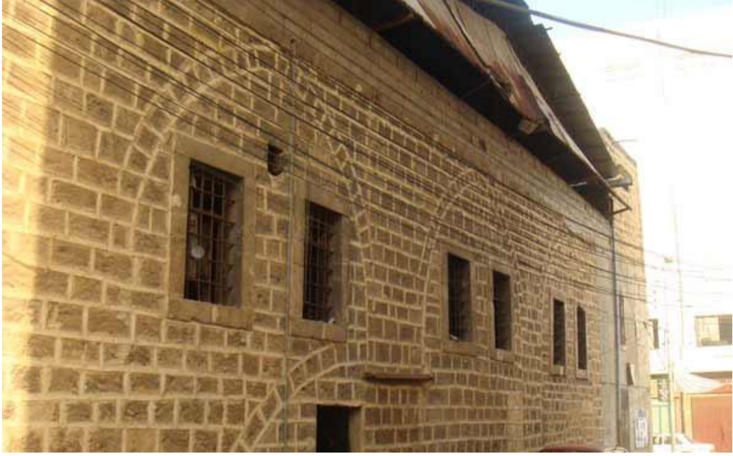
Figure 5.43. The depressed pointed blind arches on the street facade of the spreading and drying area in Sadık Adra Soap Factory, Tripoli
