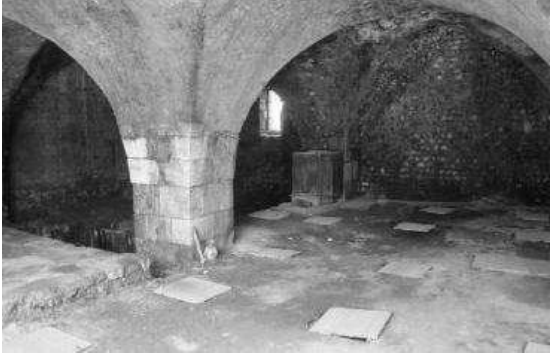
Figure 5.114. The wooden shutters of the original circular olive oil wells buried beneath the ground of the semi-open gallery adjacent to the stone cauldron and causticizing pits on the ground floor in Aselci Soap factory, Antakya (Source: Rifaioğlu, 2014)
