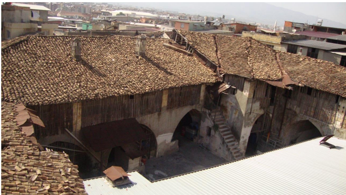
Figure 4.51. The wooden hipped roof covered with over and under tiles
