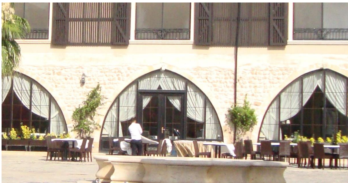
Figure 5.70. The depressed pointe arches on the courtyard facade on the ground floor in Şeyhoğlu Soap Factory, Antakya
