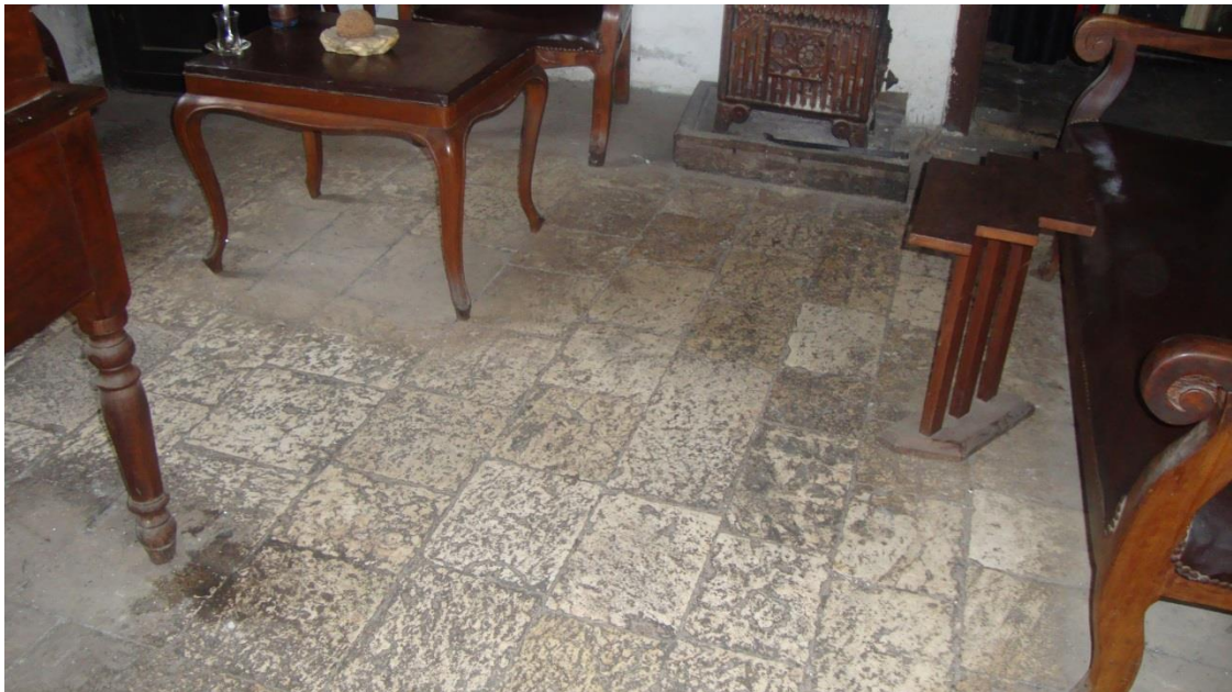
Figure 4.107. The original stone floor covering of the office
