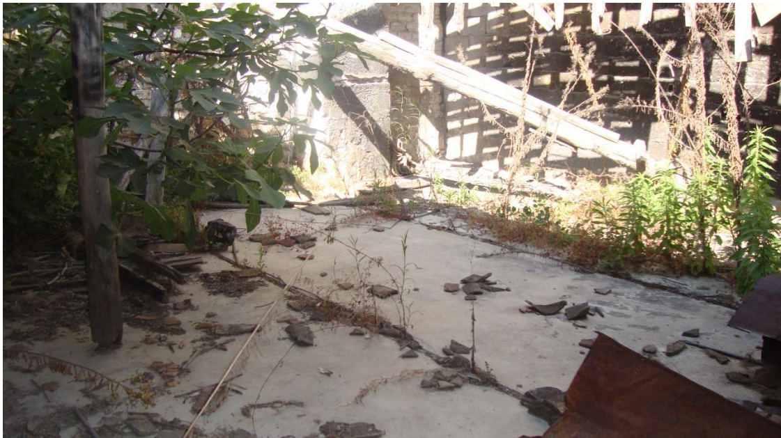
Figure 4.154. Colonization by higher plants on the first floor on the west part of the building
