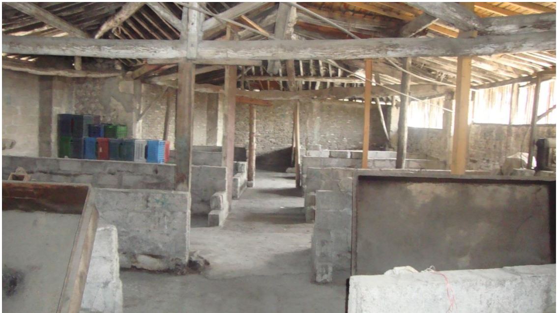
Figure 4.41. Later added low partition cinder blok walls on the drying area
