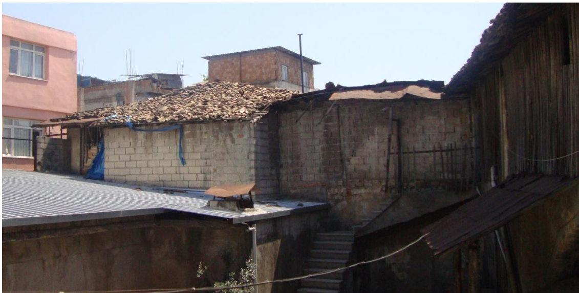
Figure 4.49. The later added cinder block masonry wall of the unoccupied space on the south of the courtyard
