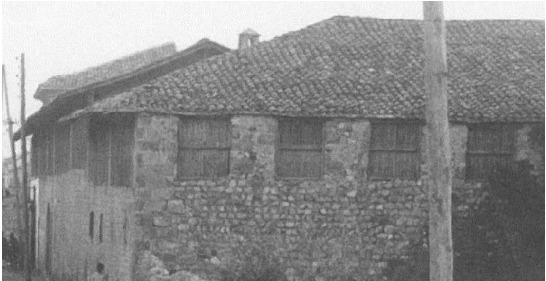
Figure 5.98. The wooden screen on the street and adjacent facades of the spreading and drying area in Aselci Soap Factory, Antakya
