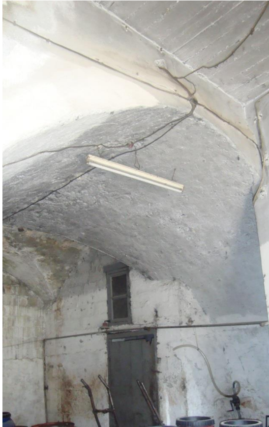
Figure 4.132. The converted part of the original cross vault into the reinforced concrete floor on the L shaped semi-open gallery on the ground floor
