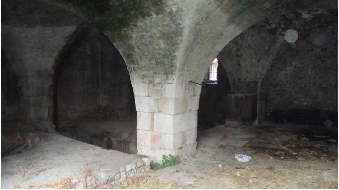
Figure 5.60. The cut stone masonry piers in Aselci Soap Factory, Antakya
