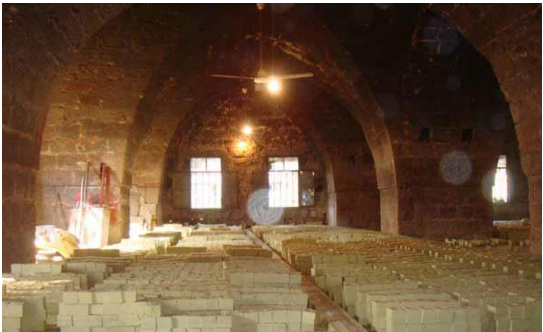
Figure 5.78. The cross vault on the spreading and drying area on the first floor in Sadık Adra Soap Factory, Tripoli
