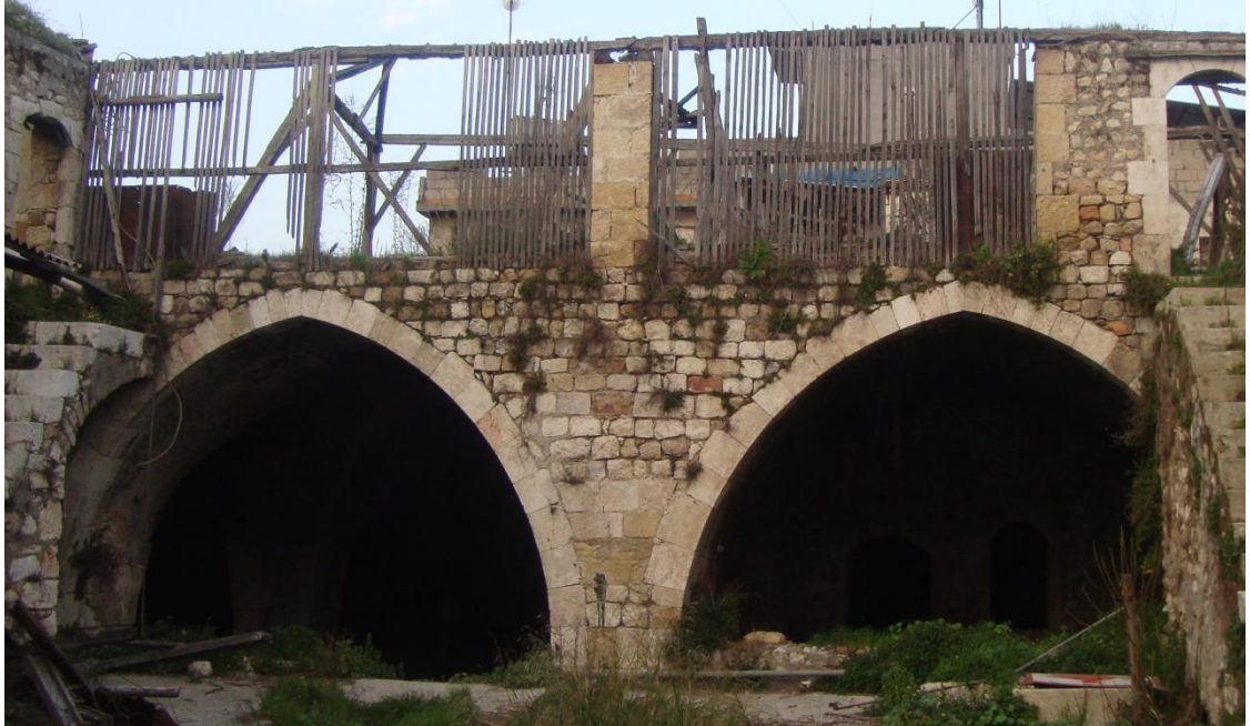
Figure 5.23. The semi-open gallery connected to the courtyard through the depressed pointed arches in Aselci Soap Factory, Antakya
