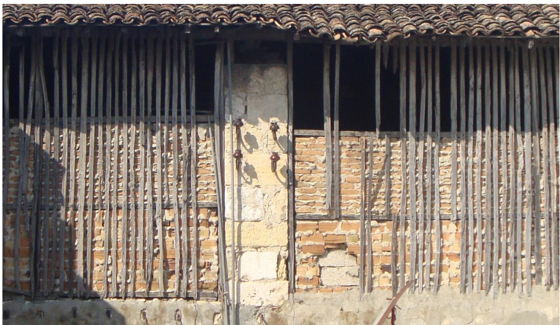
Figure 4.148. Crumbling on the cut stone masonry column on the northern courtyard facade
