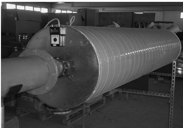
Fig. 3. Single circular duct test system.
