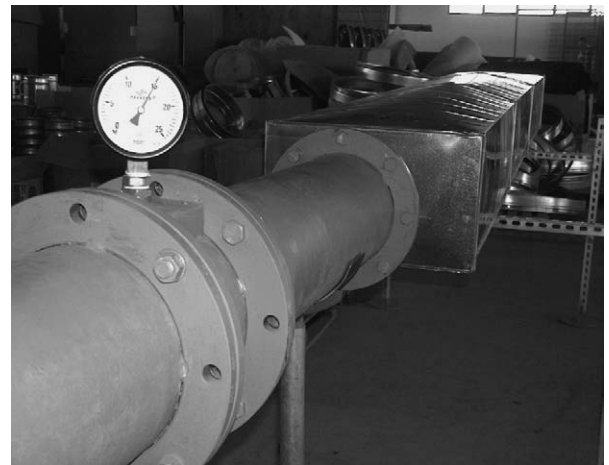
Fig. 4. Rectangular duct test system.
