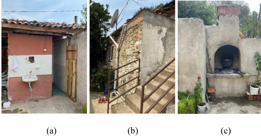
Figure 56: (a) The toilet, (b) the mass addition and (c) the fireplace (Photos taken by Author 2022)
