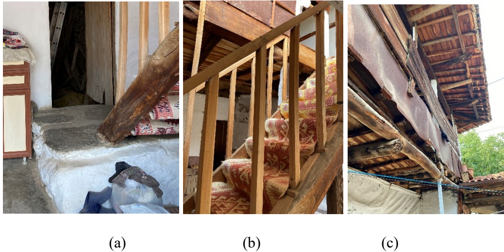
Figure 93. (a) Stepping stone, (b) timber stair and (c) hayat in the case 1 (Photos taken by Author 2022)
