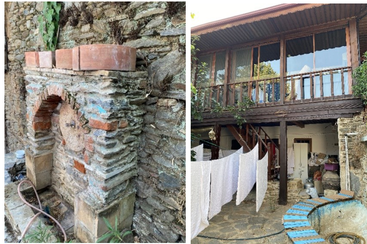
Figure 87. The contemporary fountain (left) and pool (right) in the case 4 (Photos are taken by Author 2022)
