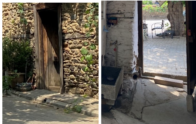
Figure 96. Drainage in the case 3 (Photos taken by Author 2022)
