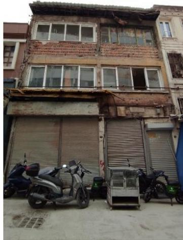
Figure 5.20. An example of a building with floor height incompatible with the conservation development plan, Block 187, Lot 58
