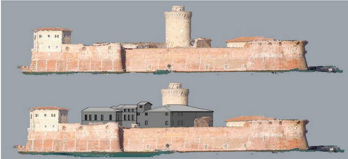
Figure 2. 19. Virtual 3D model with and without the Palazzo di Cosimo reconstruction. - An example of integration of geometry-based modelling technique with IBM technique (Source: Caroti et al. 2021)
