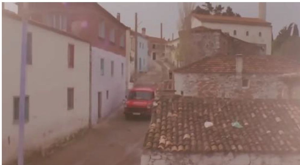
Figure 4. 38. The comparative approach provides a view of 12098 Street in terms of reliability degree (Source: Author 2024; Yılmaz 1985)
