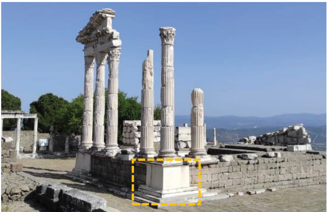
Figure 2. 7. Example of Anastylosis (yellow framework) and Partial Reconstruction in Pergamon Acropolis which is a UNESCO World Heritage Site (Source: Author 2022)
