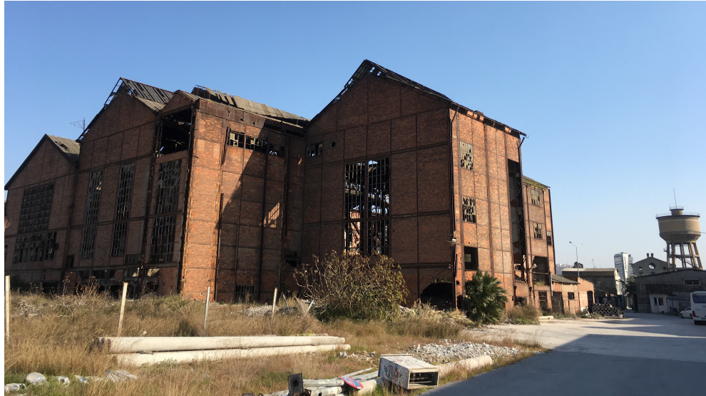
Figure 31. Alsancak Electricity Factory (Author, 2022)
