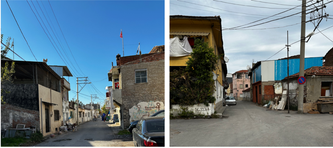
Figure 32. The View of Streets in the Backside of Port (Author, 2024)
