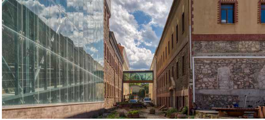
Figure 33. Flour Plant I (Source: İZKA 2021)
