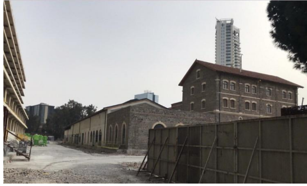
Figure 87. Building 3 (Source: Author 2022)
