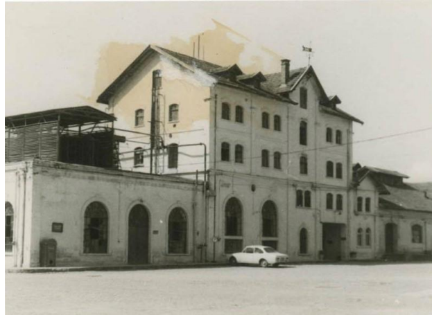
Figure 86. An old photo of 2, 3 and 4 numbered buildings.
