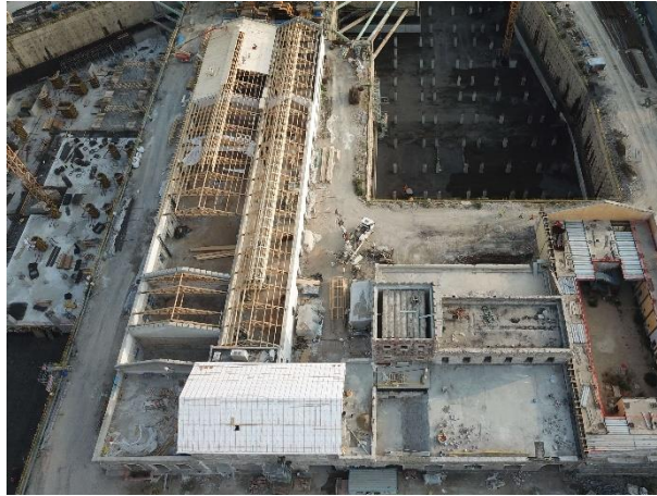
Figure 91. Roof system of Building 5 during the restoration process (Source: Grid İnşaat)
