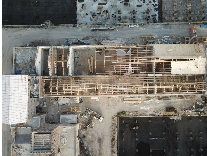
Figure 81. Roof system of Building 1 and 2 (Source: Grid İnşaat)
