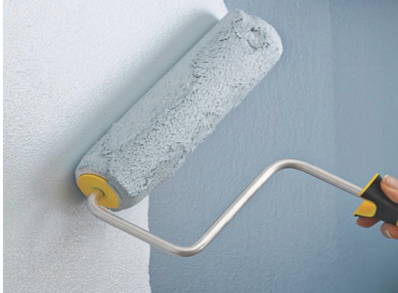
Figure 2.8. Roller Application of Painting
