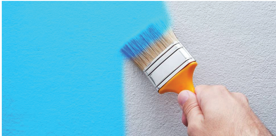
Figure 2.7. Brushing Application of Paint
