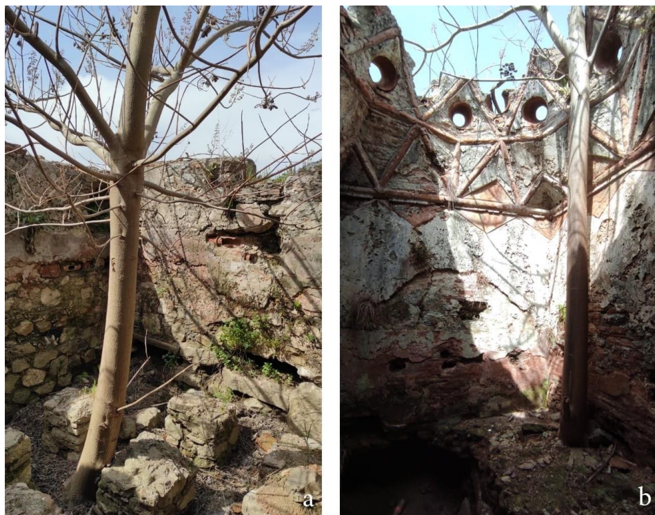
Figure 3. 14. Photos from Yahşi Bey Bath: East Halvet – Plant growth (a), Weast Halvet – Microbiological colonization (b)
