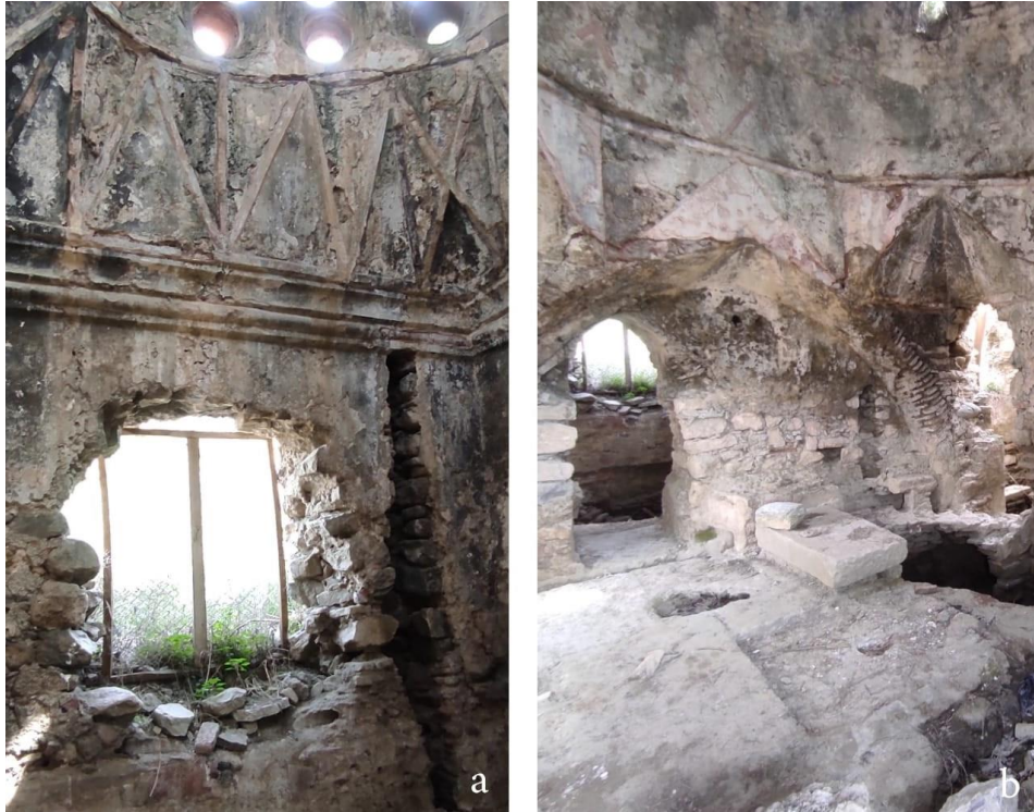
Figure 3. 13. Photos from Yahşi Bey Bath: Soyunmalık – Discoloration (a), Ilıklık – Vandalism (b)
