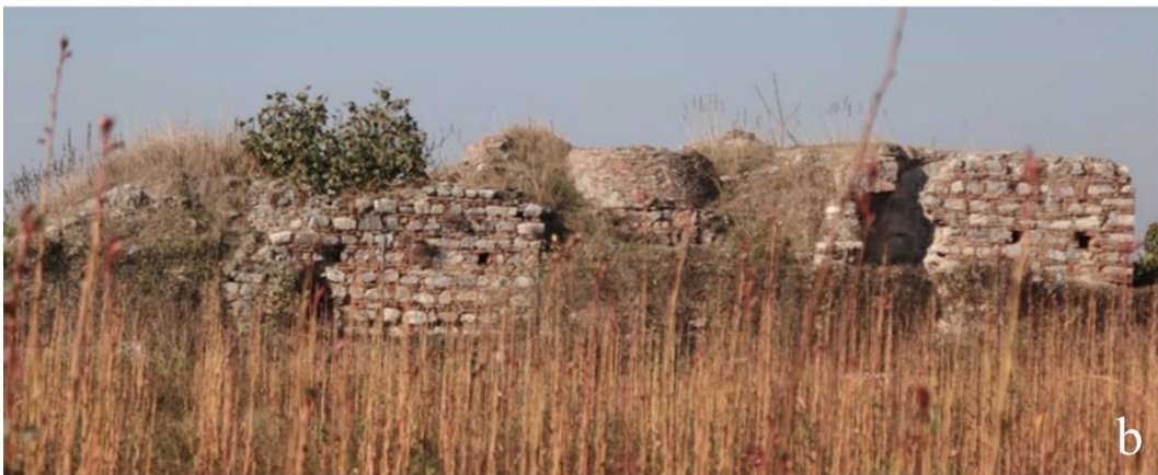
Figure 3. 9. Plan of Kale Altı Bath (Daş 1997), North-East view (a), East view (b)
