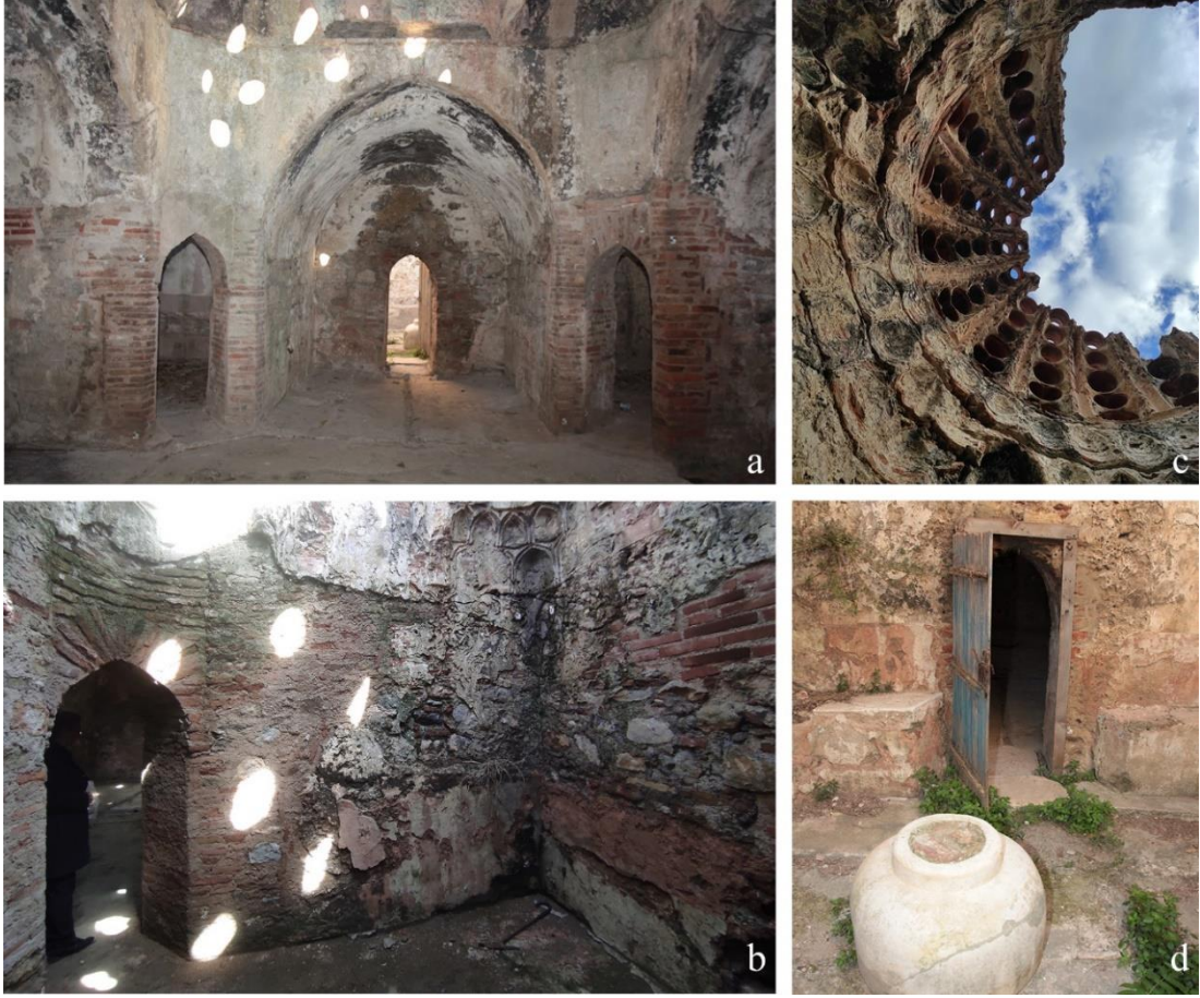
Figure 3. 7. Photos from İsa bey bath; General view from Sıcaklık (a), Halvet , (b), The dome of the Ilıklık (c), General view from Ilıklık (d)
