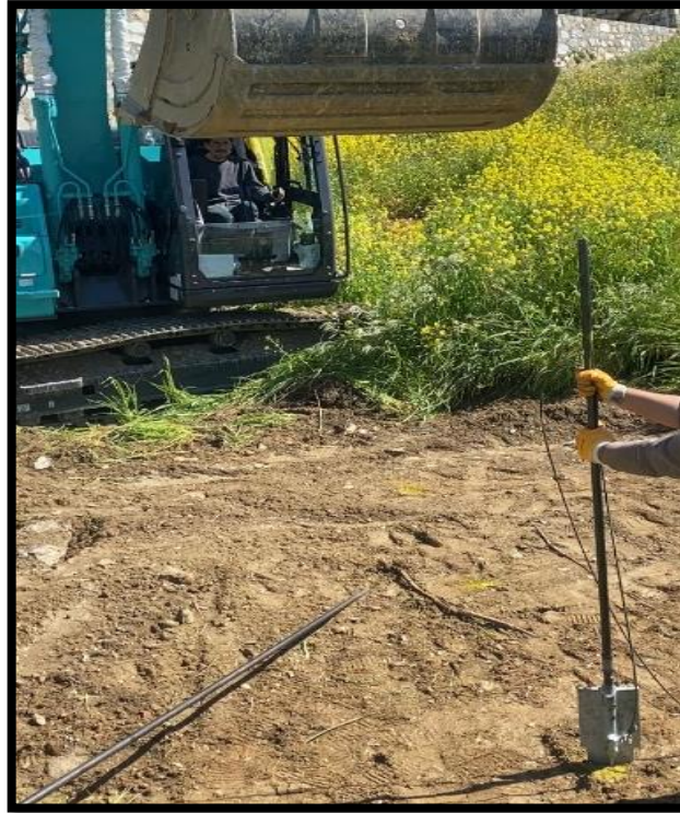
Figure 3.8 The installation of the FPA-I anchor vertically to the soil
