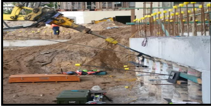
Figure 2.37 Location of flip anchors used to support pile retaining structure (Australia) (Source: Platipus Civil Engineering & Construction Brochure, 2022)
