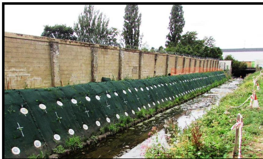
Figure 2.34 Layout of flip anchors used in Salmons Brook River (England)(Source: Anchor System International, 2020)
