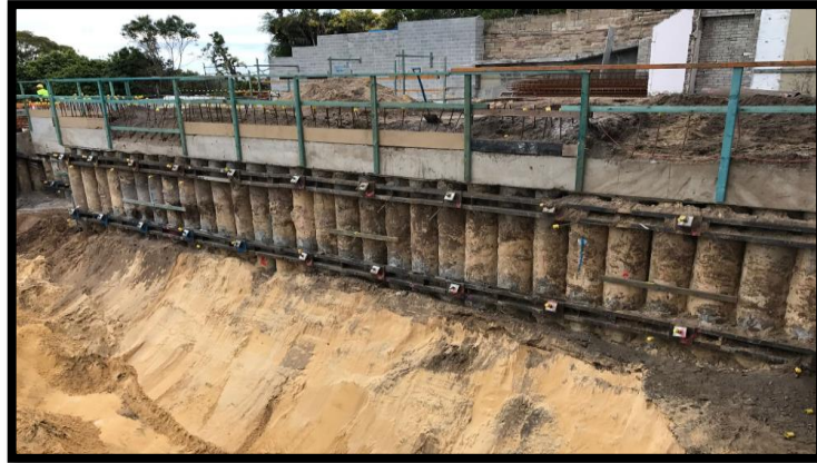
Figure 2.38 Flip anchor systems applied on Cranbrook Road (Australia)(Source:Platipus Civil Engineering & Construction Brochure, 2022)
