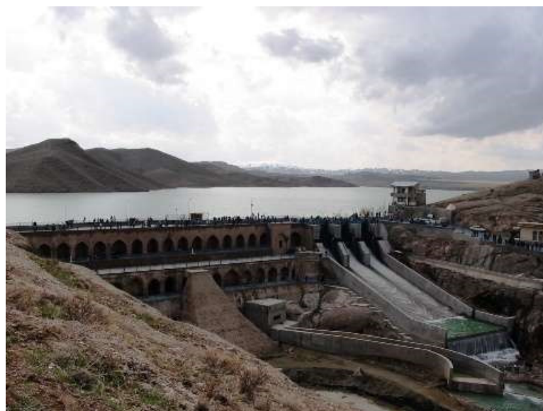
Figure 3. A view of Fariman Dam. An ancient dam possibly dating back to the reigns of the Sassanid kings of Persia (224–710 AD), it was rebuilt during the Timurid and the Qajar eras in its current form (adapted from [9]).
