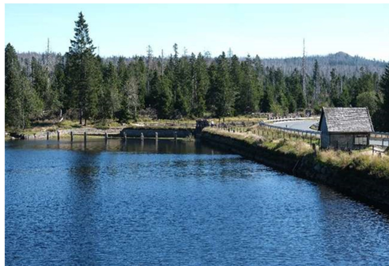
Figure 11. Oderteich Dam (with the permission of J. Dietrich).
