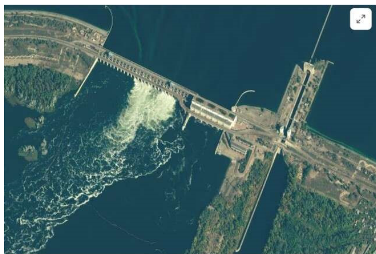
Figure 21. The Nova Kakhovka hydroelectric power dam.
