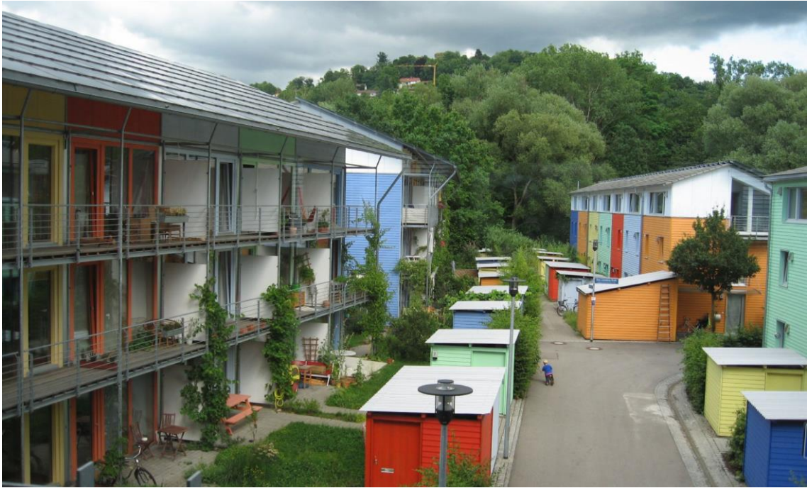
Figure 3.15. Freiburg is a Neighborhood with Solar Panels
