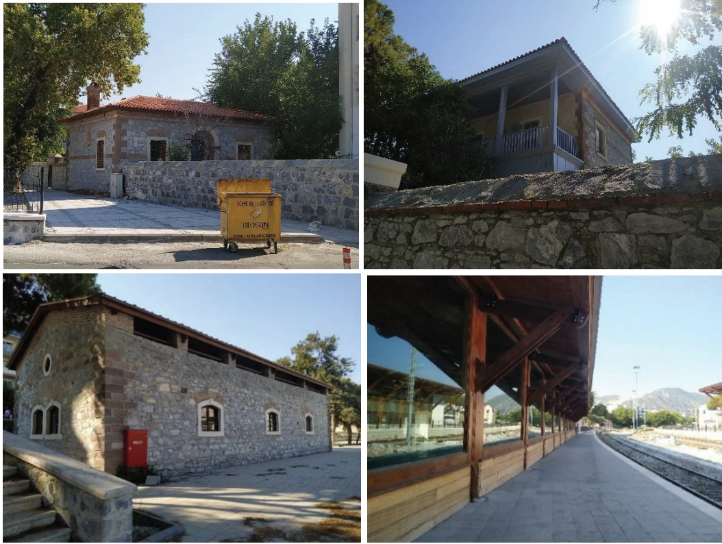
Figure 84. Guest houses of the Söke station and warehouses from Söke station, recently renovated by the author, 2019
