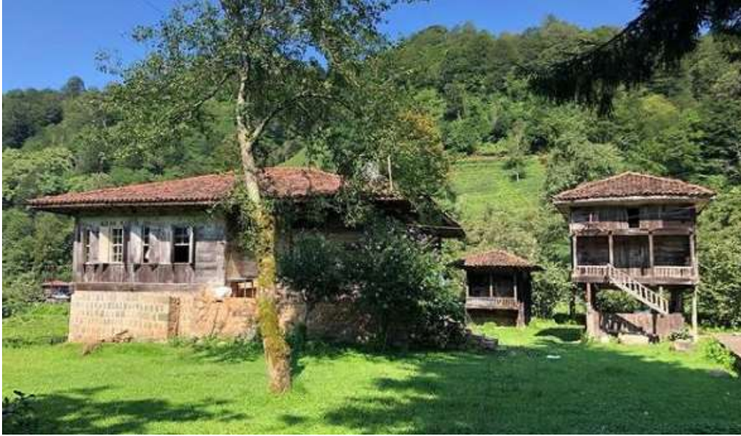
Figure 4.27. Kitapçı House (1771) with its Bağu and Nayla , Hara Village (Source: Yasayan Lazca 2019)
