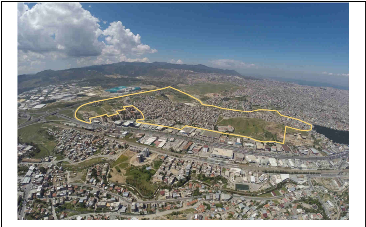
Figure 75: Ariel Photo from East Direction
