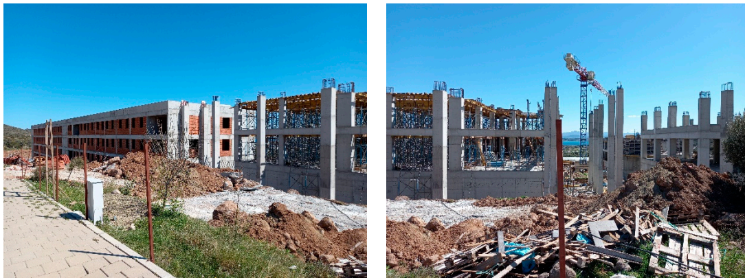
Figure 6. The construction site of the new dormitory.
