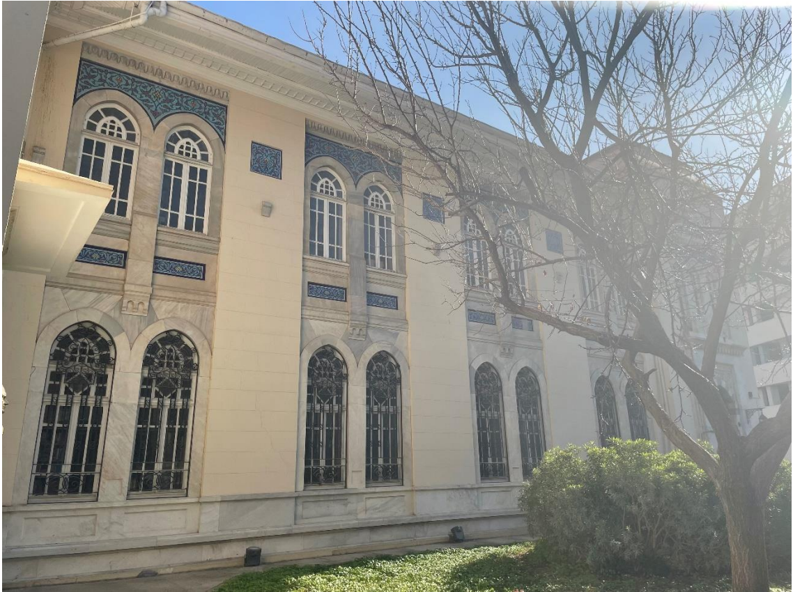
Figure 3. 4 Exterior view of the library (Source: Umut Özsvaşıcı, 2022)
