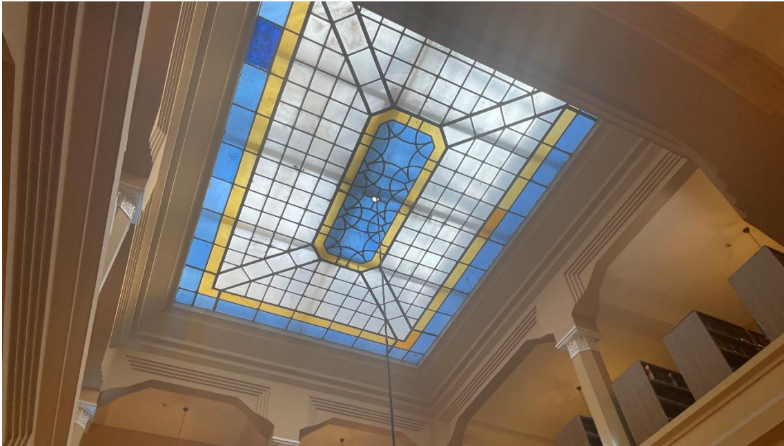
Figure 3. 9 Roof of the building in interior view (Source: Umut Özsavaşcı, 2022)
