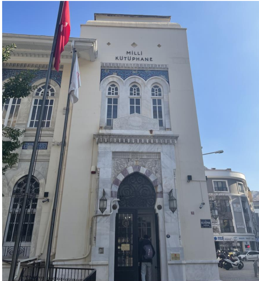
Figure 3. 10 Doors and windows of the library (Source: Umut Özsavaşcı, 2022)
