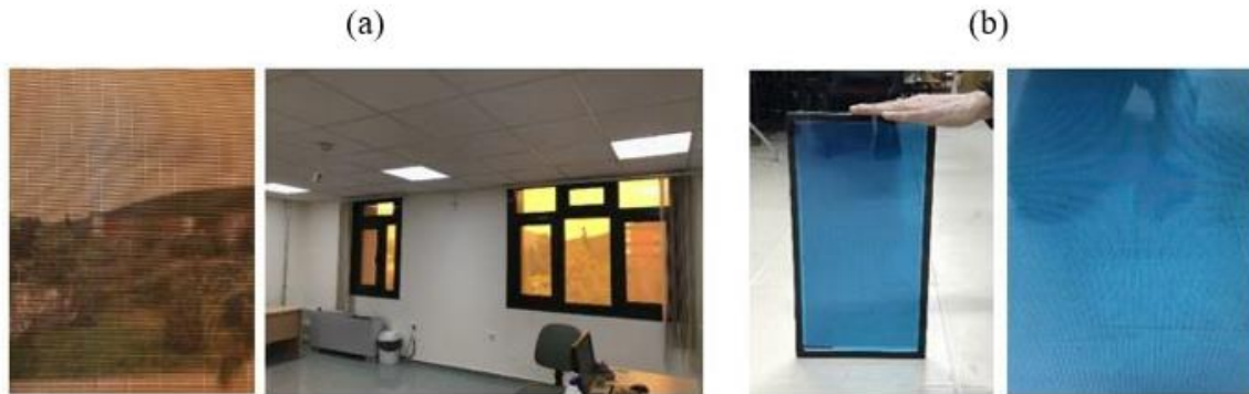
Figure 2.3. (a) Colored (orange) PV glass application in Block E, IZTECH Campus (b) Colored (blue) PV glass application in Block E, IZTECH Campus *Glazing is supplied by OnyxSolar Company © for a Doctoral Thesis supported by TUBITAK.
