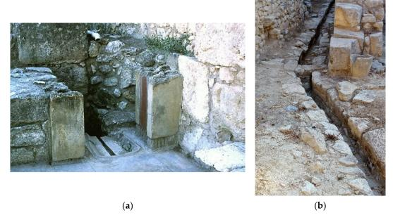
**Figure 3.** Minoan sanitation: (a) A general view of the ground-floor toilet in the residential quarter of the palace of Knossos and (b) part of the Minoan drainage system at the "Little palace" at Knossos (with permission of A. N. Angelakis).
