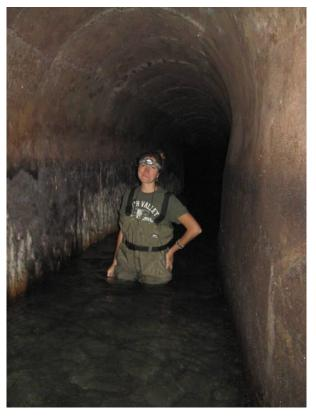
**Figure 11.** The AQUA VIRGO in Rome is a Roman aqueduct that still transports approximately  $1 \text{ m}^3/\text{s}$  ( Photo Cees Passchier) [11].
