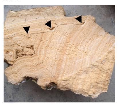
**Figure 12.** Cleaning traces in the aqueduct of Divona, with marks made by a scraping tool (Photo Cees Passchier).
