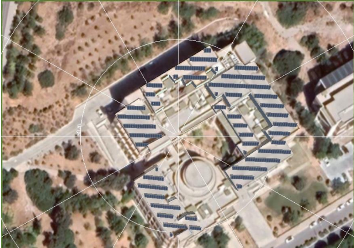
Figure 18. Flat Roof Panel Installation
