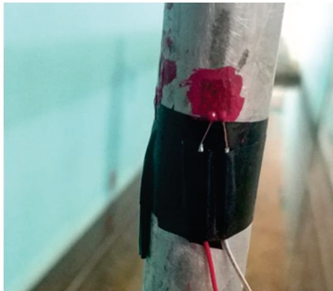
Figure 4.16. Strain gauge sensor on the tower bottom
