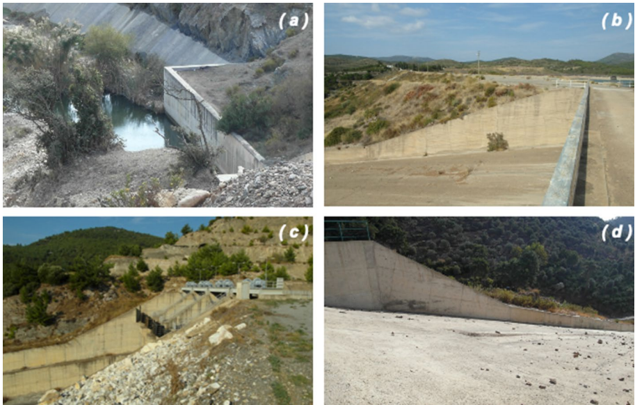
Fig. 29 a Wall on the end of spillway chute of Kavakdere Dam, and side walls of spillways of b Urkmez Dam, c Tahtalı Dam, and d Gumuldur Dam
