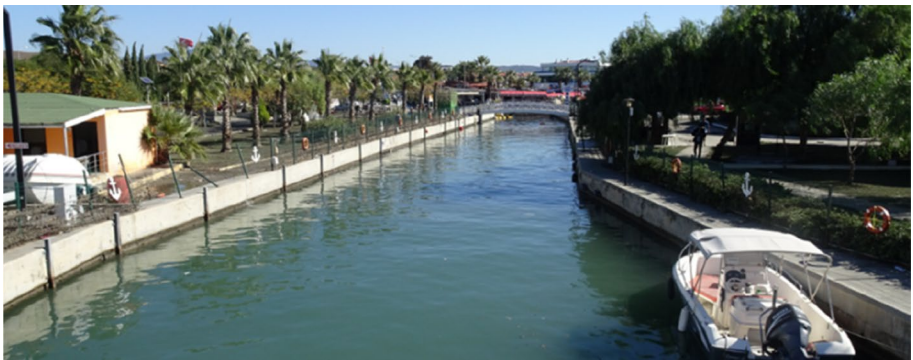
Fig. 30 Sidewalls of the river canal in the Sığacık Marina where no displacements were observed (Photo: Courtesy of Gurel Özdemir). (38°11'33.86"N 26°47'4.07"E 14:16 / 31.10.2020)
