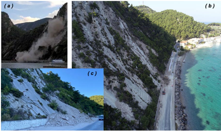
Fig. 21 a Snapshot of Avlakia rockslide from a video recorded during the failure (source: https://www.cnn.gr/ellada/story/240726/seimos-samos-vinteo-apo-katolisthisi-sta-aylakia ) b aerial photograph of the slide 2 weeks after the earthquake (courtesy of I.N. Spyrou and Prof. K. Ziopoulou 37°47'48.0" N, 26°51'27.7" E), and c a closer view of the rockslide illustrating the rock formation more clearly (picture by HAEE/ETAM reconnaissance team)
