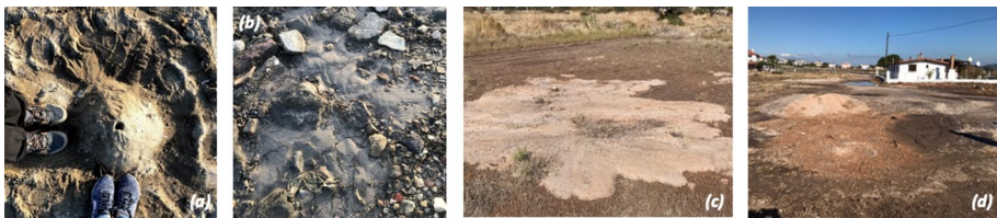
Fig. 7 Surface manifestations of earthquake-induced soil liquefaction in the form of sand boils at shores of Icmeler and Gulbahce district: a 38^{\circ}20'18.4'' N 26^{\circ}38'51.0'' E, b 38^{\circ}18'37.3'' N 26^{\circ}40'47.1'' E, and c-d 38.338088 N, 26.647763 E
