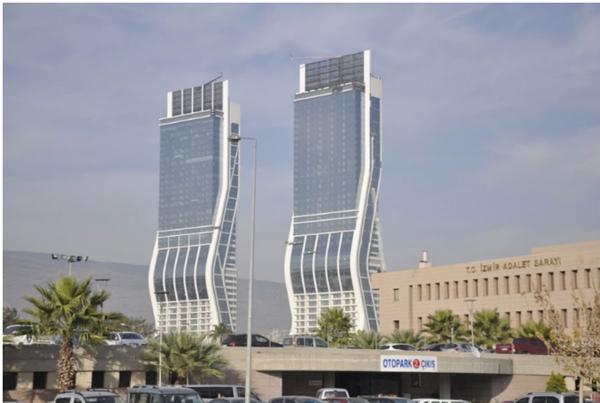
Fig. 3 200 m high Twin Folkart Towers in Bayrakli supported on a piled raft system. No earthquake-induced damage was identified or reported for such foundation systems
