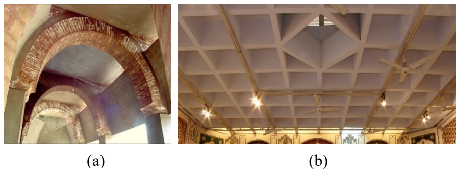
Figure 4.60. brick arch supporting RCC slab (a) waffle slab of multipurpose hall (b) (Source (a &b): Kamil Khan Mumtaz Official Facebook page,2021)
