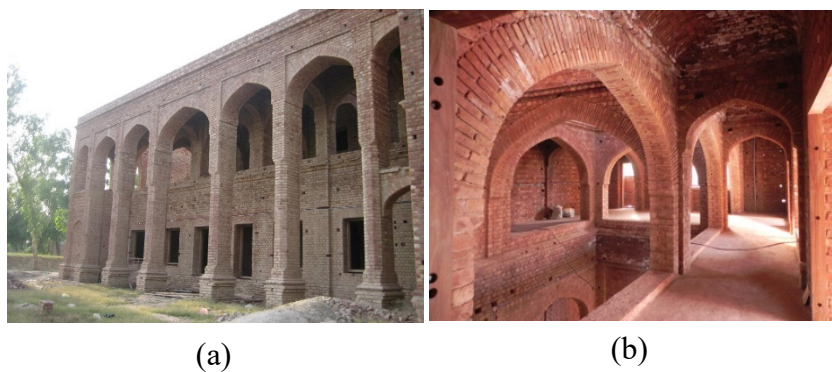
Figure 4.27. Red brick used as construction media (a) red brick used as finishing media (b) brick vaults (Source: Kamil Khan Mumtaz official Facebook page, 2012)
