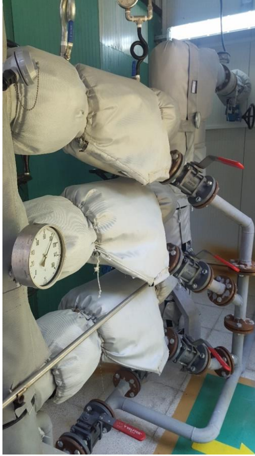
Figure 18. Picture of the test setup with aerogel blankets in B4A well.
