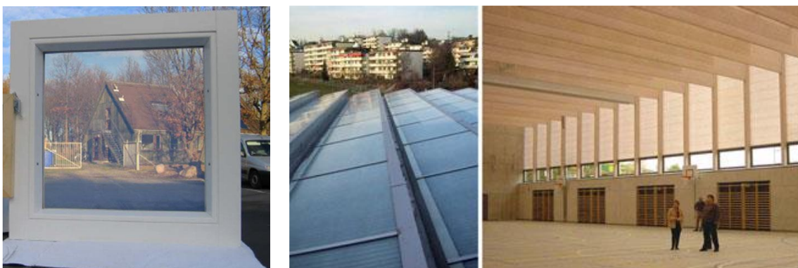
Figure 14. Examples of super insulating silica aerogels window and aerogel granulate filled glass fiber composite panels in the form of a transparent day lighting roof construction [22].
