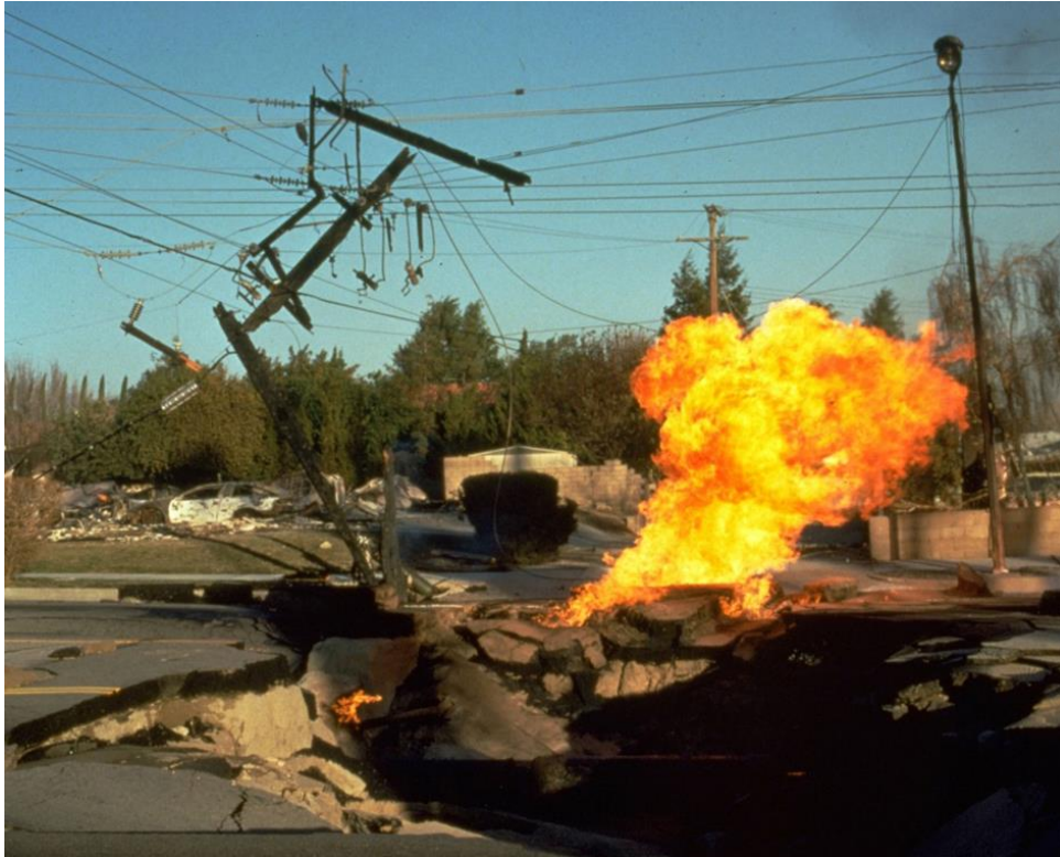
Figure 2.5. A fire ruptured by failed gas pipeline in the city center of Granada Hills The during Northridge Earthquake, 1994 ( M_w=6.7 ) (Jeon and O'Rourke, 2005).
