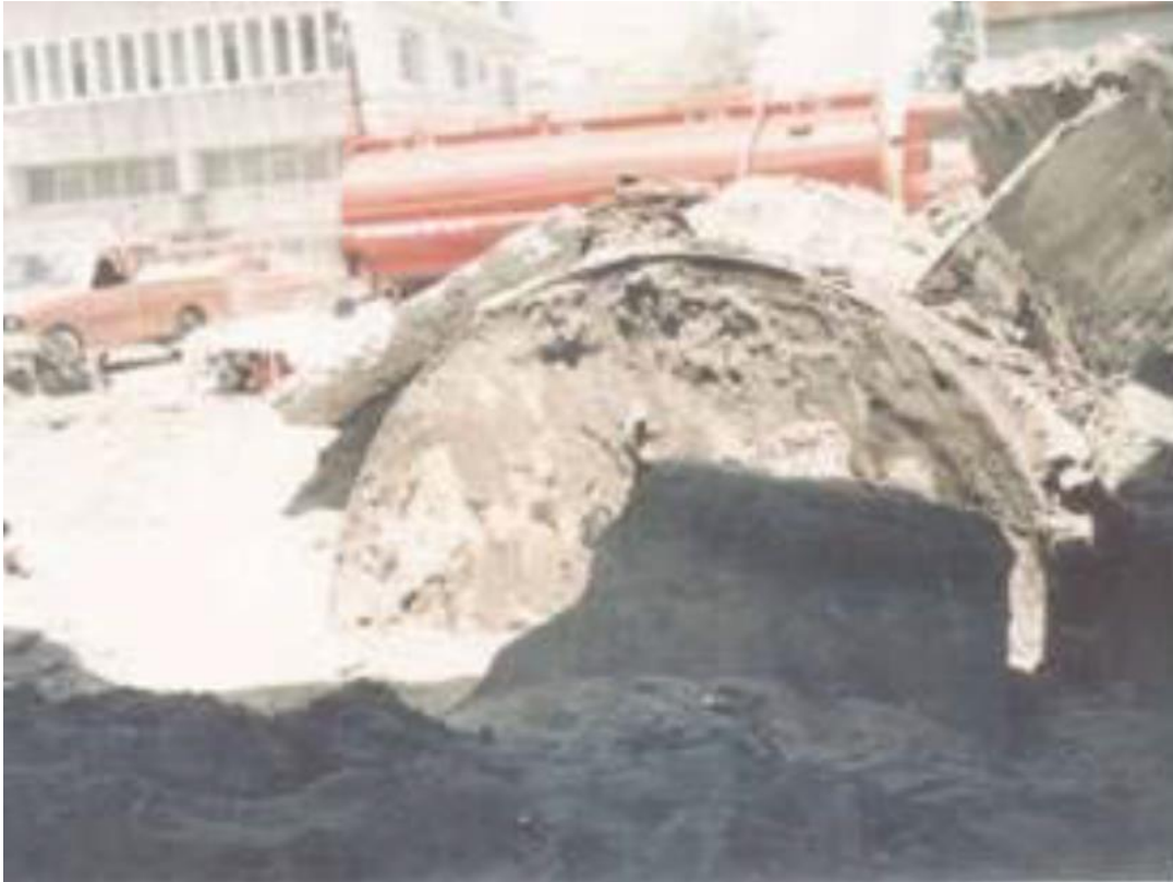
Figure 2.6. Uplifting of gasoline tank during Luzon Earthquake, 1990 ( M_w=7.7 ) (Orense et al., 2011)
