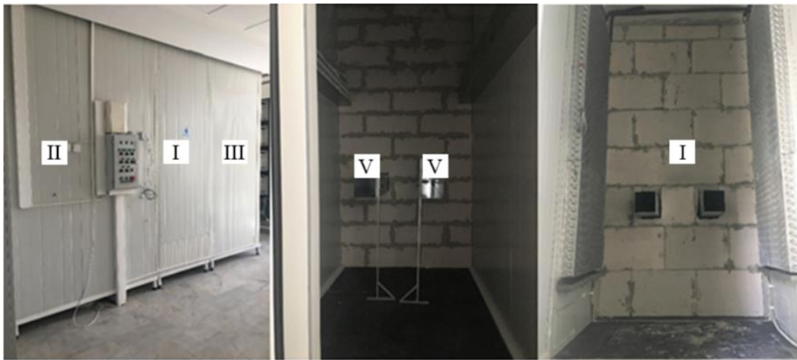
Figure 3.3. I: aerated concrete wall, II: indoor environment, III: outdoor environment, V: air ducts
