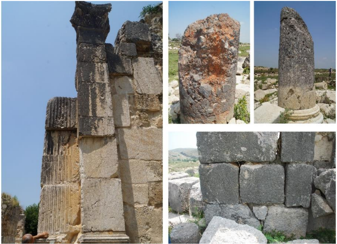
Figure 11. Deterioration on limestones in the forms of black crust, yellow patina, loss of cohesion, biological colonization, cracks.
