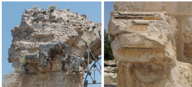
Figure 18. Crumbling and erosion observed on stone surfaces.
