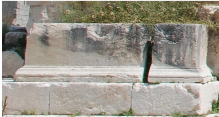
Figure 14. Soiling on the excavated and black crust on the standing parts of stone surfaces.
