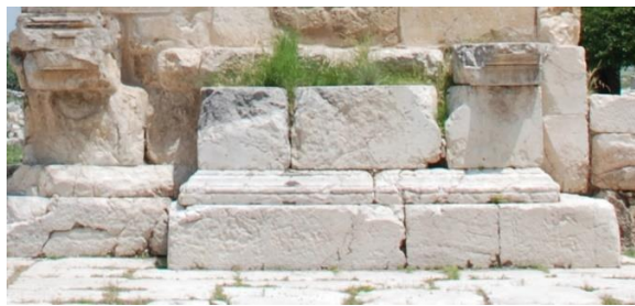
Figure 17. Scaling and hair cracks observed on stone surfaces.
