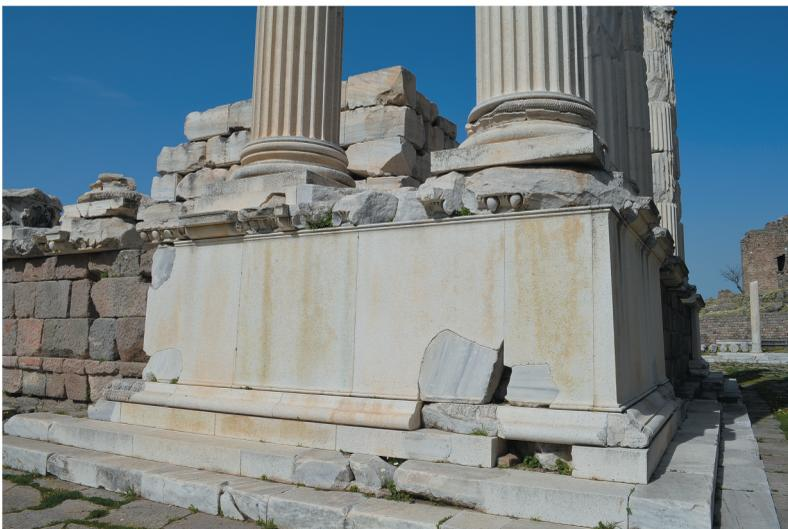
**Figure 18.** New concrete parts with original pieces, Pergamon.
