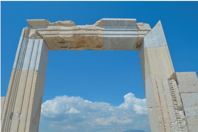
**Figure 23.** Completions of the door with different materials as marble and reinforced concrete at Laodikeia.
