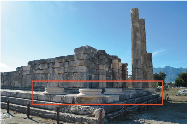
**Figure 7.** New column bases for two-dimensional plan layout, Letoon.
