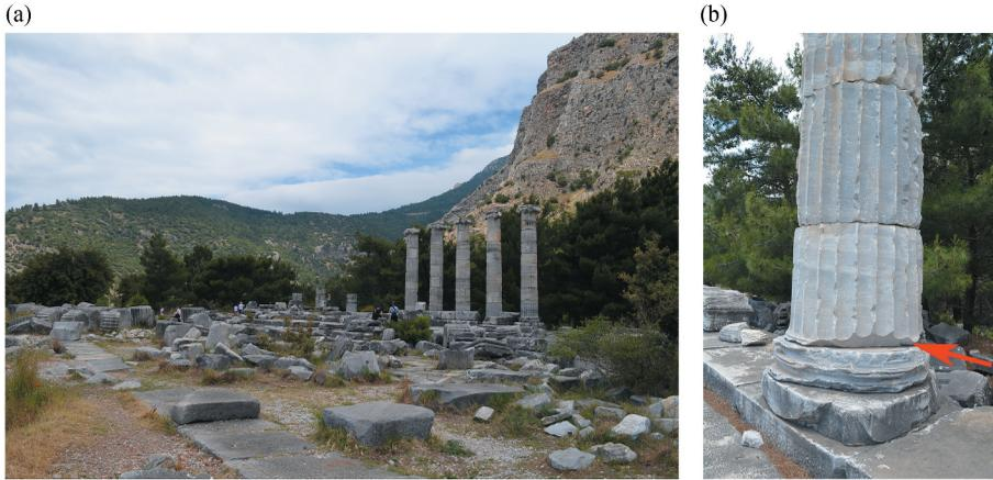
**Figure 5.** Re-erected columns of the Temple of Athena with reduced height in the sanctuary and missing torus, Priene.
