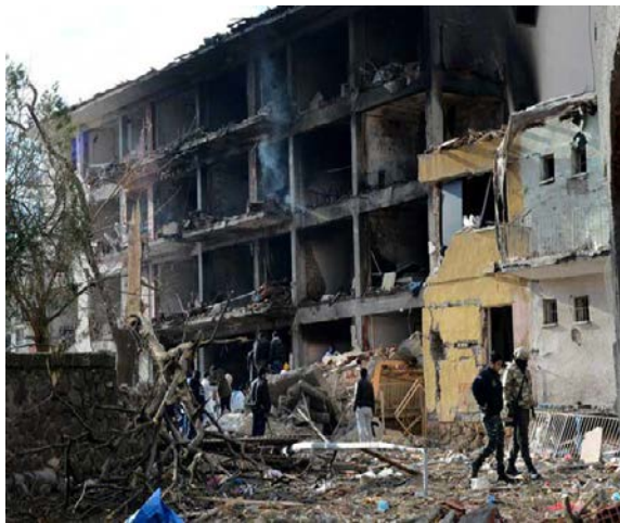
(a) Diyarbakir Cinar District Police Department (14.01.2016)
