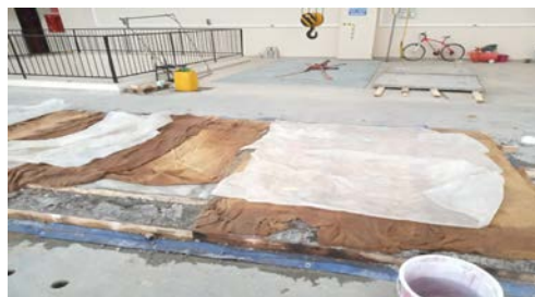
(g) Burlap and plastic for curing
