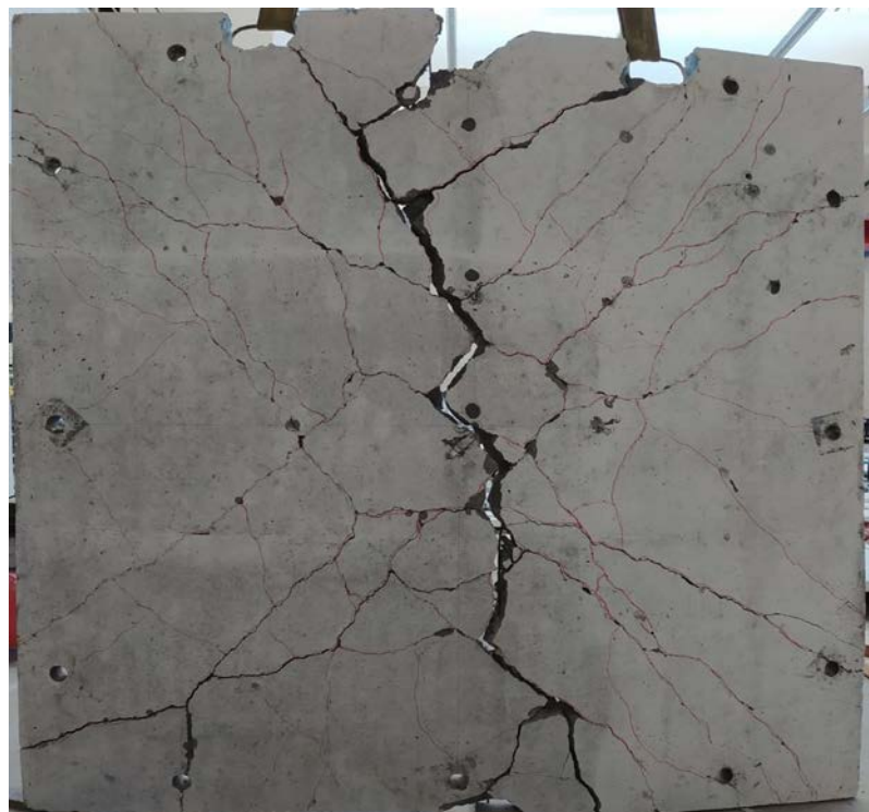
Figure 4.4.24. Rear Face Crack Patterns After Testing for Panel JA-Plain-RF
