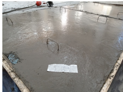
(f) Finishing smooth surface
