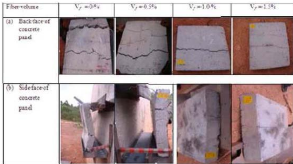
Figure 2.3. Back and Side Face of Panels After Testing With the Varying Volume of Steel Fibers
