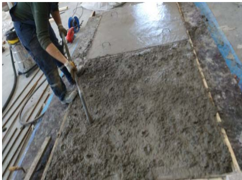
(e) Compaction by handheld electric vibrator
