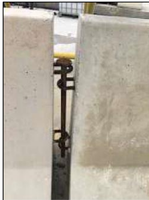
Figure 4.25. Concrete barriers connected pins for pendulum test
