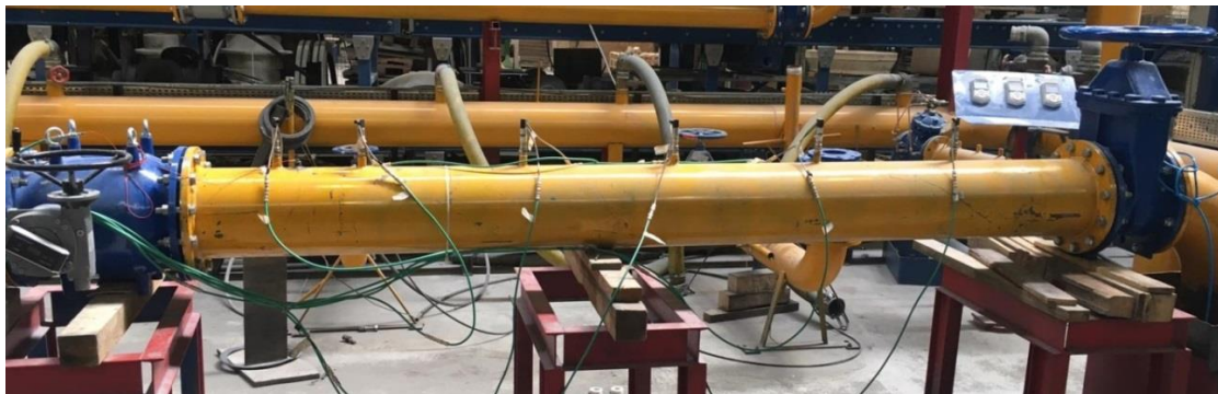
Figure 3.6 Sensors on the Downstream Pipeline
