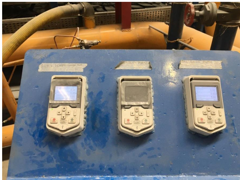
Figure B.2 Pump Control Devices
