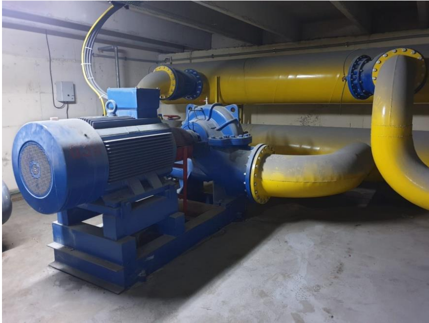
Figure B.3 Centrifugal Pump
