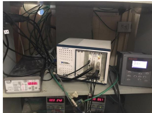
Figure B.5 Accelerometer Preamplifier / NI PXIe – 1071 chassis / Power Supplies
