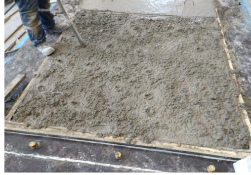
b) Compaction by handheld electric vibrator
