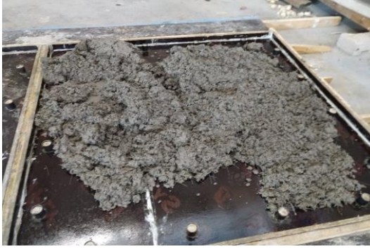
a) Pouring half mixture into formwork
