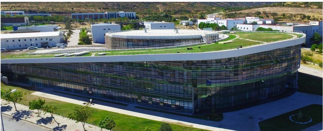
Figure 3.2. IZTECH Innovation Center.
