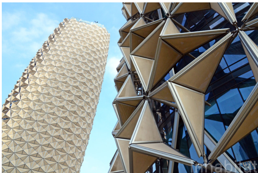
Figure 2.3. Spherical mechanism usage as sun shading component. (Source: Url2)
