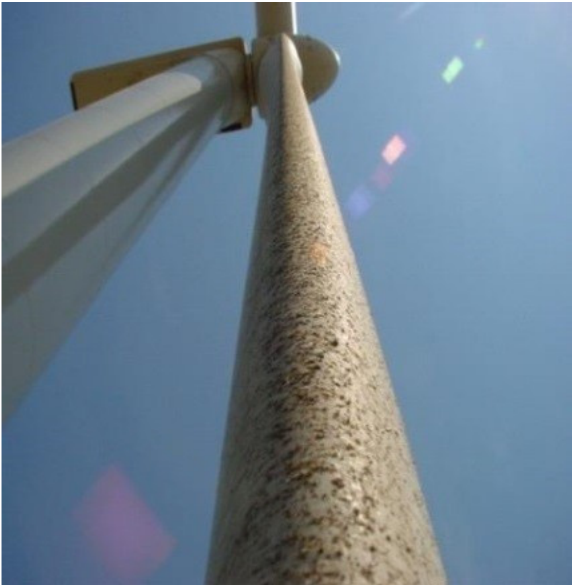
Figure 4.5: Insect Accumulation on Wind Turbine Blade (Source:[Wilkinson, 2014])
