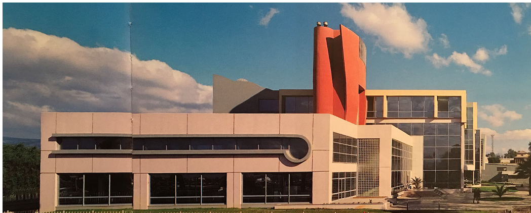
Figure 4.58. Çimentaş Social Service Building. (Source: photo by Cemal Emden, source: Mimarlık Yıllığı 1, 2000, p.138)
