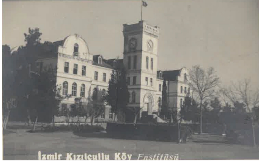
Figure 2.8. The Clock Tower in Kızılçullu, 1951. (Source: Erbil Coşkuner Archive)
