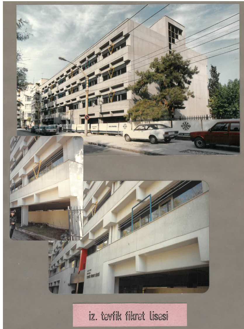
Figure 4.28. İzmir Tevfik Fikret High School during construction, before the top floor was added, collage by Pro-Dek (Source: Erbil Coşkuner Archive).
