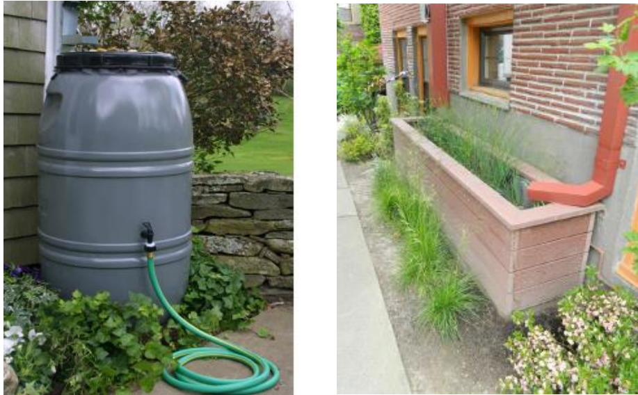
Figure 3.9. Rain Barrel and Stormwater Planter (Source: Vysoky, 2017)
