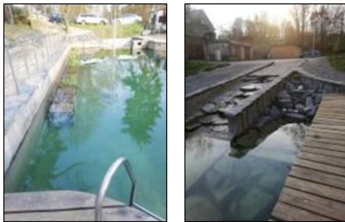
Figure 4.65. An Ecological Pool Which is using Stormwater and Surface Water for Water Supply and Plants for Purifying the Water. (Source: taken by the author in Prague)
