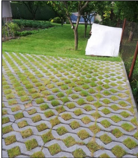
Figure 3.8. Concrete Block Pavers for Purpose of Parking Place in a Garden in Prague, Czech Republic (Source: taken by the author on 24/03/2020)
