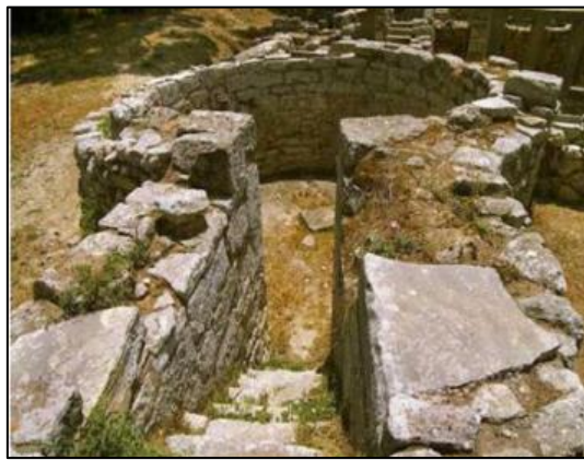
Figure 2.2. Minoan Cistern at the Ancient Town of Tylissos, Crete (Source: Angelakis & Spyridakis, 2010)
