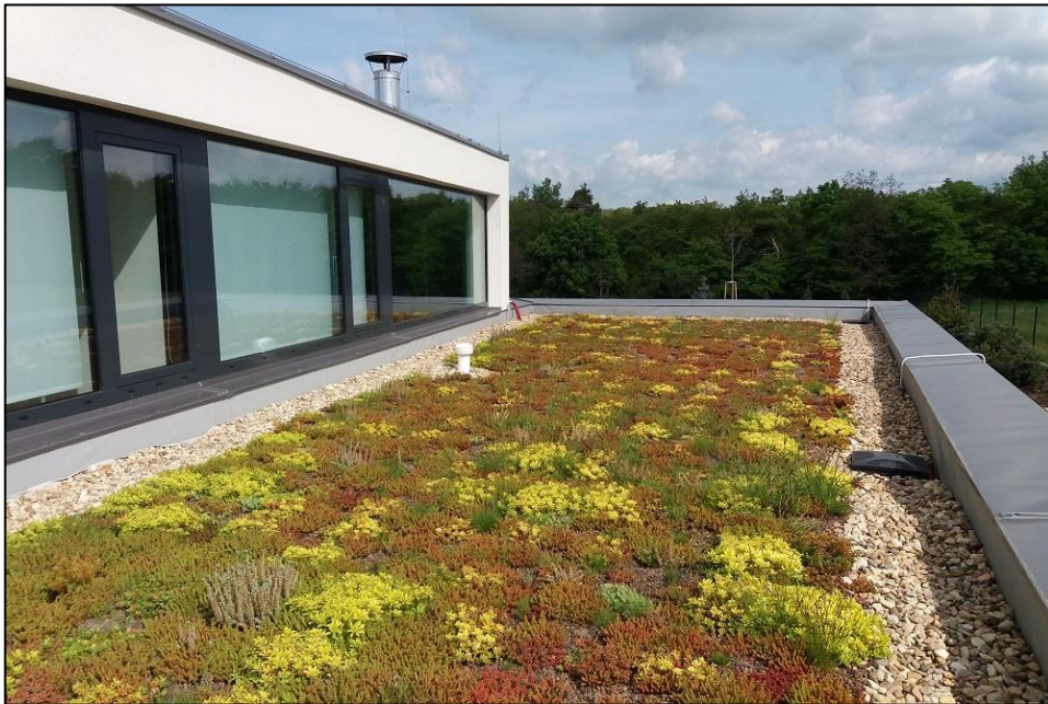
Figure 3.6. Green Roof of a House in the Czech Republic (Source: Url 9)
