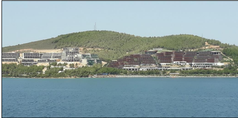
Figure 4.22. A 5-Star Hotel Construction after Deforestation (Source: Url 17)
