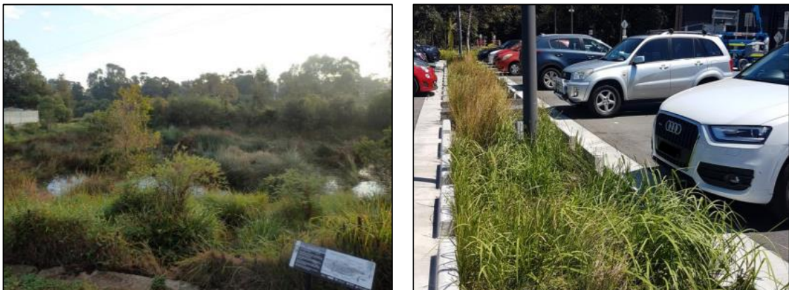
Figure 3.13. On the left, bioswales near carparks to collect stormwater. On the right side, constructed wetlands treats stormwater runoff from local streets before it enters to the creek (Source: Sydney WATER, 2018)
