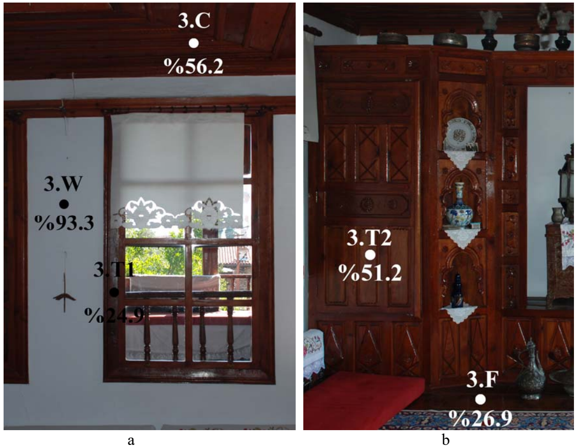
Figure 5.58. The surface reflectance at the measurement points in the main room of Kestaneciler House on the south wall (Prepared by Author, 15.10.2018) (a), on the west wall (Prepared by Author, 15.10.2018) (b)
