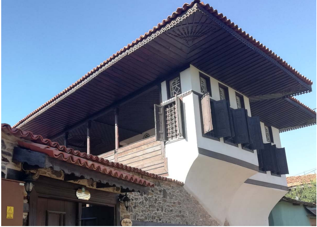
Figure 4.11. Under the eave flat and inward sloping wood veneer in Beyler House, Kula, Manisa (Prepared by Author, 02.10.2019)
