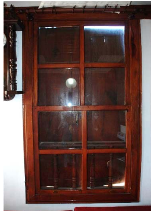
Figure 2.13. The perpendicular sliding sash ( giyotin ) in main room, Kestaneciler House, Kula, Manisa (Prepared by Author, 15.10.2018)
