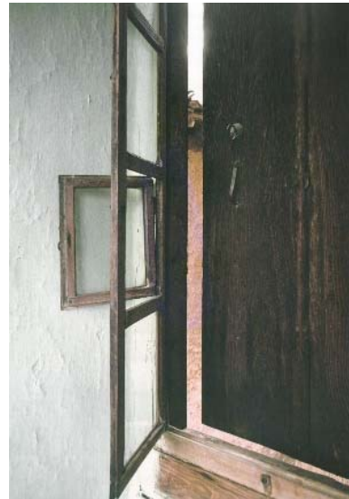
Figure 2.15. The combination sash ( karma kanat ) which has a second small sash in the vertically hinged casement (Source: Küçükerman, 1978/2007,123-126)
