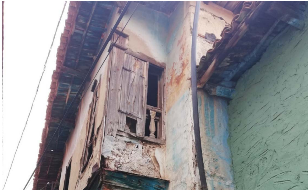
Figure 4.10. Under the eaves uncoated and exposed beams in Urlar House, Kula, Manisa (Prepared by Author, 26.07.2018)
