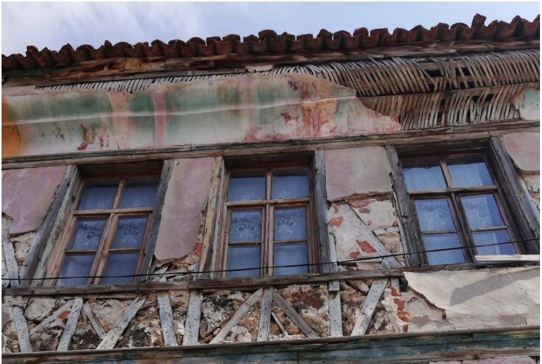
Figure 4.12. The wood-lath concave eave in Kula, Manisa. (Prepared by Author, 25.07.2018)
